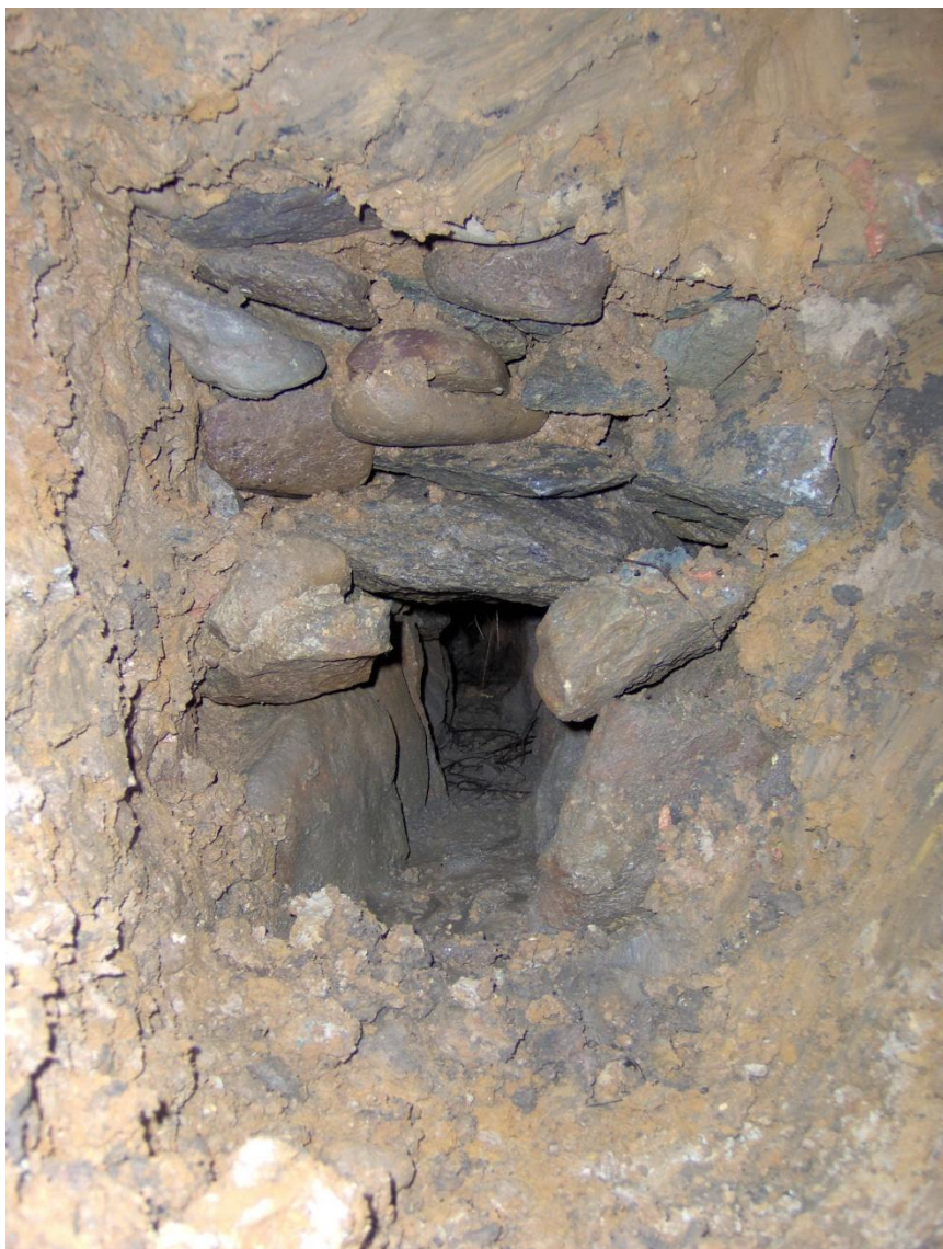
Figure 5: View showing an exposed section across the stone culvert
