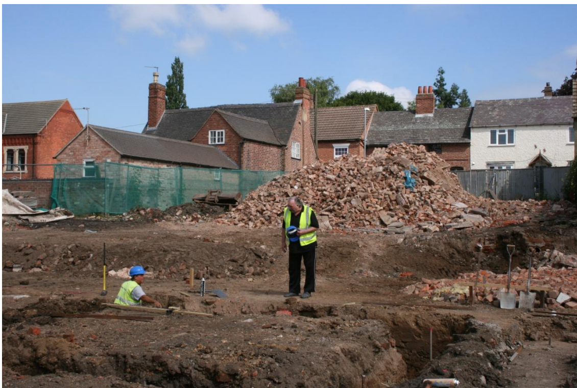
Figure 3: View looking north across the development area towards Dennis Street
