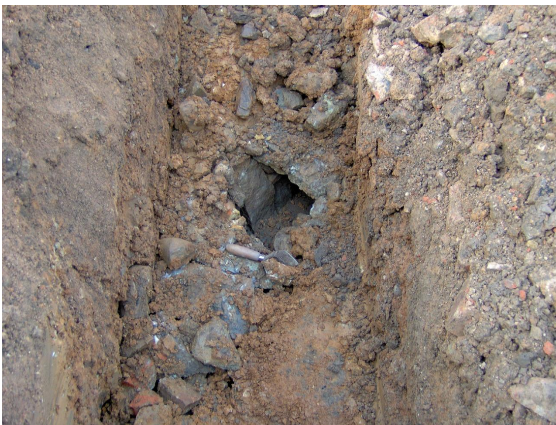
Figure 4: View showing the exposed stone culvert beneath Plot 1. Looking west
