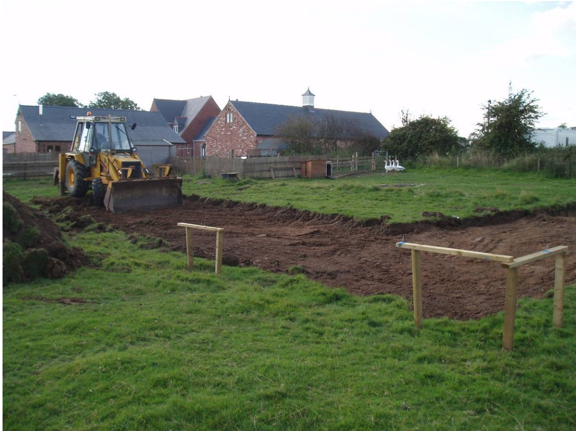
Figure 3 General Shot Looking South-West
