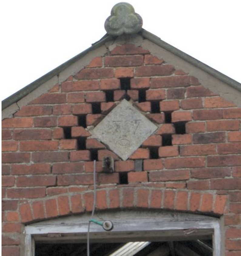
Figure 8 Date Stone on Left Hand Gable.
