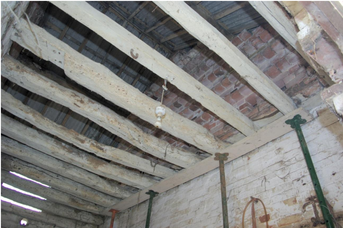
Figure 12 Limited View of Roosting Ledges on Right Hand Gable.
