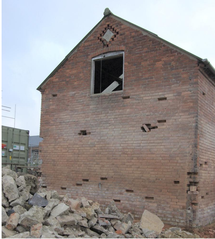
Figure 5 Left Hand Gable (From the Southwest)
