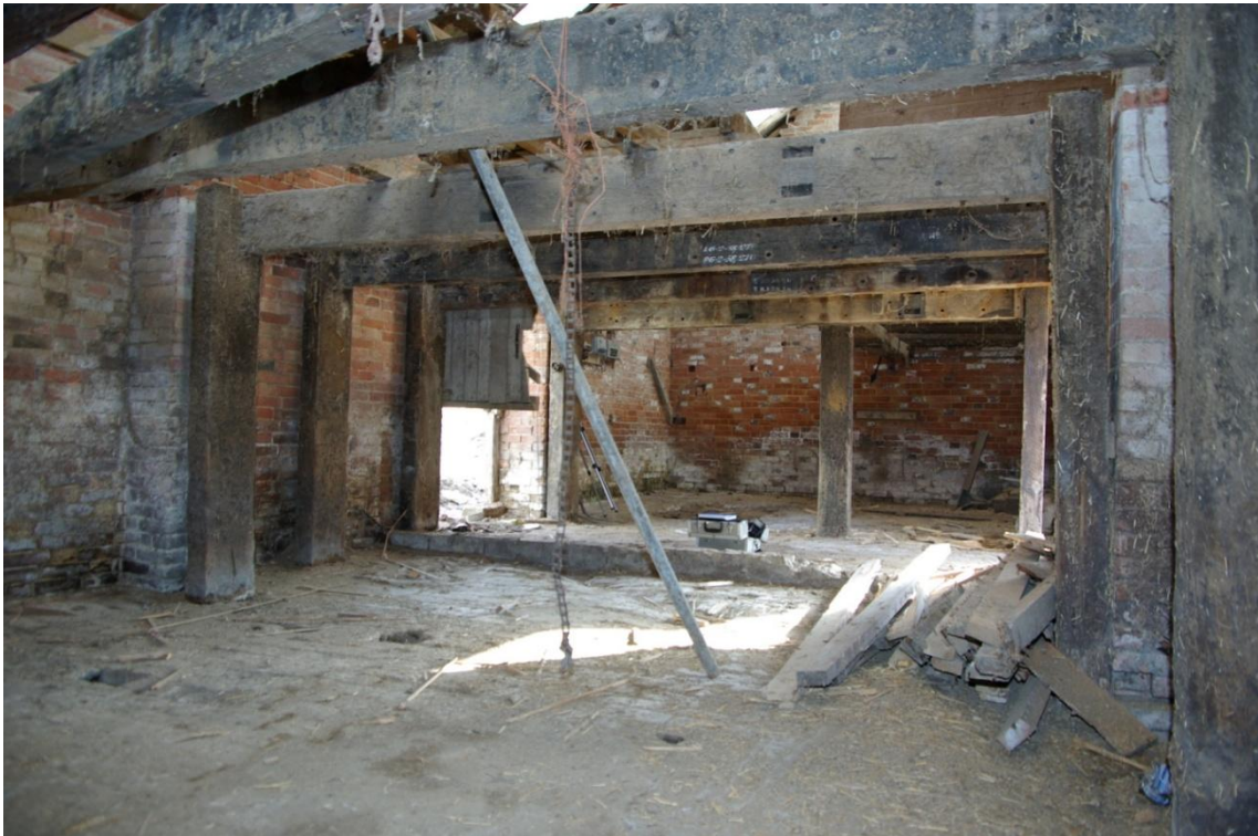
Figure 10 Inserted Floor of Reused Railway Sleepers.
