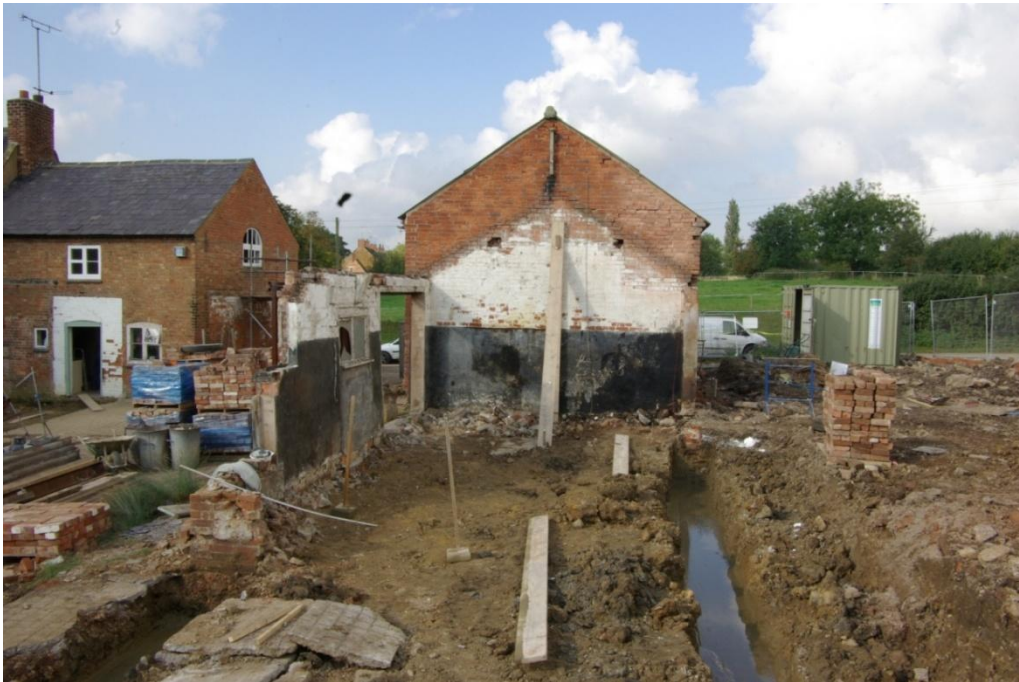
Figure 6 Right Hand Gable (From the East)
