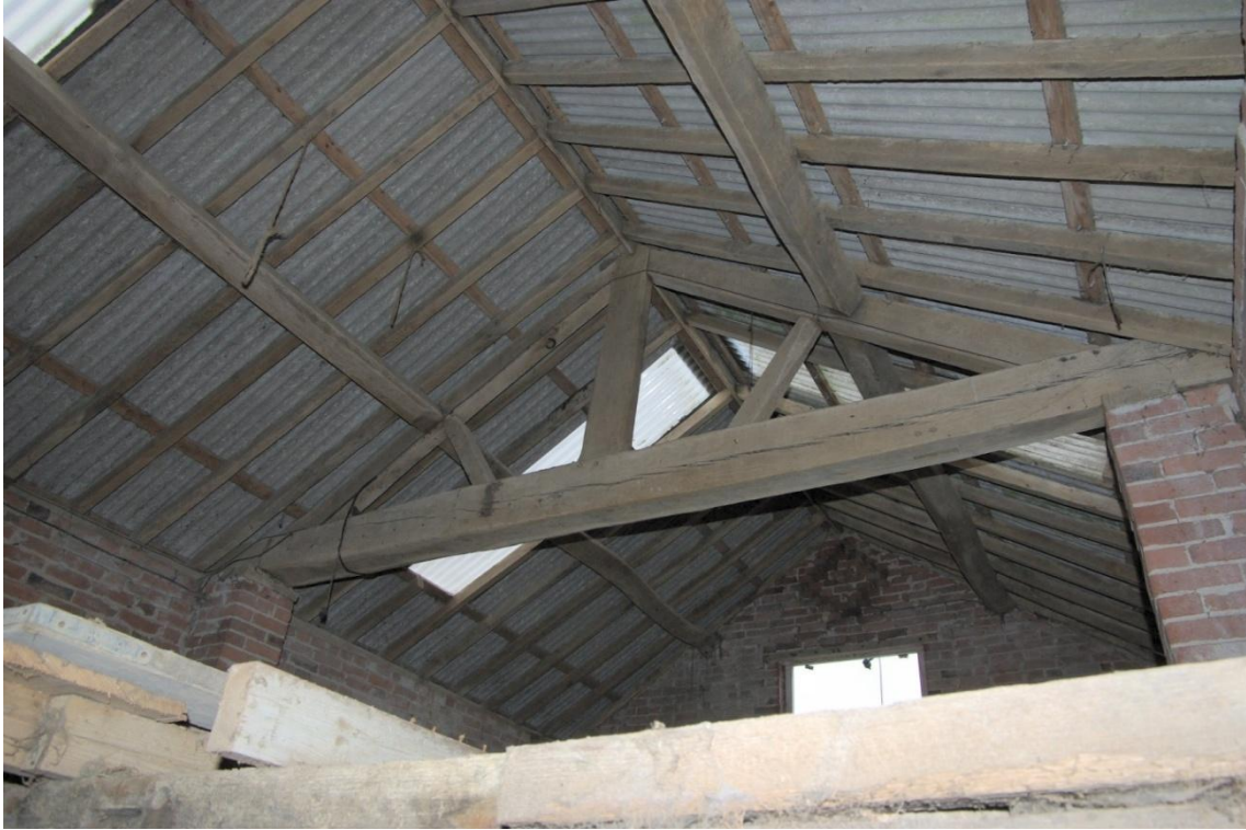
Figure 9 Roof Truss.
