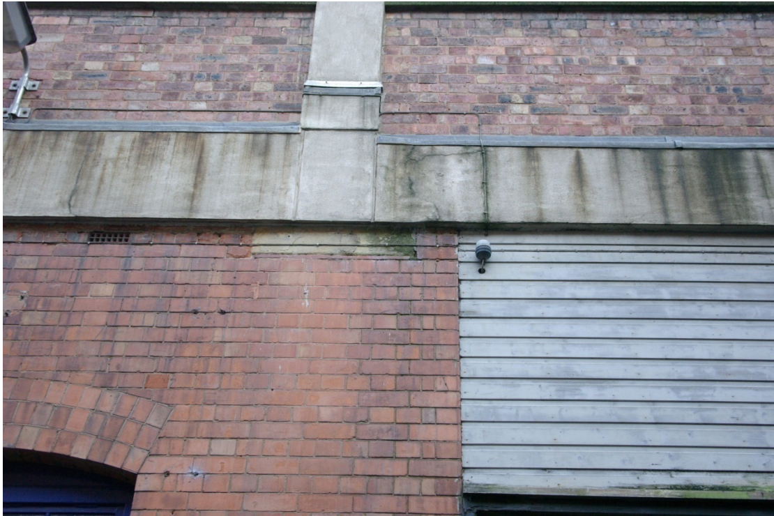
Figure 7 Change in Concrete Frame Near Retained Bays.
