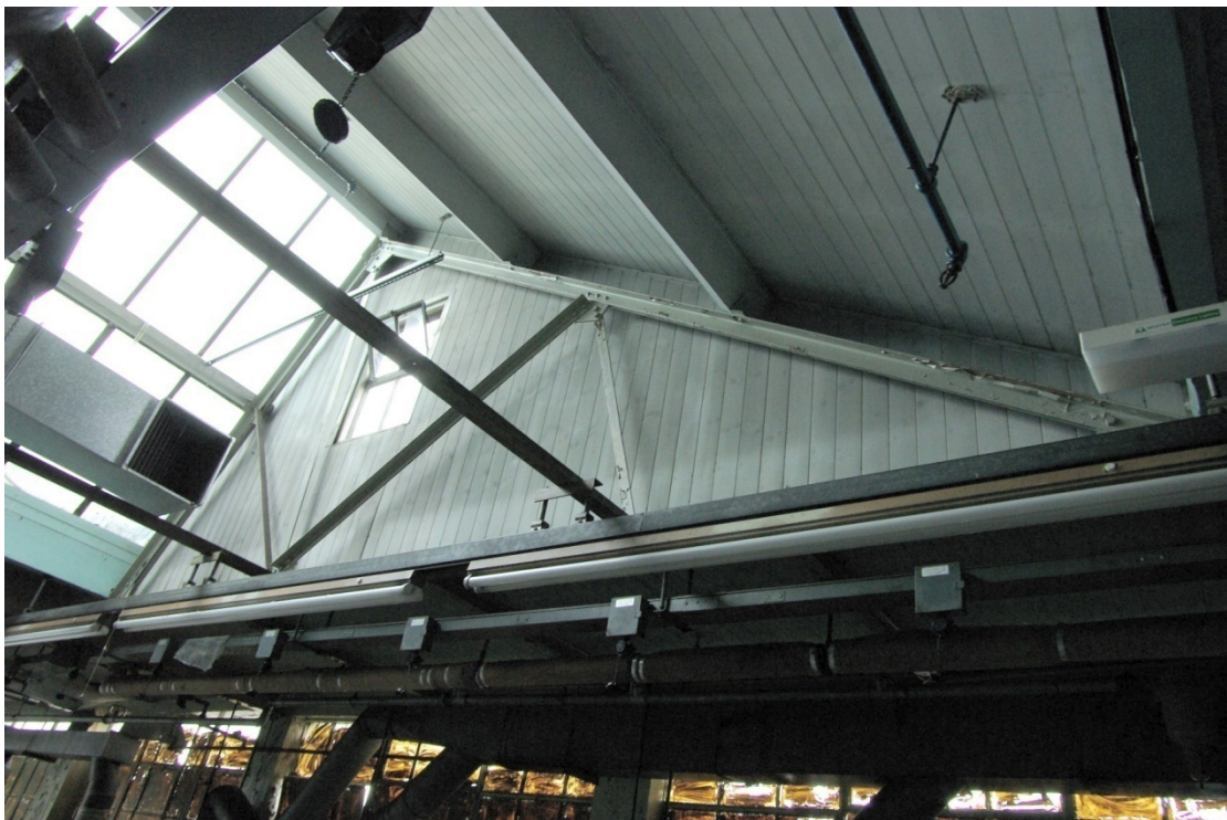
Figure 10 Detail of Roof Construction.
