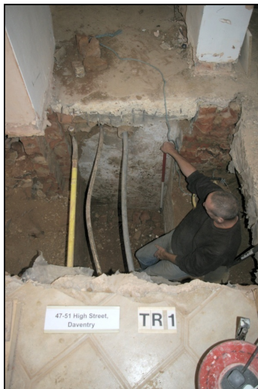
Figure 4 Trench 1 (Looking South-south-east).
