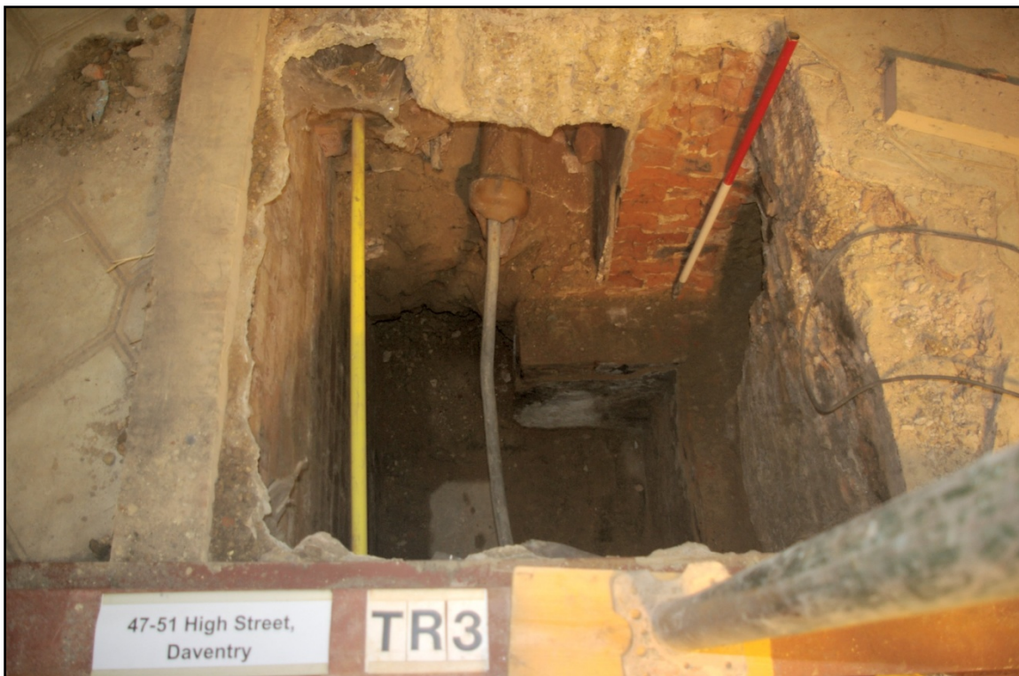
Figure 6 Trench 3 (Looking south-south-east).
