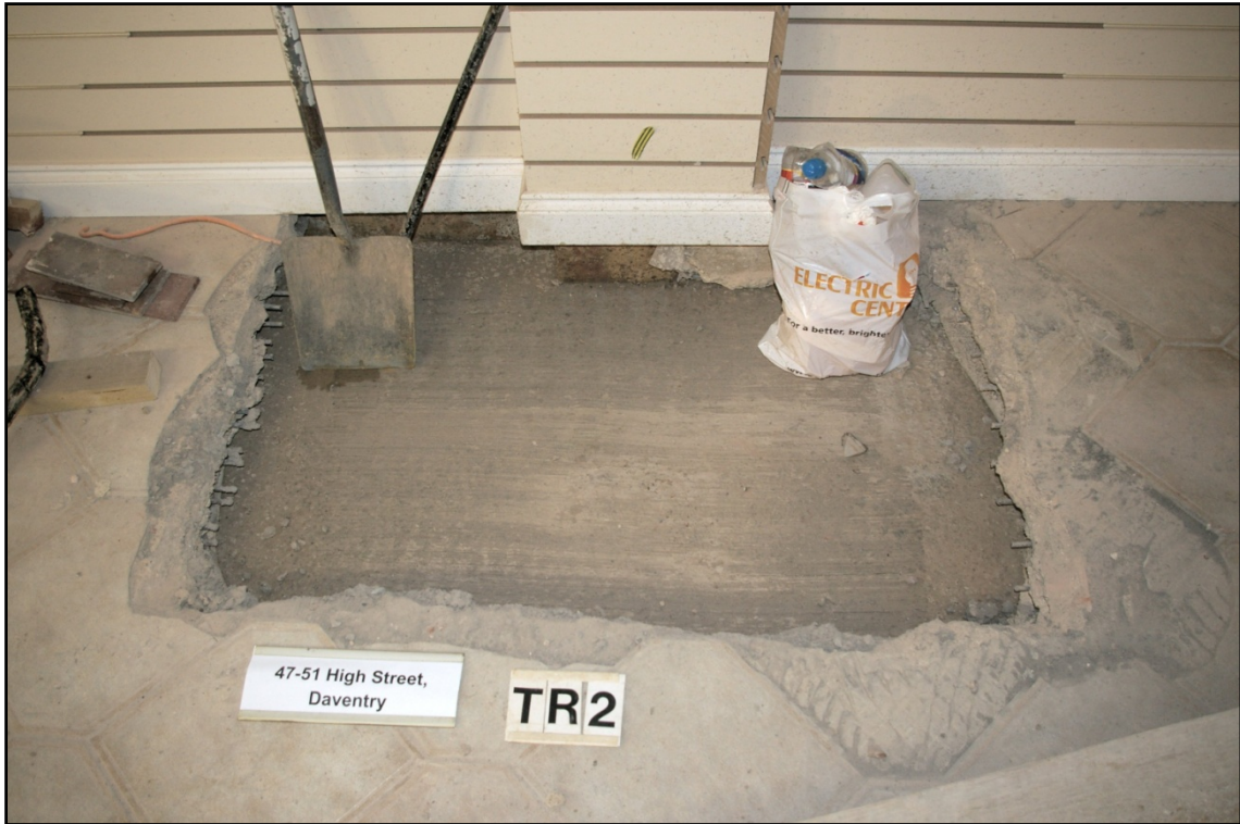
Figure 5 Trench 2 Showing Wall Stub (Looking west-north-west).
