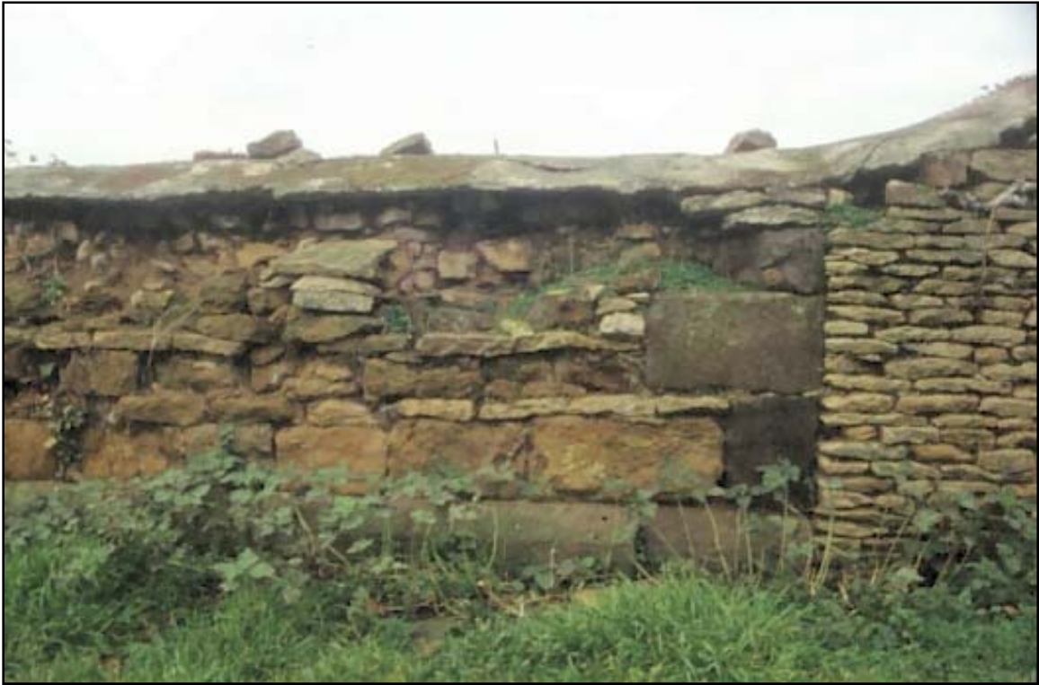
Figure 19 Building 3 Detail of quoin work and banding.
