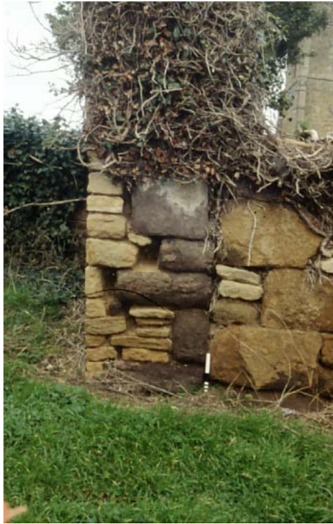
Figure 17 Building 2 Detail of quoin work.
