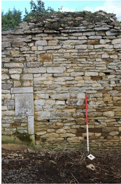
Figure 15 Building 1 Detail of easternmost quoin work.
