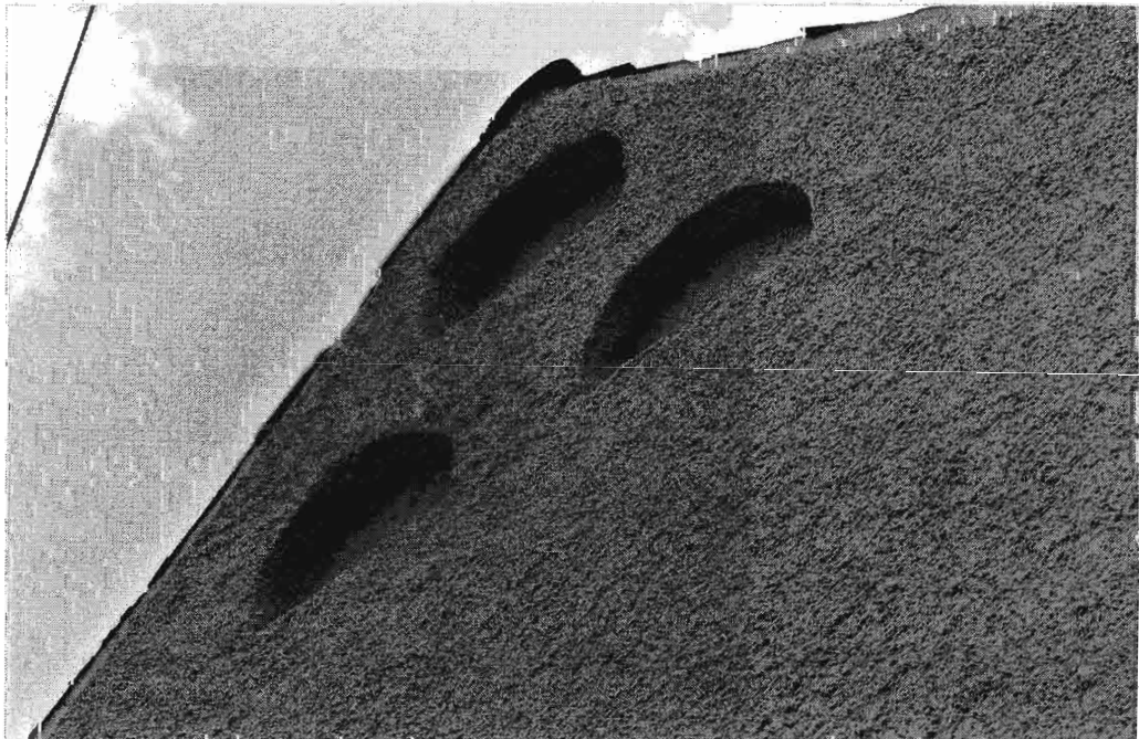
Plates 11, 12 Detail view of the 19 th century north gable of Bath Hotel showing the three recesses which may originally have been bee-boles.
