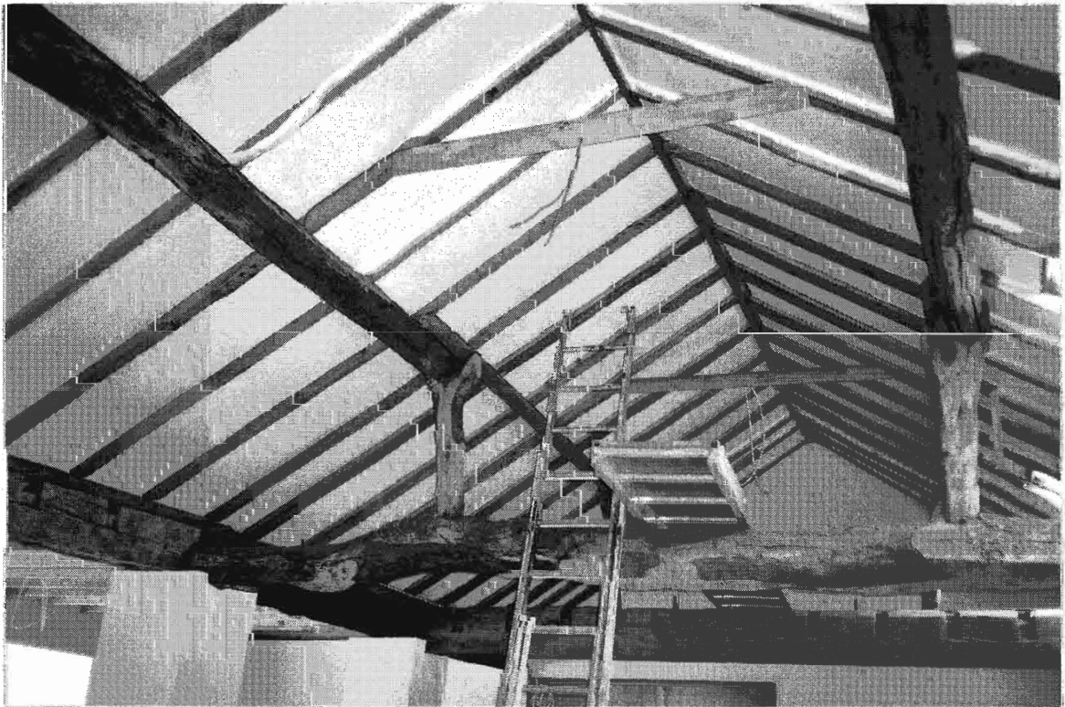
Colour Plates c13, c14 Detail showing re-used timbers in extension roof
