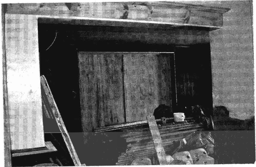
Plates 21, 22 General views of Ground Floor of 19 th century building, looking into original yard space subsequently filled by later buildings and now in process of refurbishment for restaurant use. All wooden shelves and beams shown in this series of Plates, i.e. 19 – 26, and 28 - 32 have been cleaned by sandblasting or a similar radical cleaning process.
