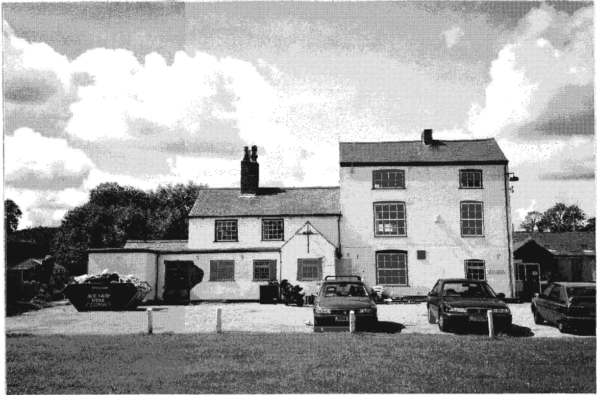
Colour Plate c1 Front elevation the Bath Hotel showing two storey 18 th century section and three storey early 19 th century section with 20 th century porch and other additions around the 18 th century build.
