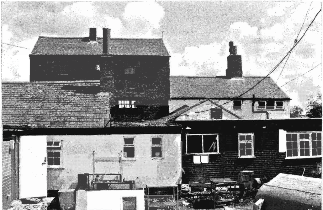
Plates 13, 14 Views of the west elevation of the Bath Hotel showing the extensive infill. The two pitched roofs belong to earlier buildings that were part of the original farmstead.
