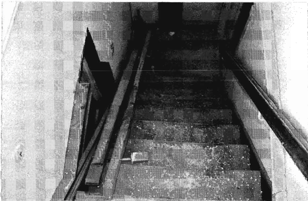
Plate 34 Staircase rising to first floor in 18 th century, two-storey Build.
