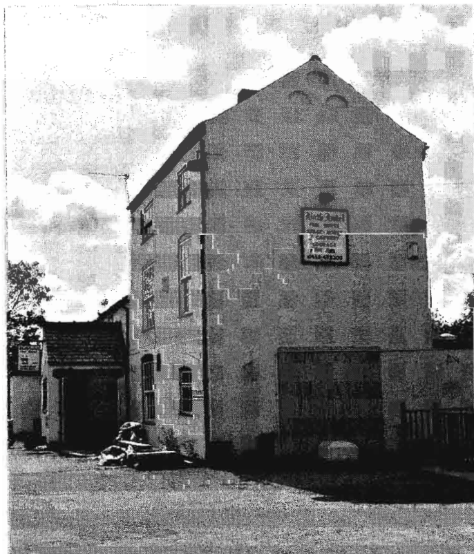
Plate 10 (below) Gable end of 19 th century, three storey build from north.
