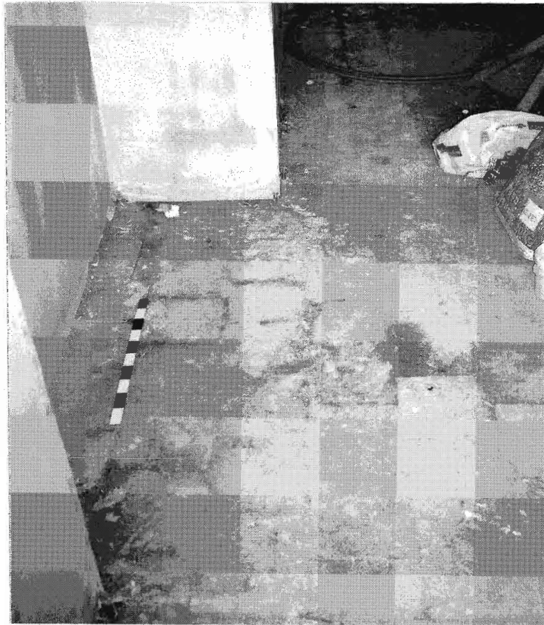
Colour Plate c9 Ground floor 19 th century quarry tiling in the 18 th century part of house.
