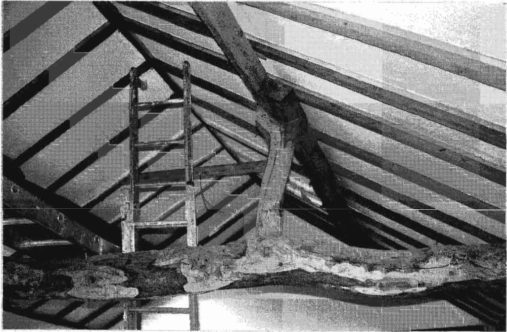
Plates 31, 32 Re-used oak structure introduced into roof of single storey extension on west side of building.
