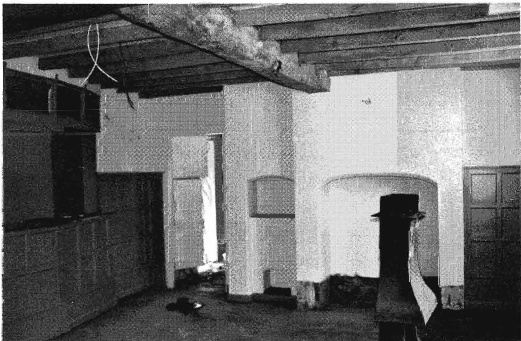
Plate 28 Re-used floor structure used as ceiling of single-storey building on west side of original farmhouse. All the panelling is 20 th century.
