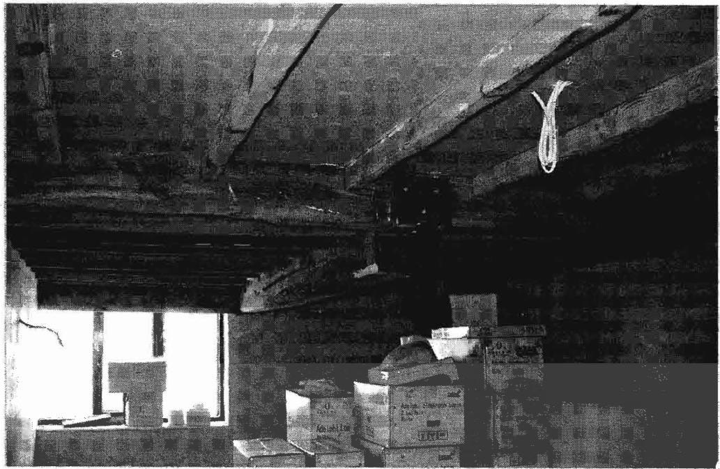
Plates 23, 24 View of Ground Floor ceiling of 19 th century building, with re-used material, (above). (Below) first floor structure of 19 th century build with re-used beam and joists visible.
