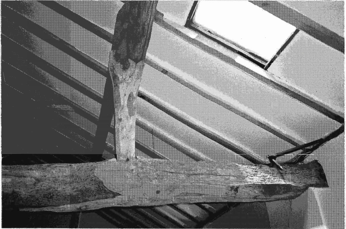
Colour Plates c13, c14 Detail showing re-used timbers in extension roof
