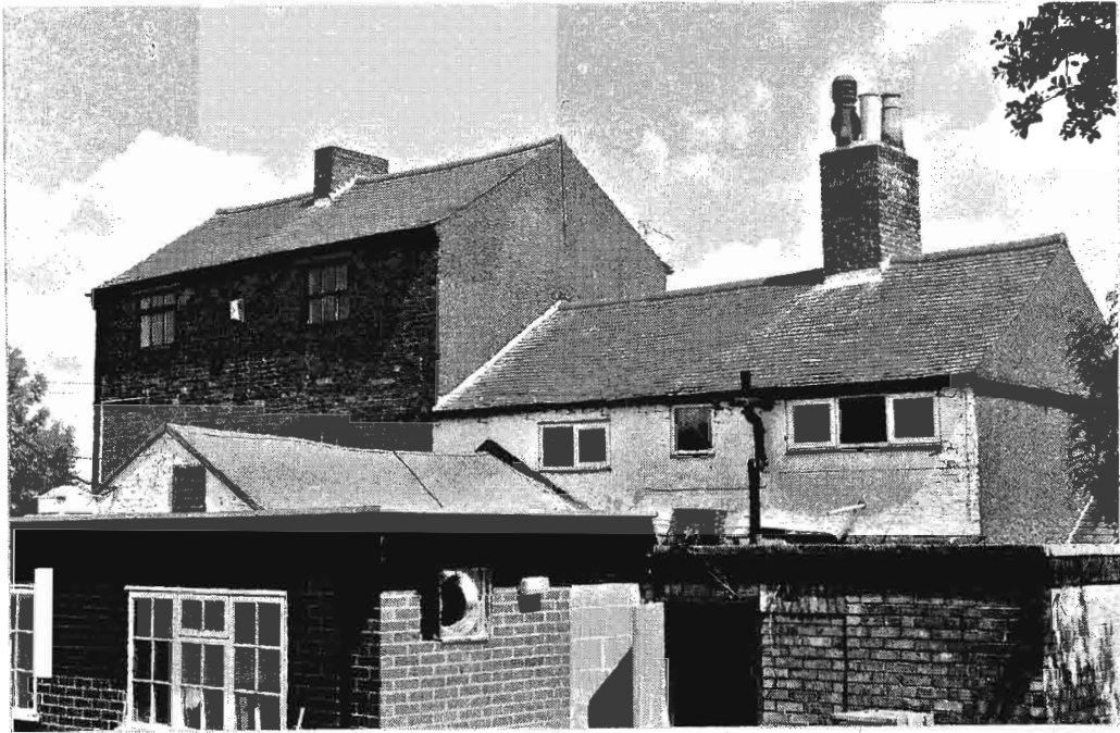
Plates 13, 14 Views of the west elevation of the Bath Hotel showing the extensive infill. The two pitched roofs belong to earlier buildings that were part of the original farmstead.
