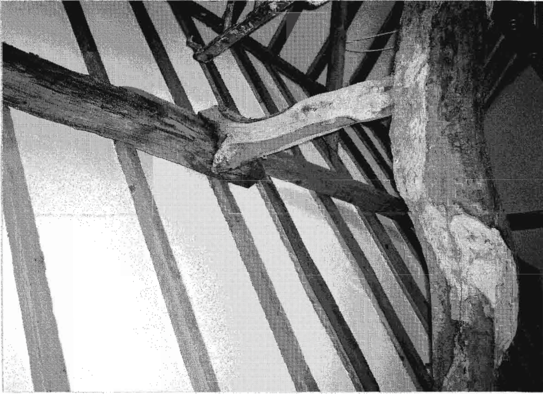
Colour Plate c15 Re-used timber detail in extension roof.
