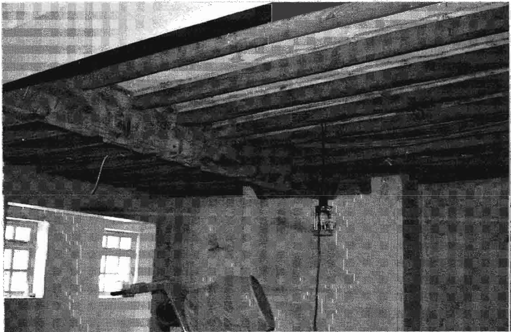
Plates 23, 24 View of Ground Floor ceiling of 19 th century building, with re-used material, (above). (Below) first floor structure of 19 th century build with re-used beam and joists visible.
