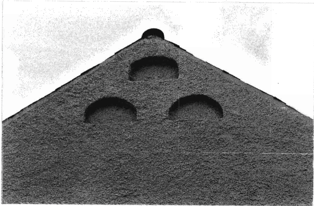
Plates 11, 12 Detail view of the 19 th century north gable of Bath Hotel showing the three recesses which may originally have been bee-boles.
