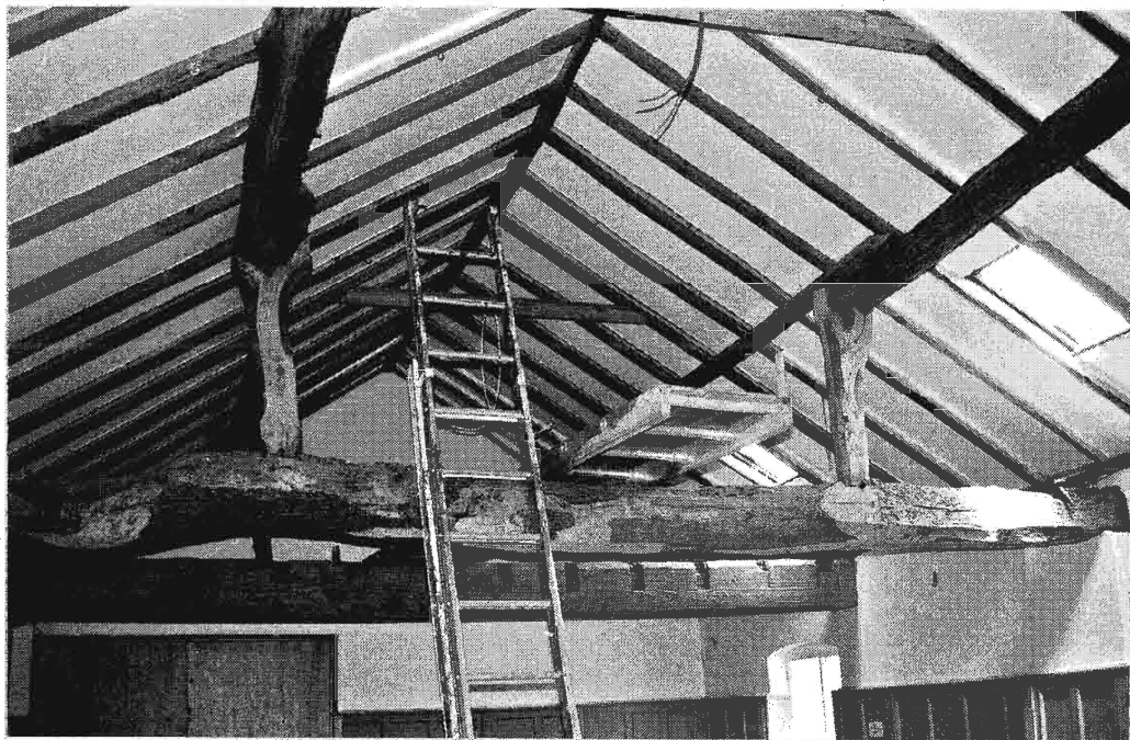
Plate 30 Re-used oak structure in roof of single-storey extension
