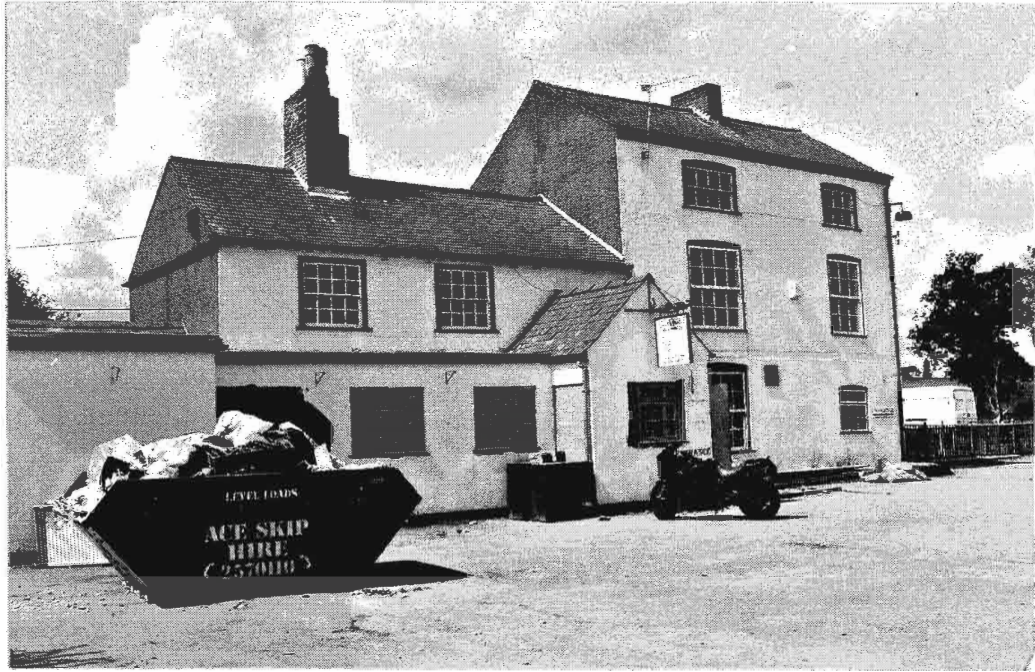
Plate 1 (above) Bath Hotel - view from the south-east. Principal elevation showing late 18 th and early 19 th century phases of building. The 18 th century section (left) is of two bays with the entrance passage, the later 19 th century three-storey, two bay section, was probably an addition to accommodate visitors to the spa. The entry porch and front passageway are late 20 th century additions.
