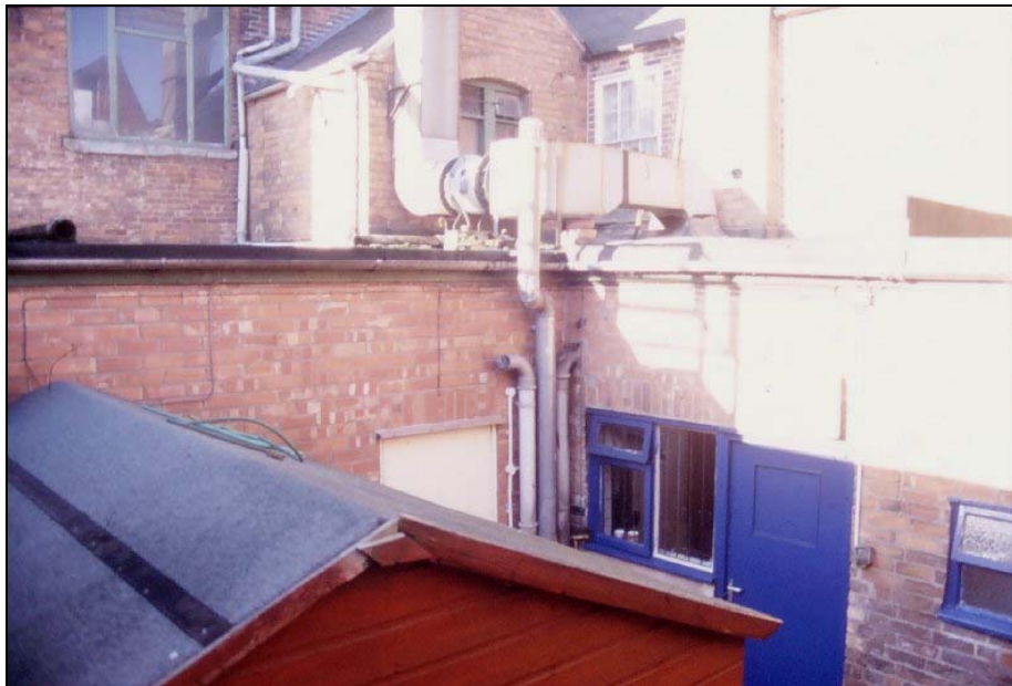
Figure 3. Rear of 59 Highcross Street showing (on right) single storey flat roofed range on north side of plot. In the lower right corner of the frame is the 19th century toilet block.
