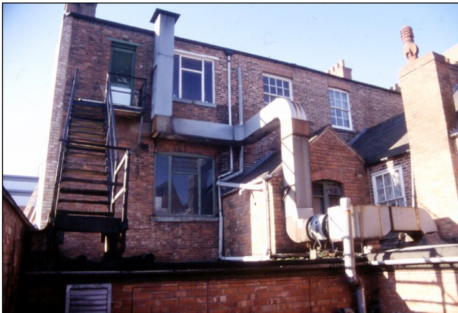
Figure 1. Rear of 59 Highcross Street showing the first floor section of the 19th century two-storey range (behind extractor ducting).
