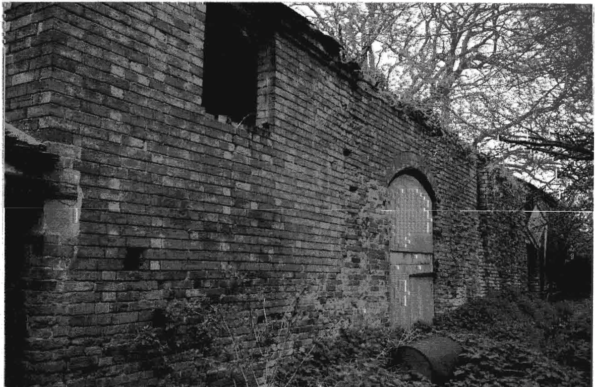
Plate 14 Rear, i.e., west elevation of Barn B with single, wagon entrance door and showing the severely weathered condition of much of the brickwork
