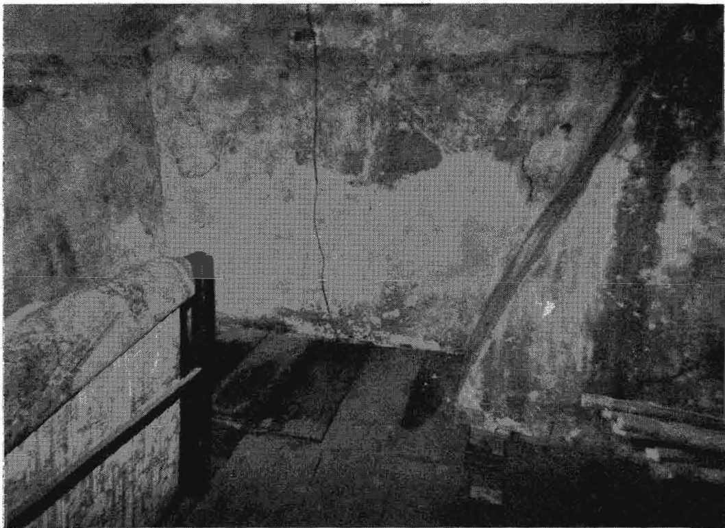
Plate 10 Detail of chimney hood at F 9 with stairs rising from G 7 to left and a section of the wide, hardwood, planked floor in foreground.
