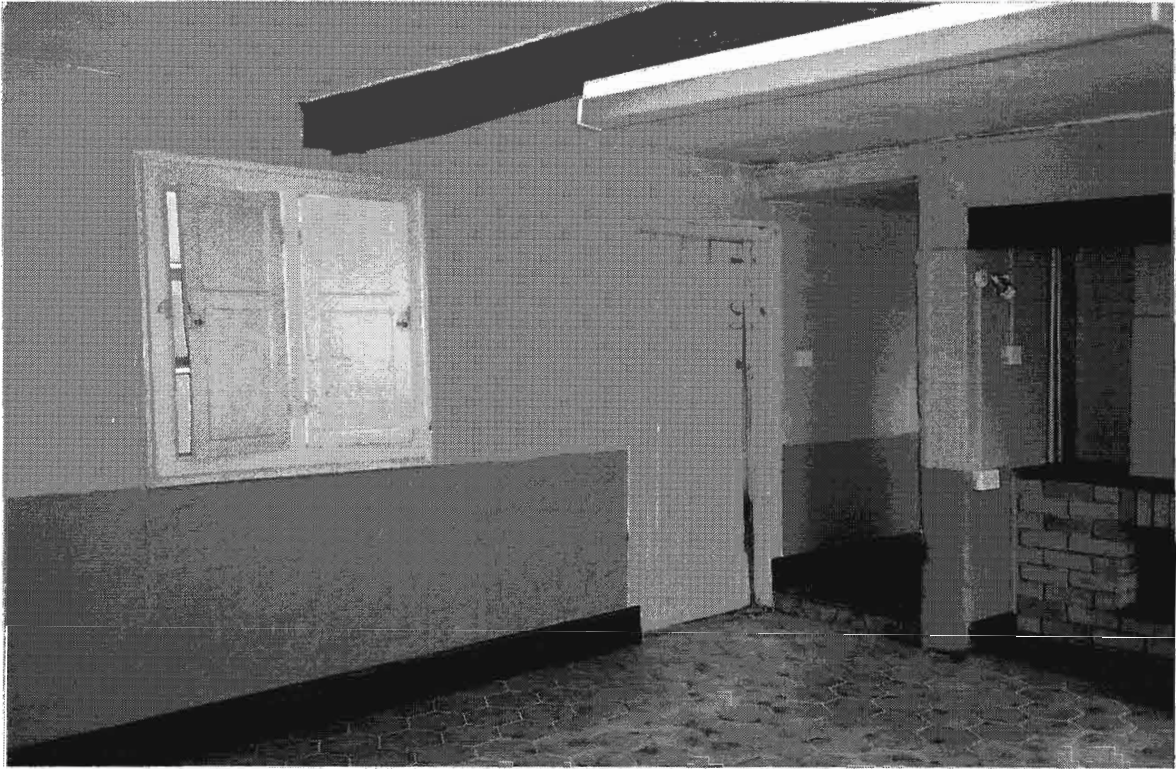
Plate 7 Interior detail of room G 4, looking towards fireplace and rear of building. Showing the plank and ledged door leading into G 6, Pantry, panelled doors of the wall cupboard, access to G 7 and part of chimney hood bressummer.
