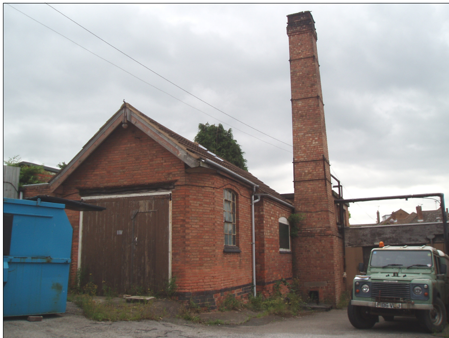
Plate 7: Engine House/Boiler Room
