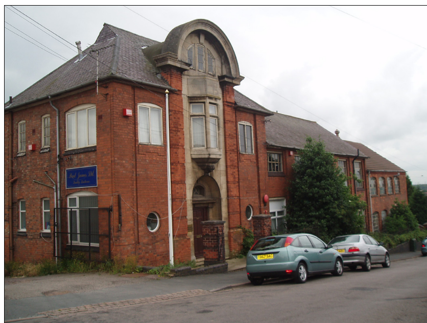
Plate 2: Principal factory building (looking south-east)
