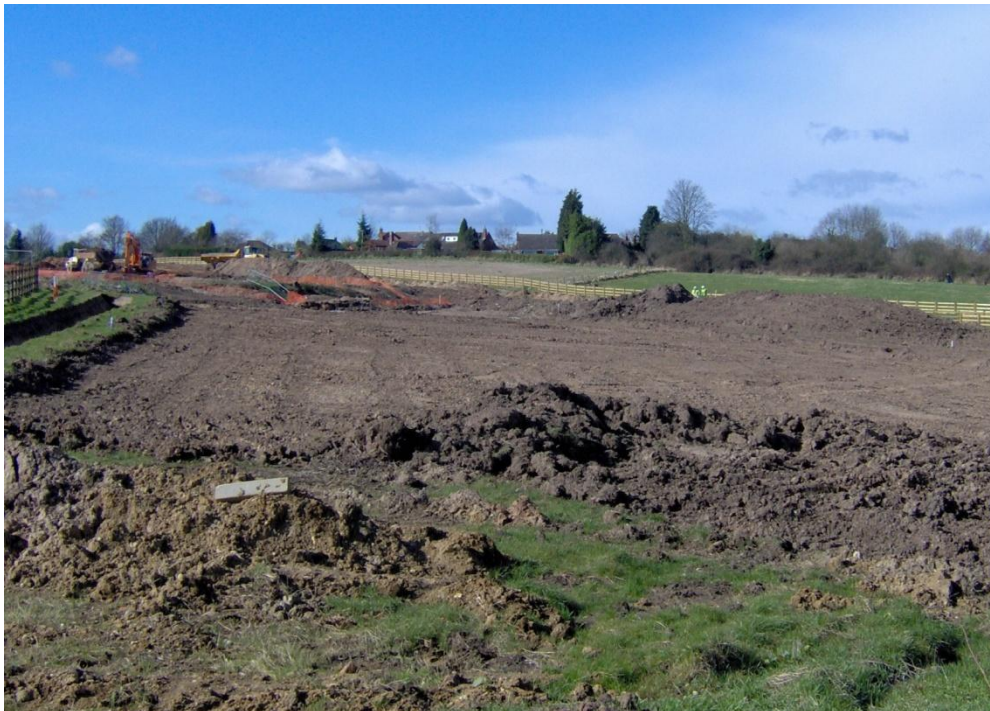
Plate 1 Site 4 looking south-west towards the fishponds. After initial topsoiling.
