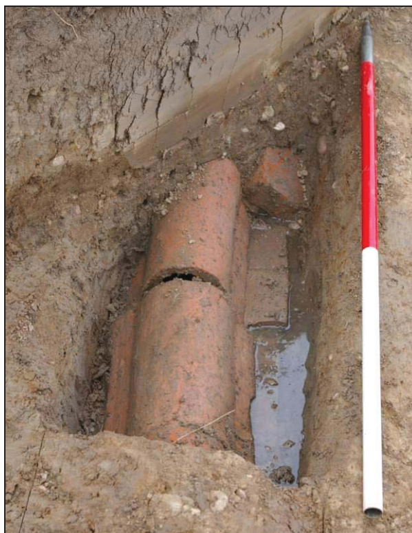
Plate 1, Land drain [11] seen north of ponds, running south to north. Note mixture of re-used material
