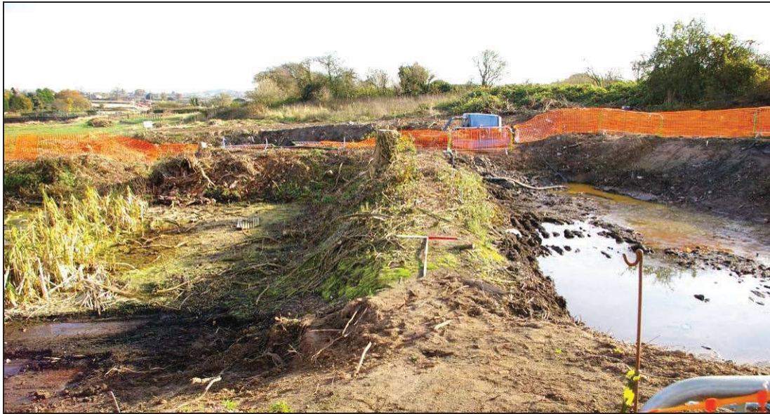
Plate 6, As plate 5, post-clearance and overburden removal. A gap can be seen in the bank at left between Pond 1 and Pond 2. Pond 3 on the right.
