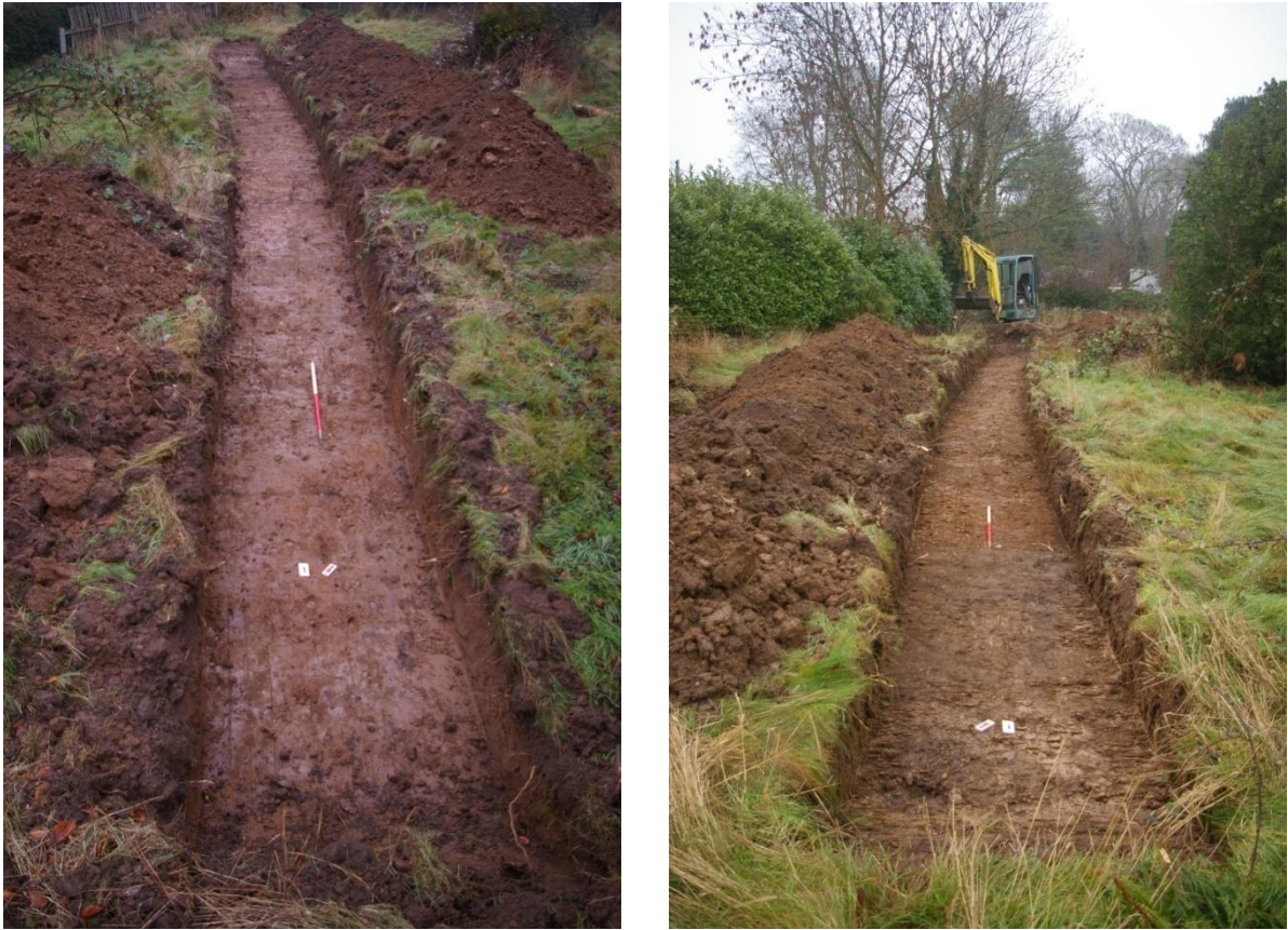
Figure 4: Trench 1 looking north-west (left) and south-east (right)
