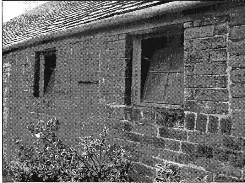
Plate 7. Partially blocked window openings, Barn 6. Looking southwest.
