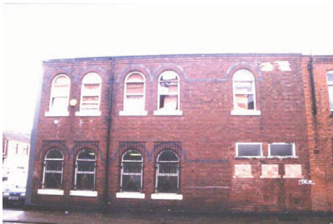
Figure 6. Fletcher Street Frontage (Building 3a).
