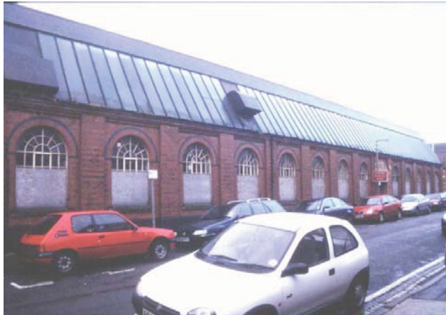
Figure 4. Oxford Street Frontage (Building 2).
