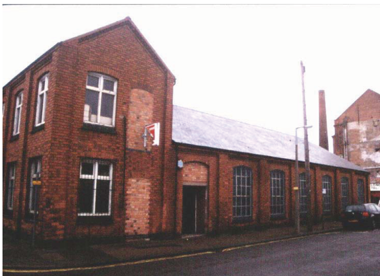
Figure 5. Regent Street Frontage (Building 2)
