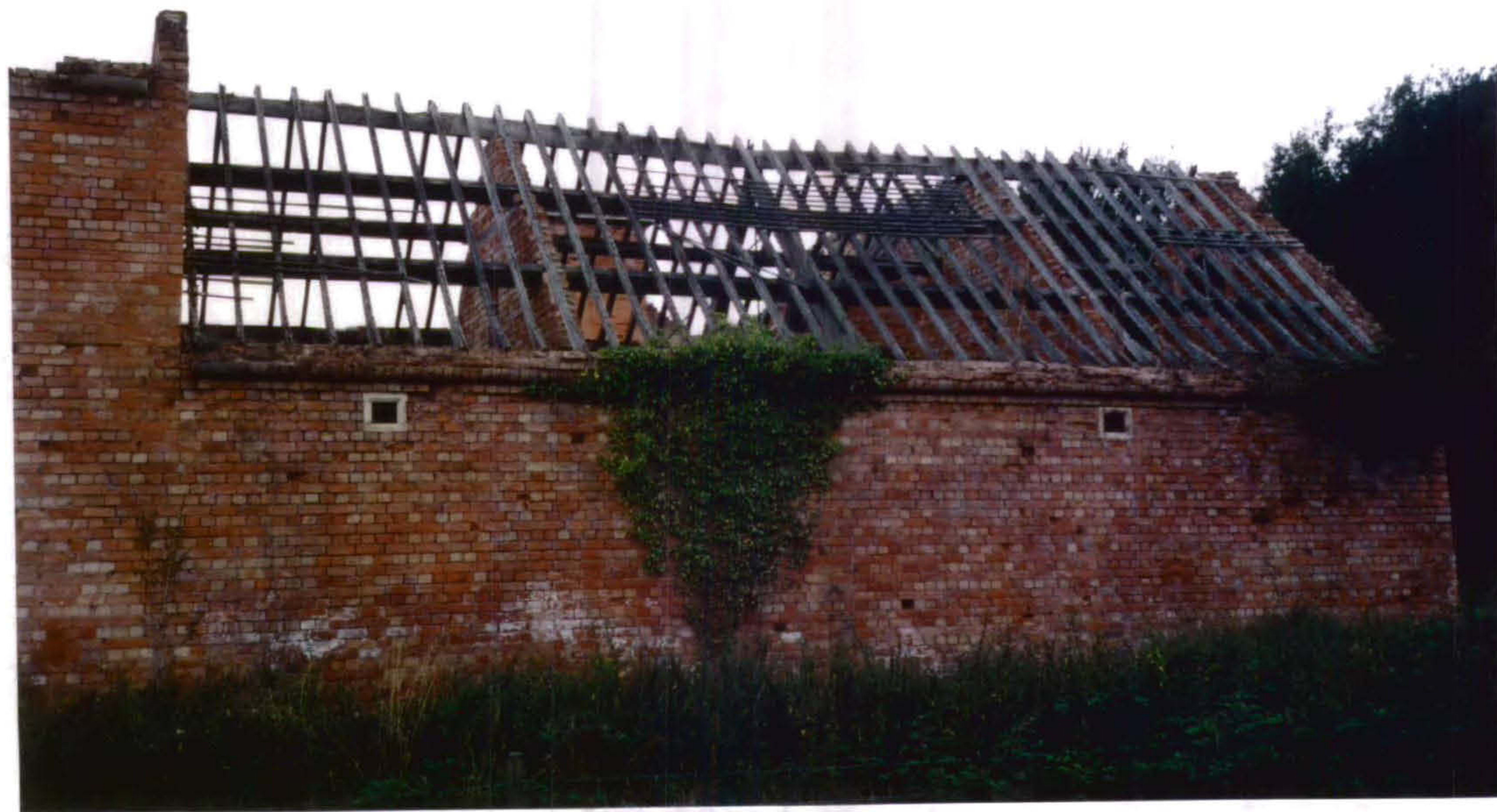
Plate 43 East Range – exterior, north-east corner. Showing original trusses and rafters still in place, 2003. Now removed.
