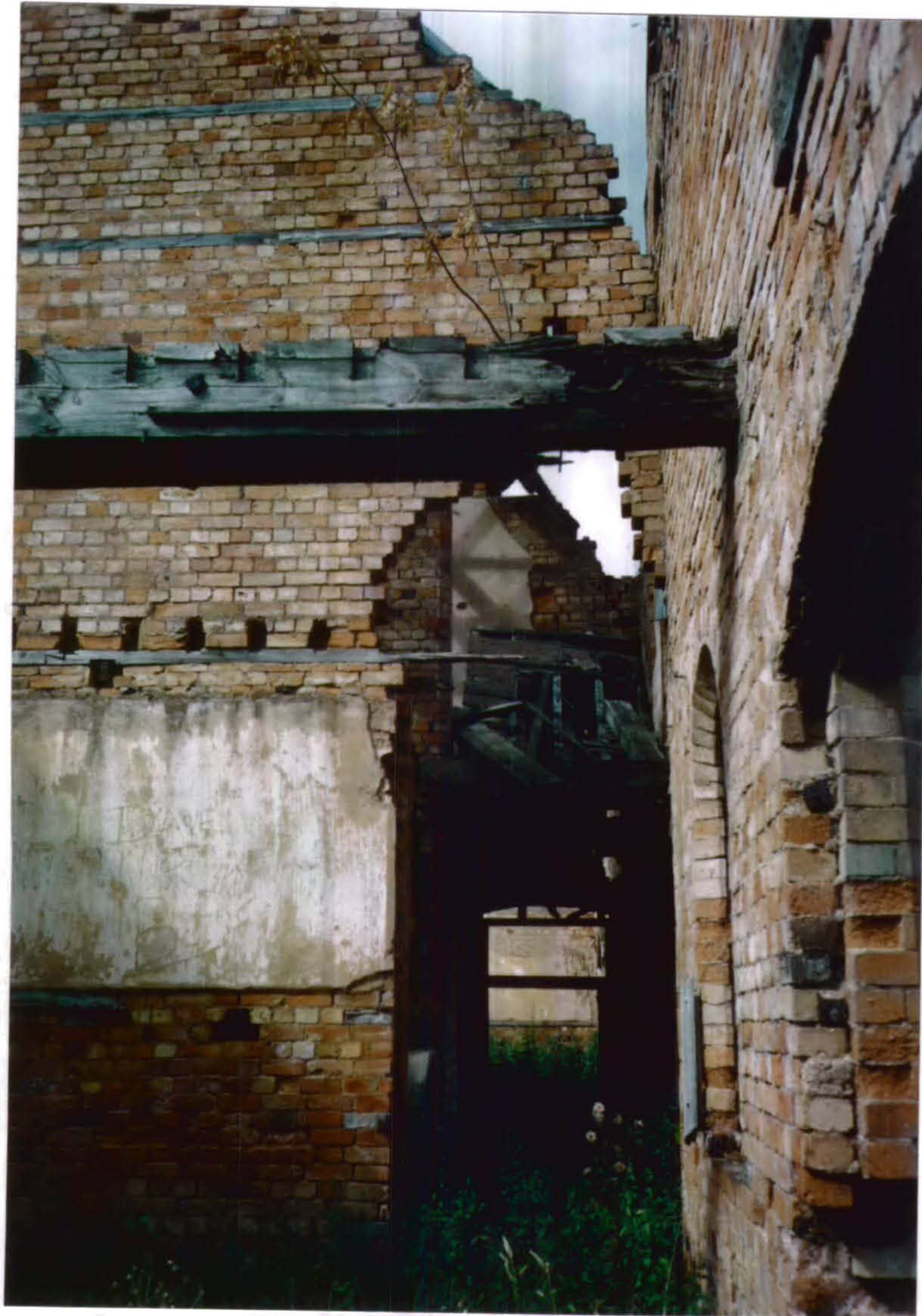
Plate 29 Interior detail in West Range, Stables. The transverse brick wall can be seen to have three sections of wooden bonding courses built into it.
