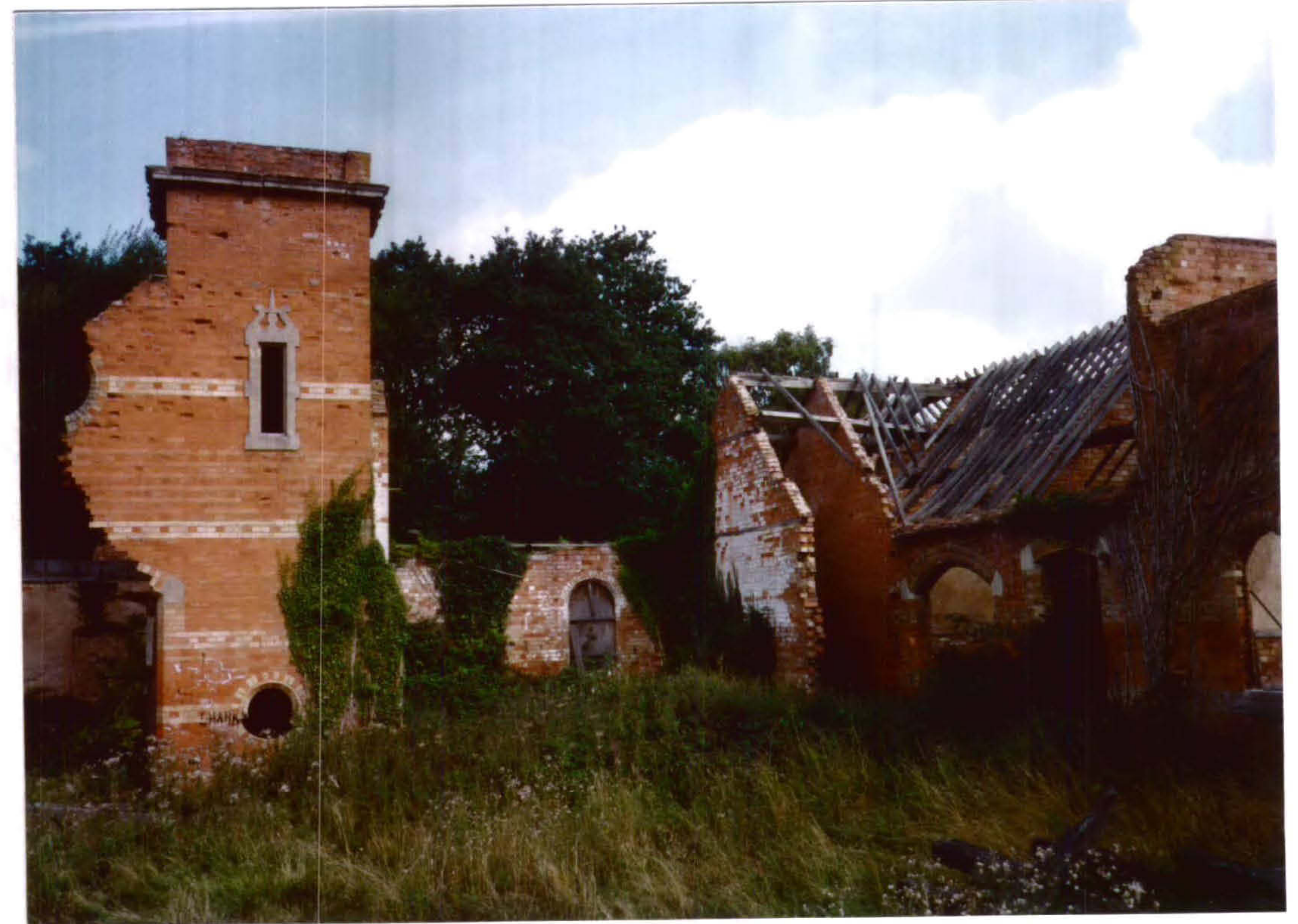
Plate 38 North Range, north-east corner. Showing void where the Blacksmith's workshop was. Also shows the walls of the passage leading out to the Gas House. The roof to the right is part of the East Range stabling.
