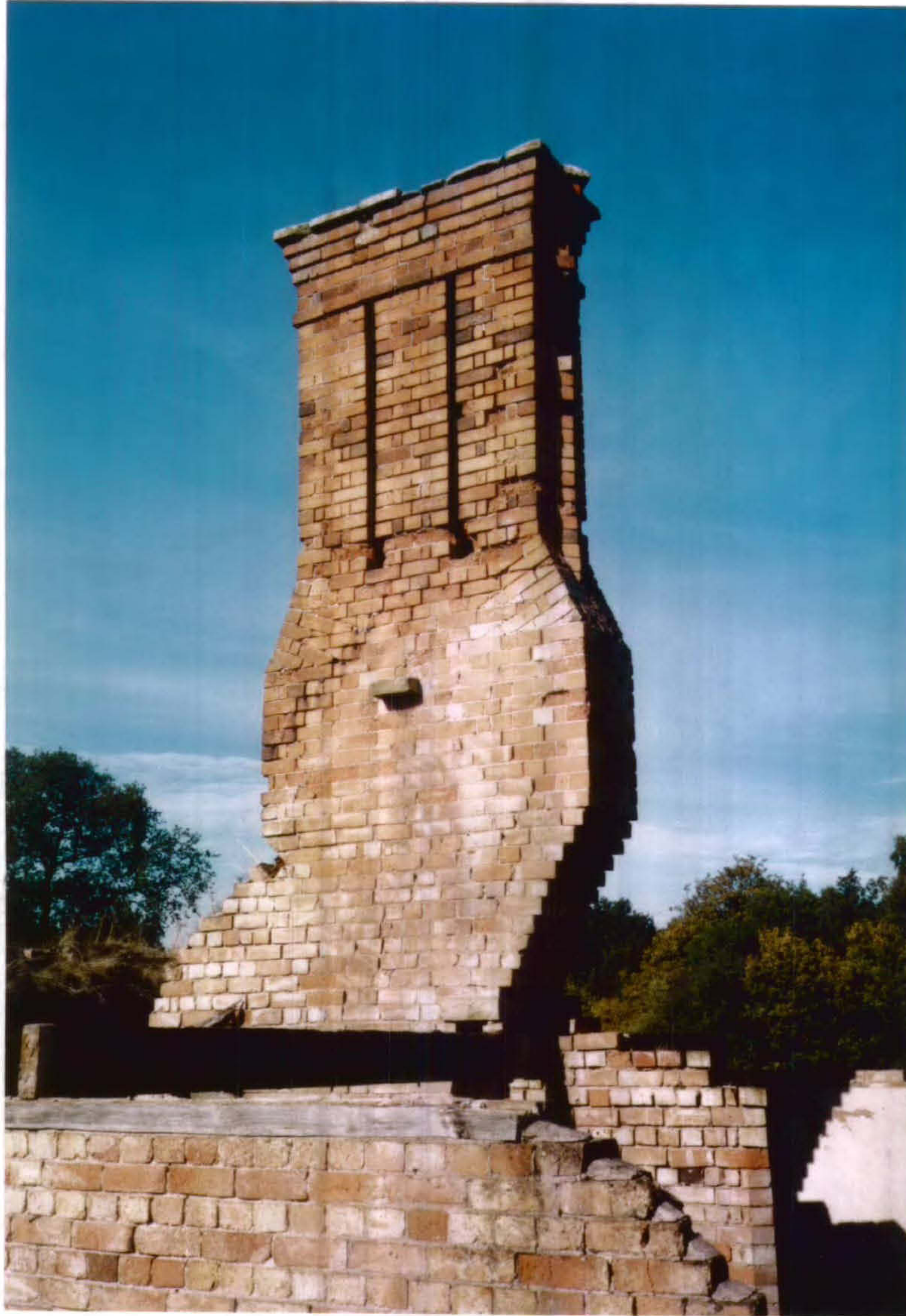
Plate 27 West Range : Brick Chimney originally servicing the Horse Grooms dormitory area.
