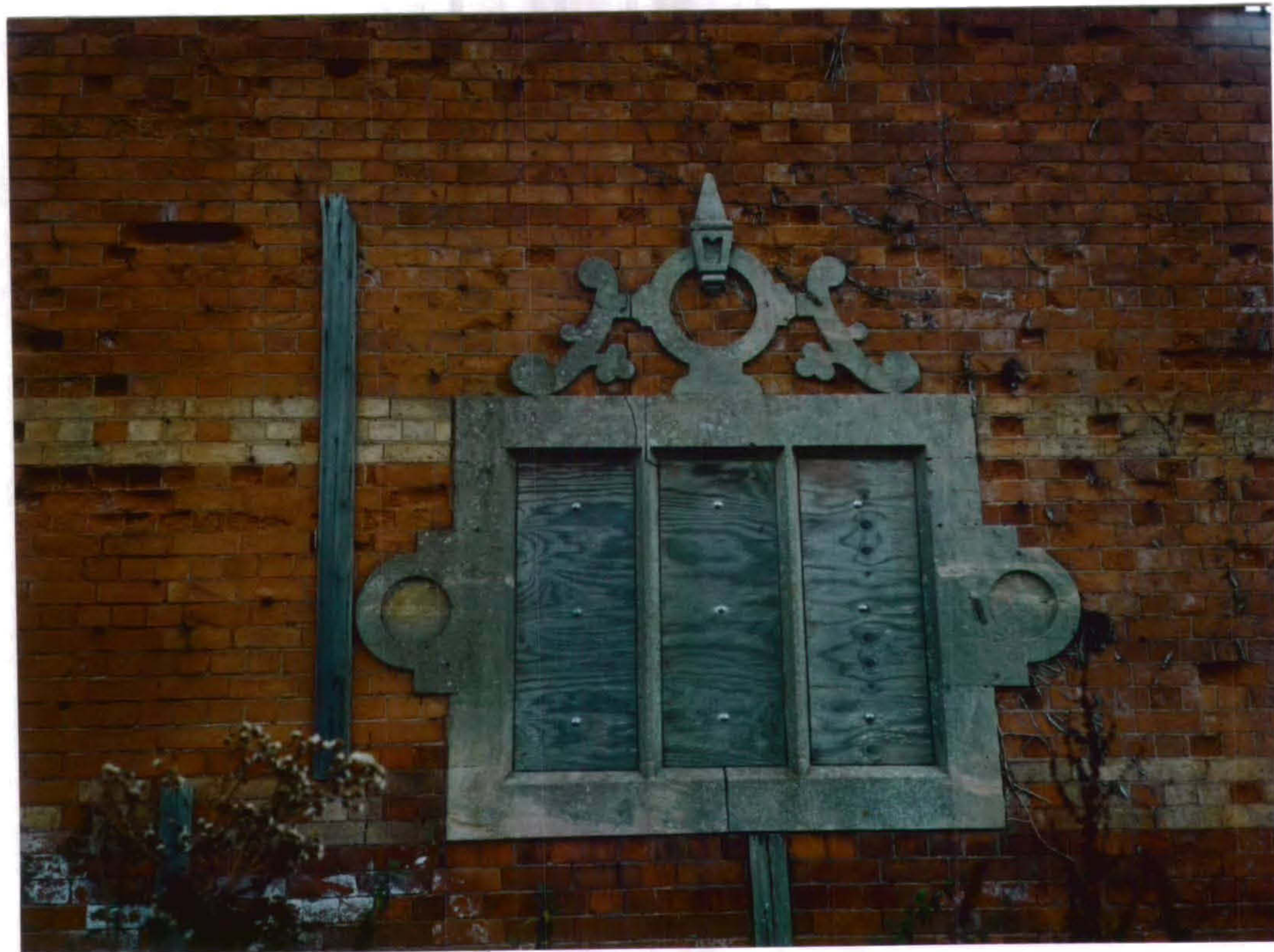
Plate 5 Detail of three-light, stone mullion window with strapwork head on the South Elevation.
