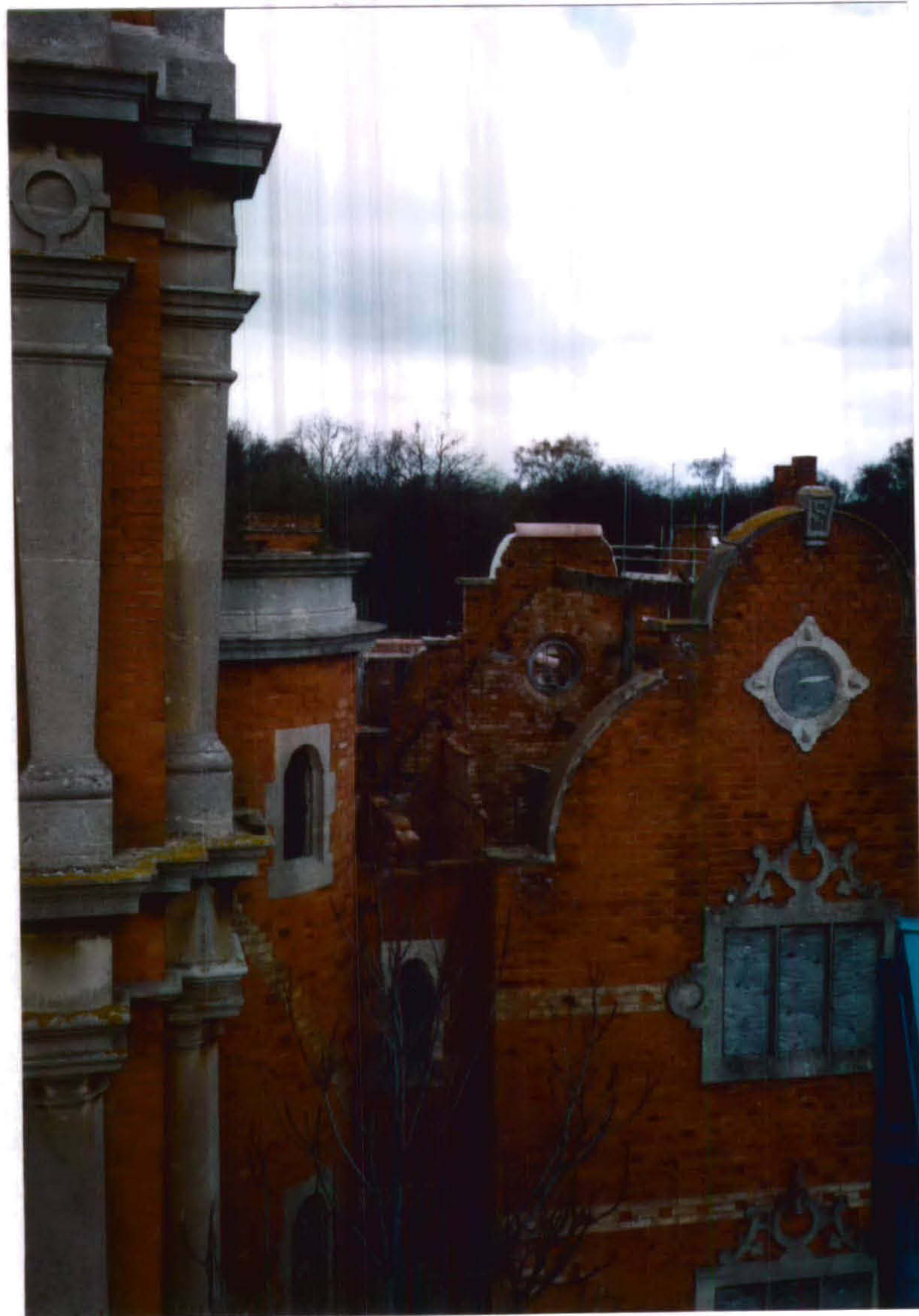
Plate 17 South elevation - detail of Clock Tower and Stair Tower with part of the residential unit showing Dutch Gable with Keytstone to coping carrying 'S' for Stamford and date 1856. The three-light mullions have strapwork ornament above them
