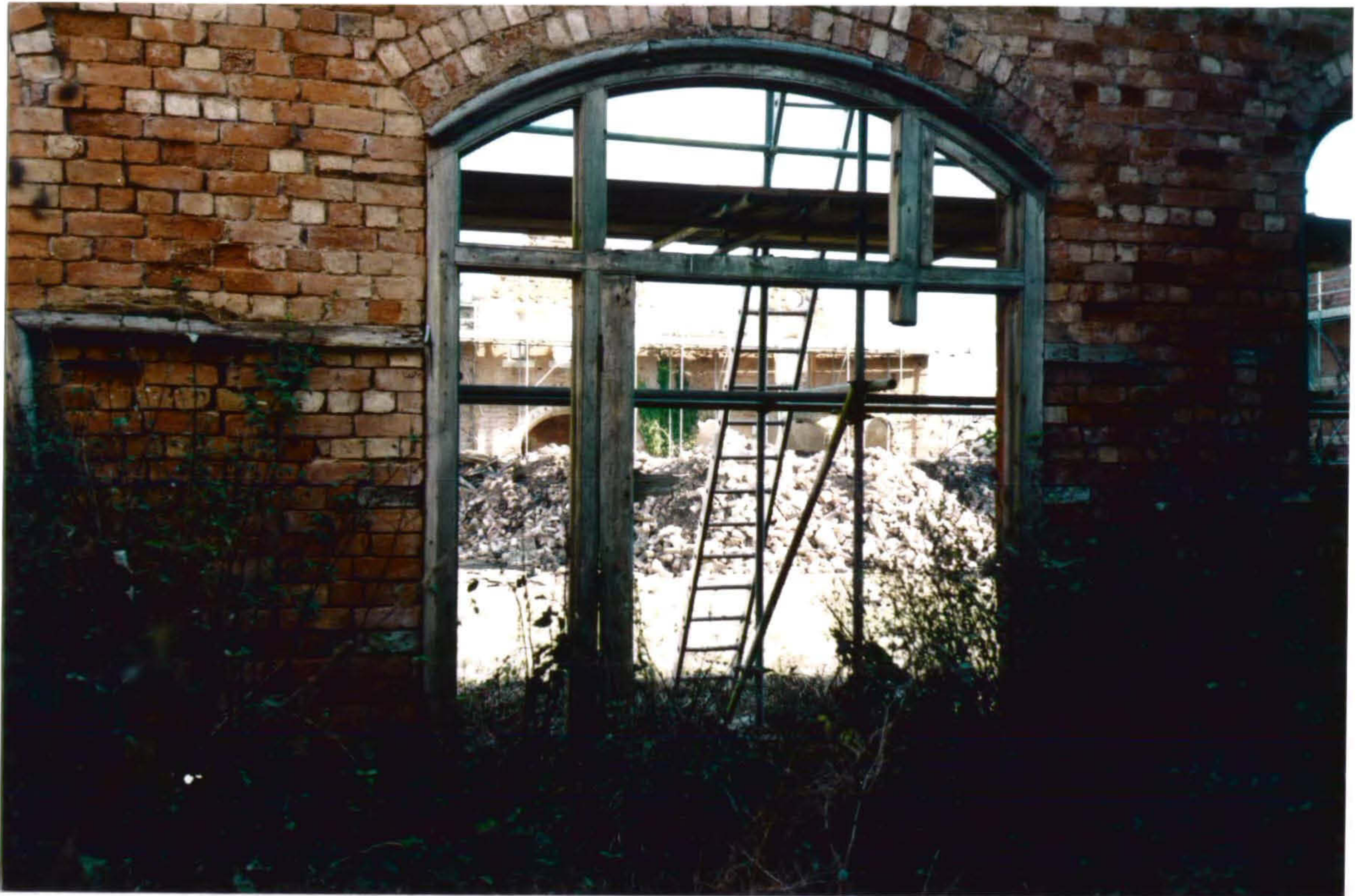
Plate 31 West Range Interior. Surviving section of glazed door frame, (see Drawing 9).
