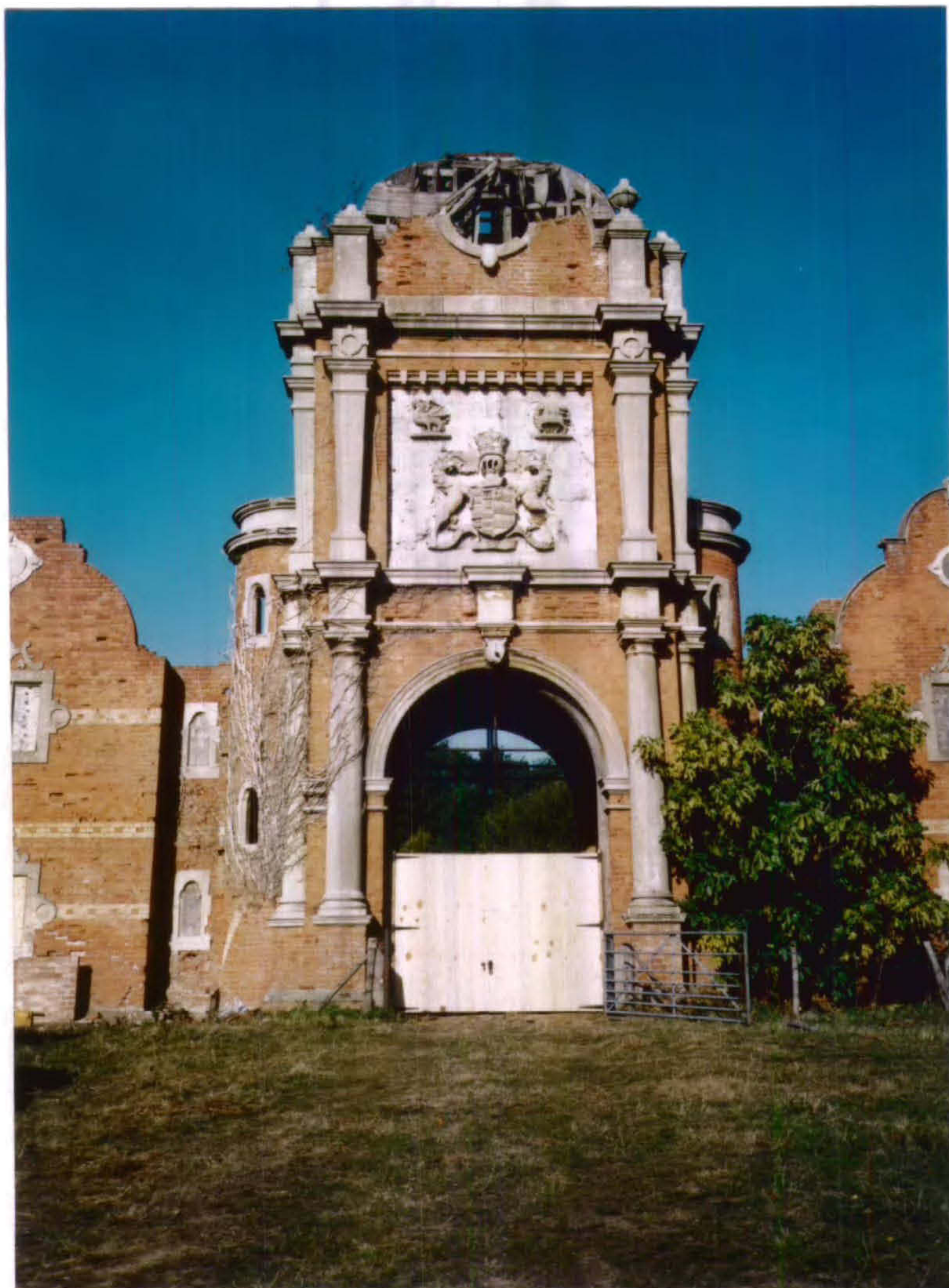
Plate 15 Bradgate Stables : General View Clock Tower entrance with flanking stair towers.
