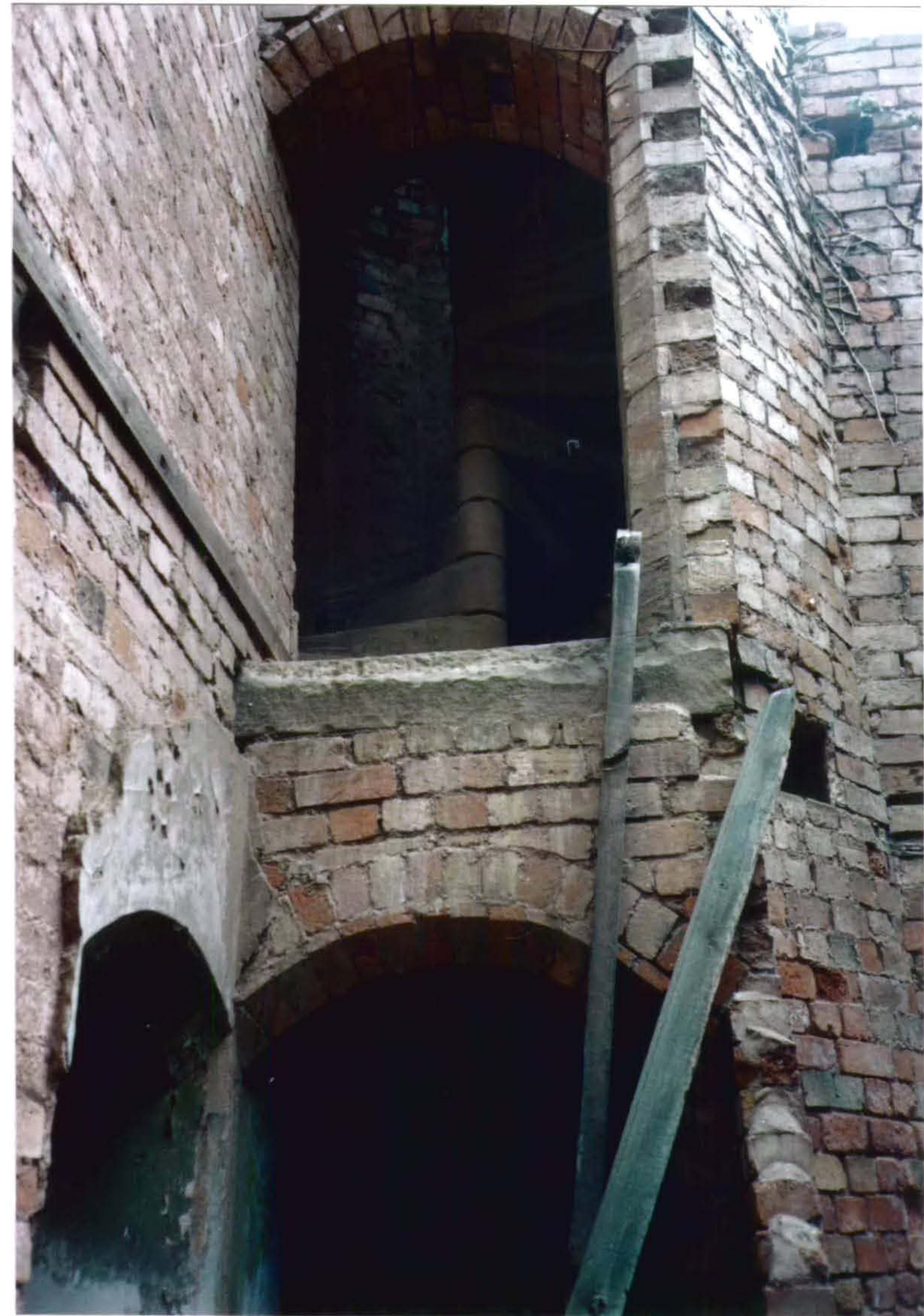
Plate 4 Detail showing the chamfered brick doorways to the Stair Tower of the Clock Tower, South Range. Also shows sandstone newel staircase.
