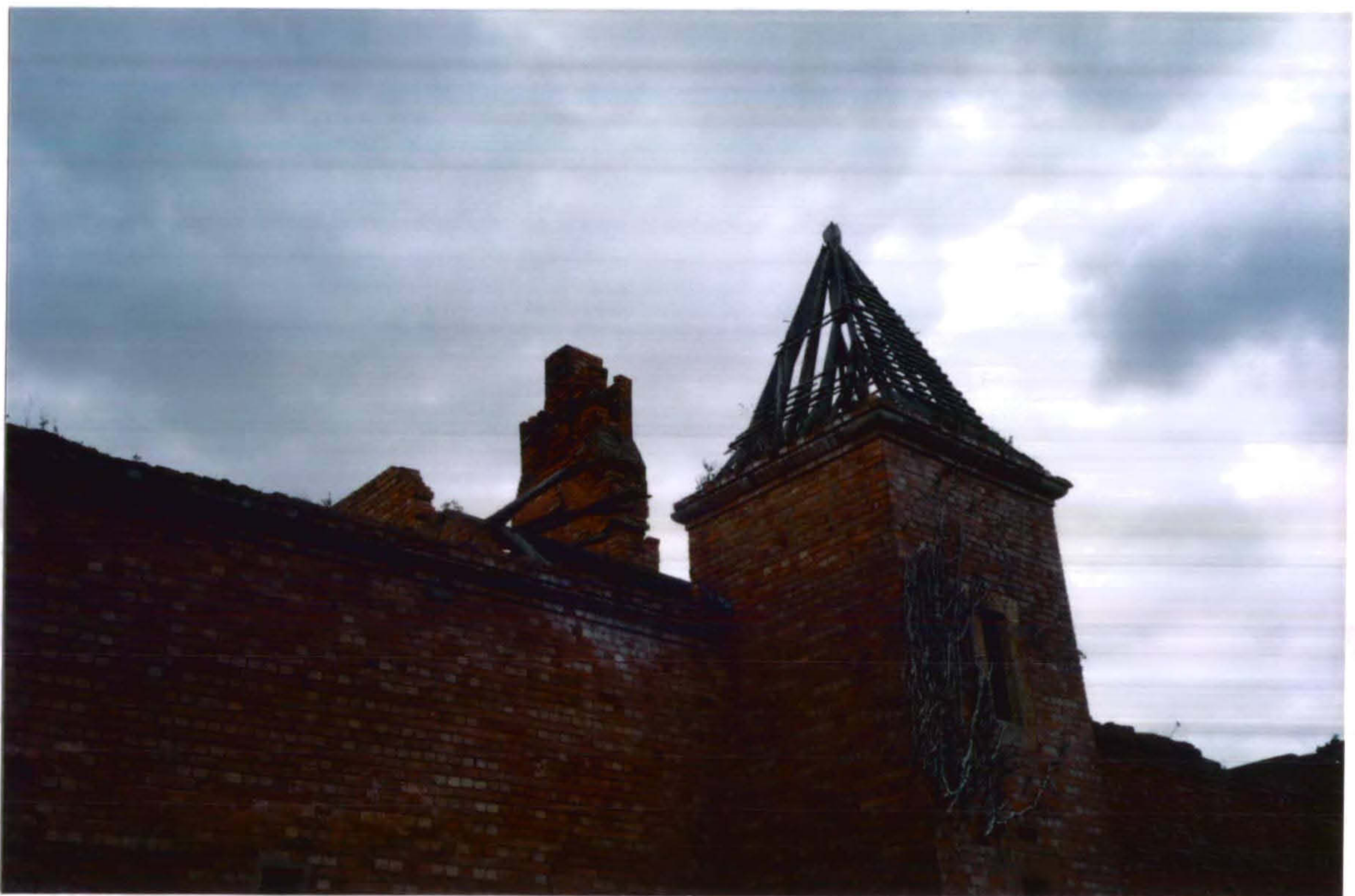
Plate 42 East Range Elevation - showing Stair Tower with pyramidal roof frame still in place, Spring 2004, now removed.
