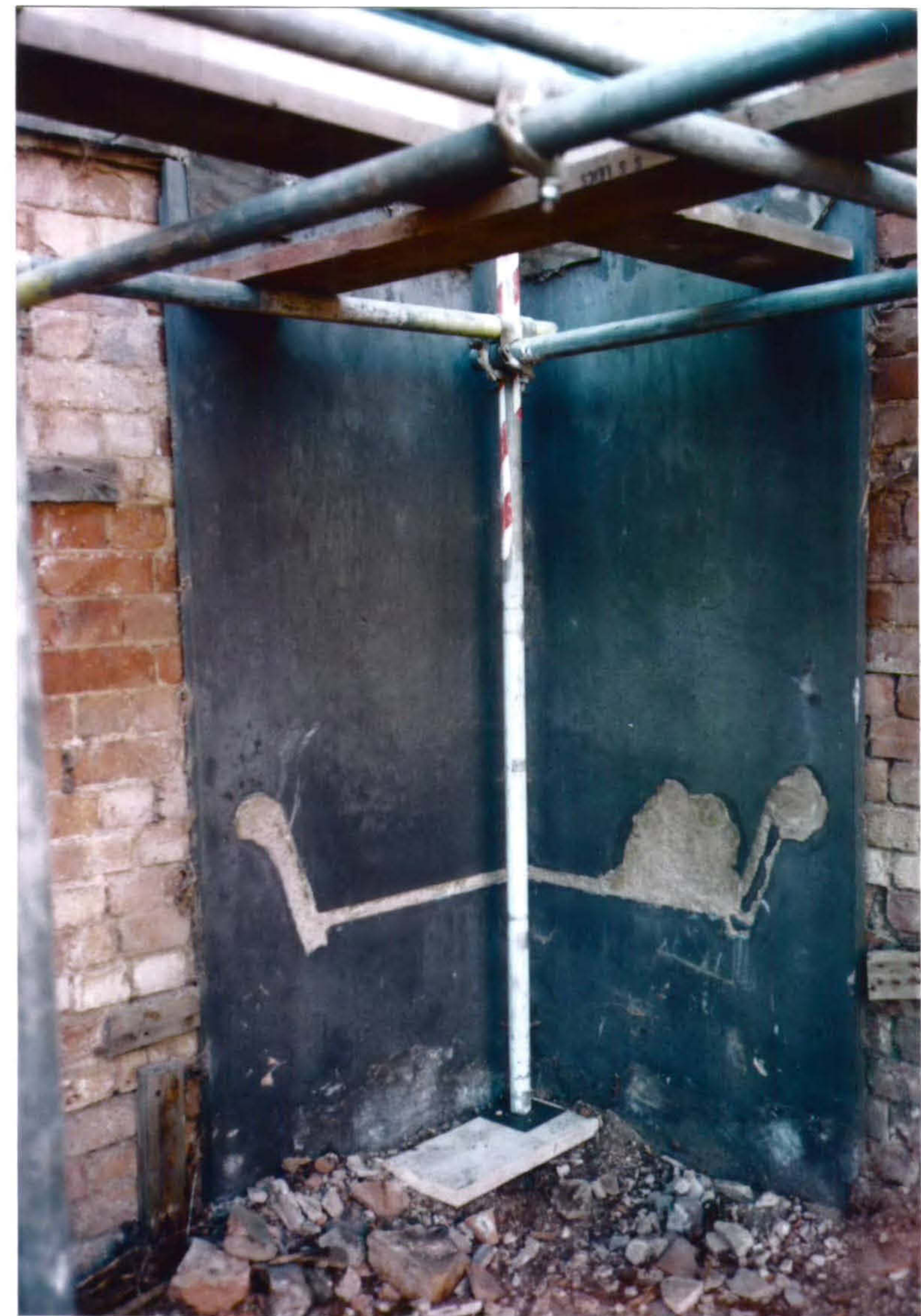
Plates 9 and 10 showing sections of Groby Slate used to line brickwork of the Stables. Both slates have chased out sections for slate manger sections. The slab on the left has a ring for a hay-net installed. Parts of the wooden, wall-mounted battens onto which the slates are mounted can be seen.
