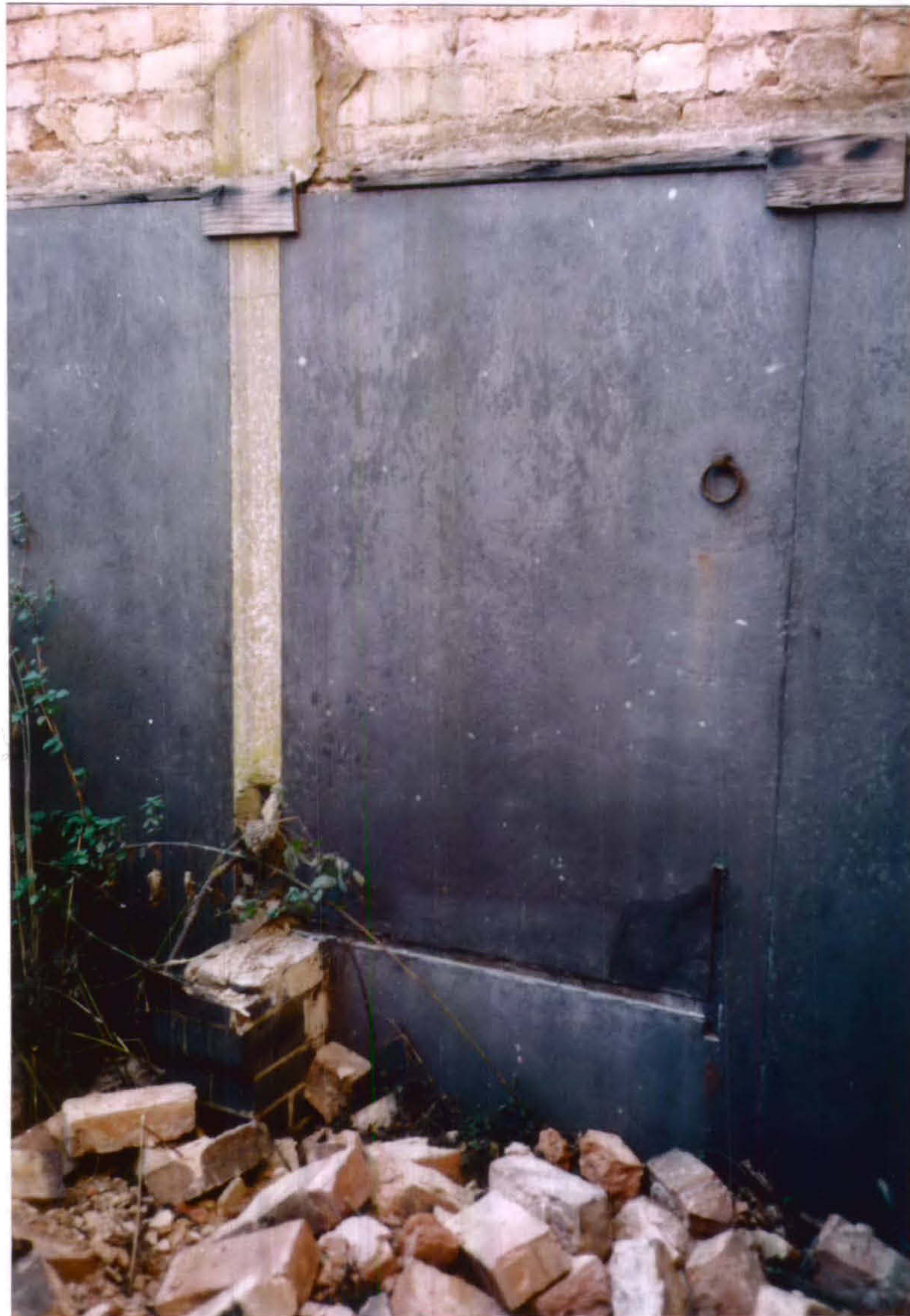
Plates 9 and 10 showing sections of Groby Slate used to line brickwork of the Stables. Both slates have chased out sections for slate manger sections. The slab on the left has a ring for a hay-net installed. Parts of the wooden, wall-mounted battens onto which the slates are mounted can be seen.
