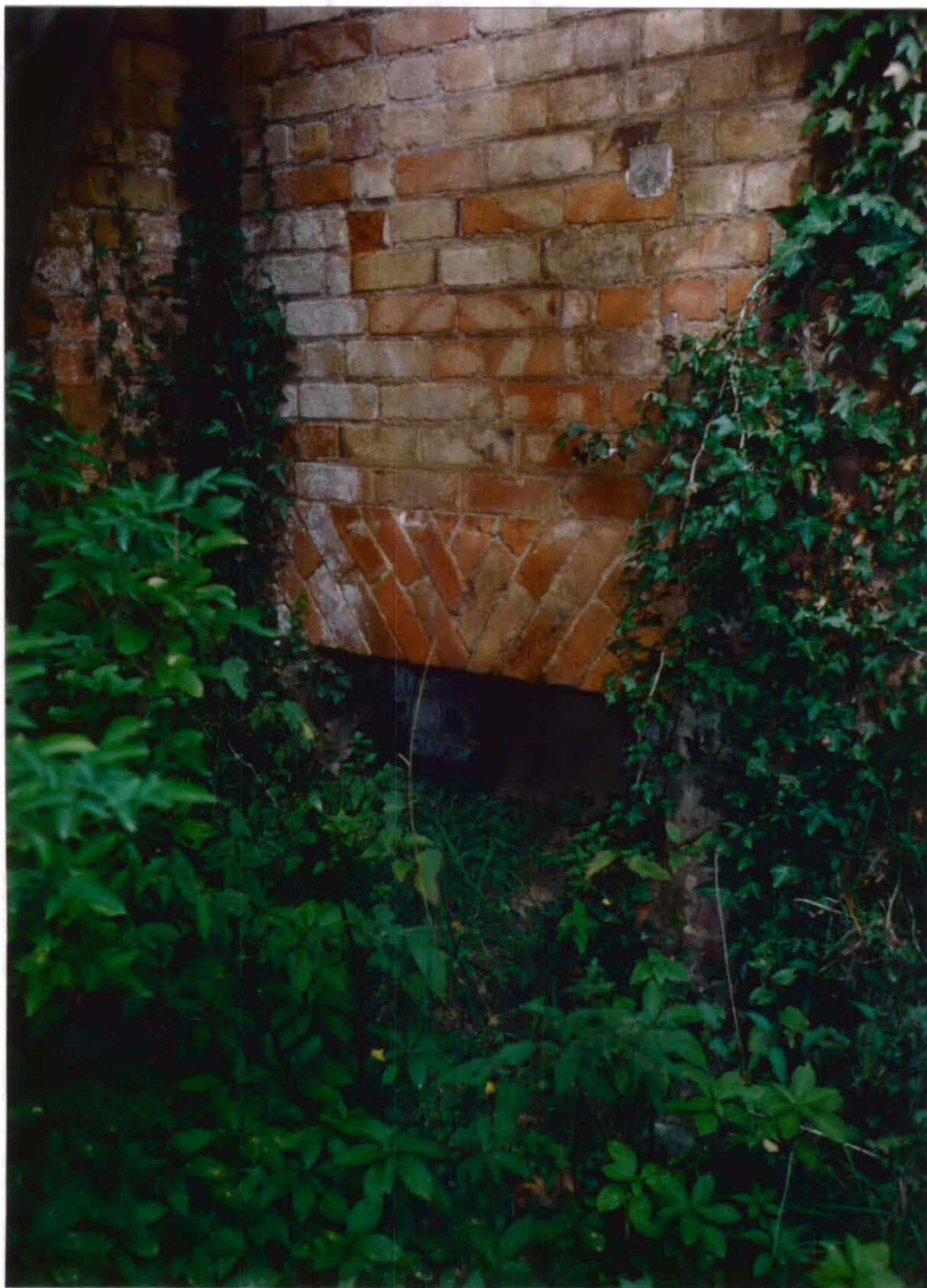
Plate 39 North Range, detail of brick over lintel to fireplace in possible Tack-room in north-west section of the range.
