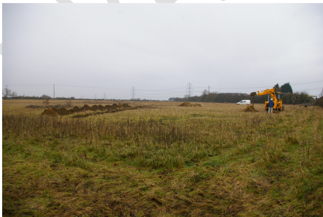
Figure 2: General site view, looking north
