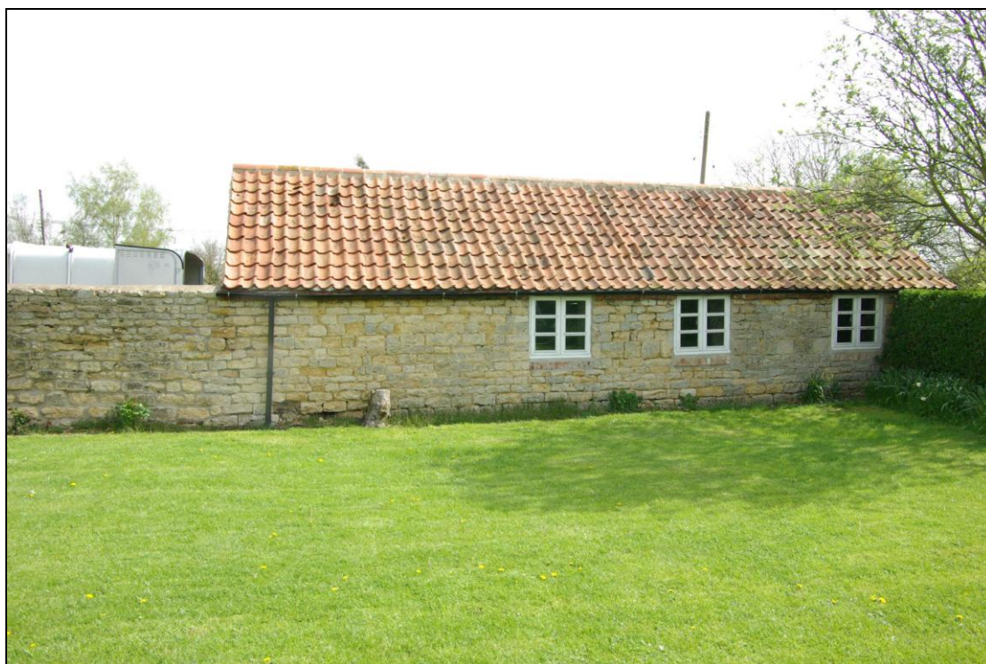
Figure 21. West face of Barn B.
