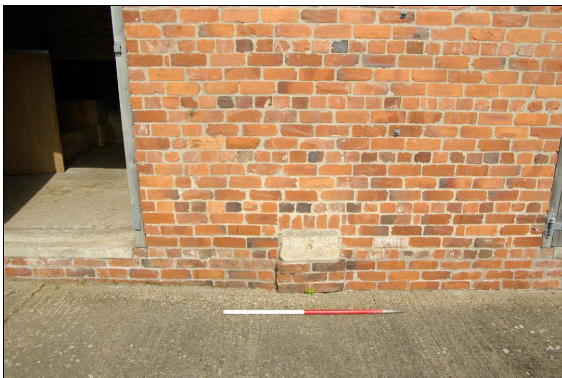
Figure 12. Plinth projecting from south face of Barn A (western section).
