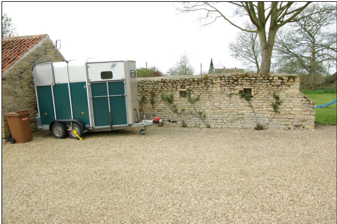
Figure 20. Remaining wall of demolished barn attached to Barn B Looking west.
