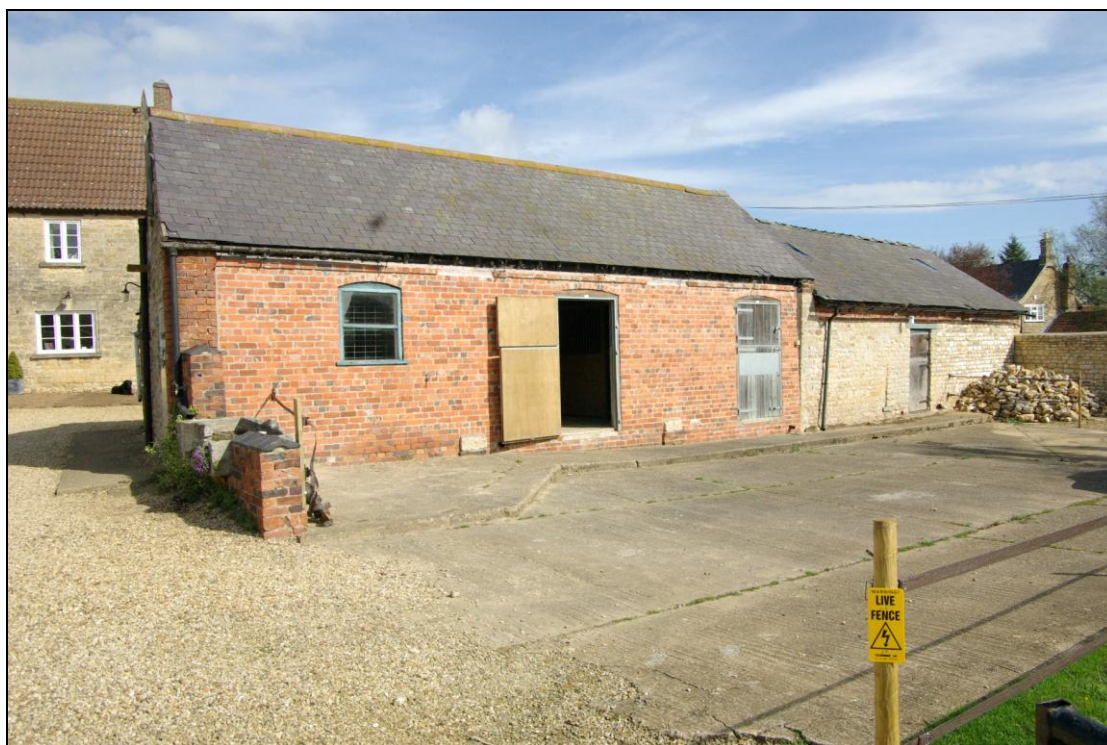
Figure 7. Barn A looking north.
