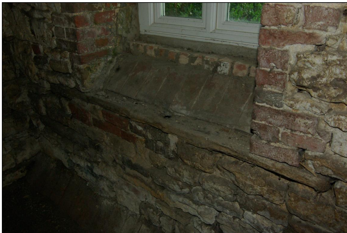
Figure 23. Window detail in Barn B. Looking south-west.
