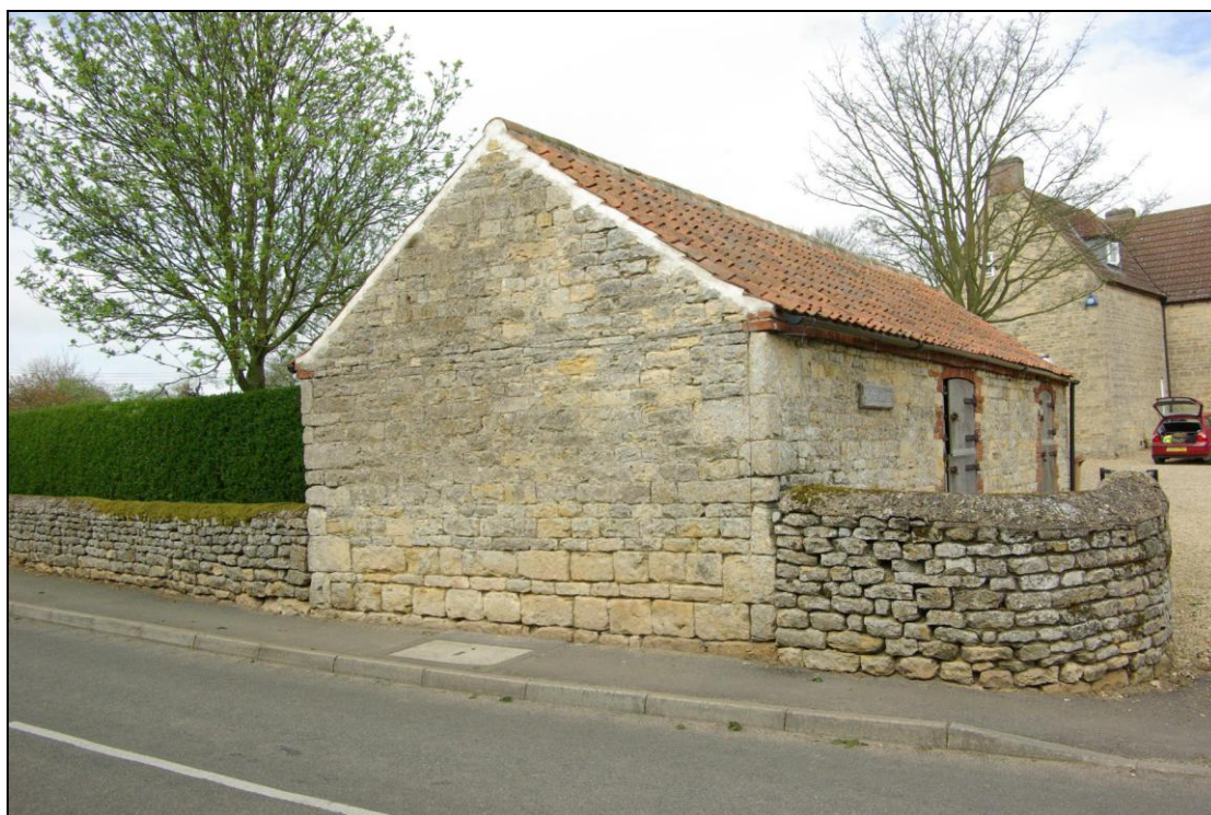
Figure 18. South face of Barn B.
