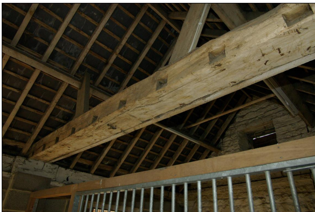
Figure 16. Barn A re-used roof timbers with carpenter's marks.
