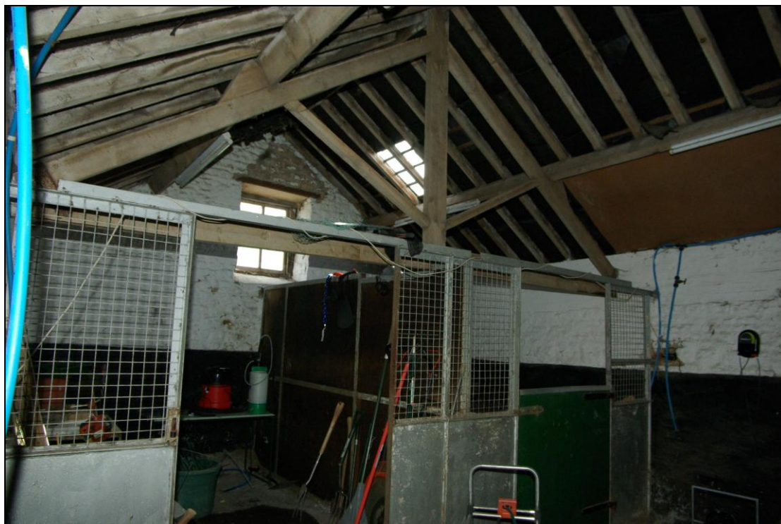
Figure 11. Interior of Barn A (eastern section) looking south-east.
