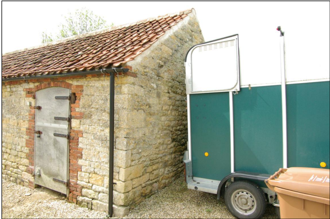
Figure 19. Building scar on Barn B north face.
