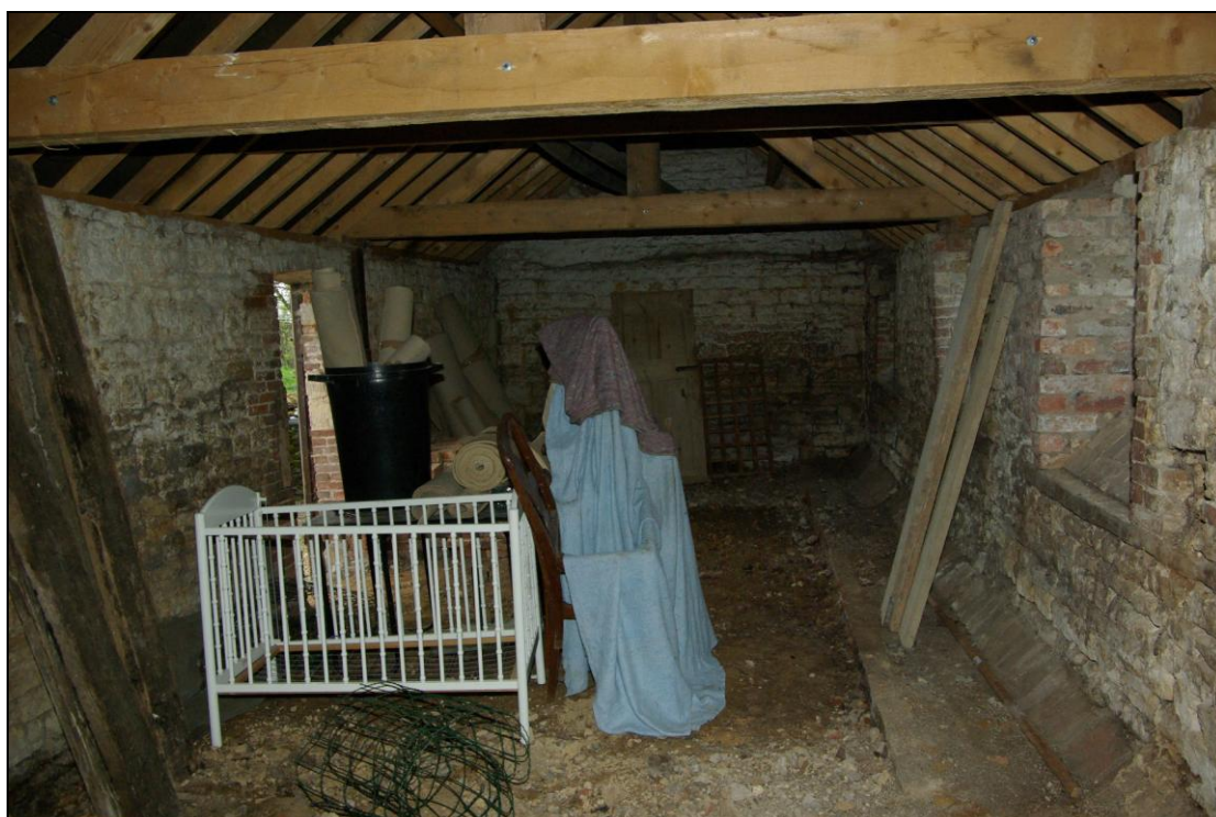
Figure 22. Interior of Barn B looking south.
