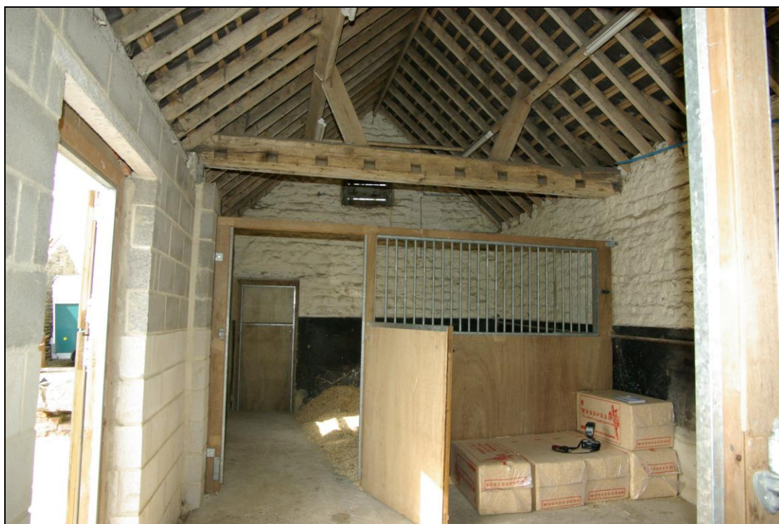
Figure 15. Interior of Barn A (eastern section) looking west.
