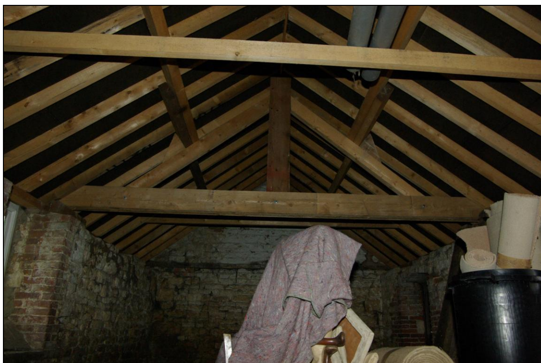
Figure 24. Roof detail Barn B. Looking north.
