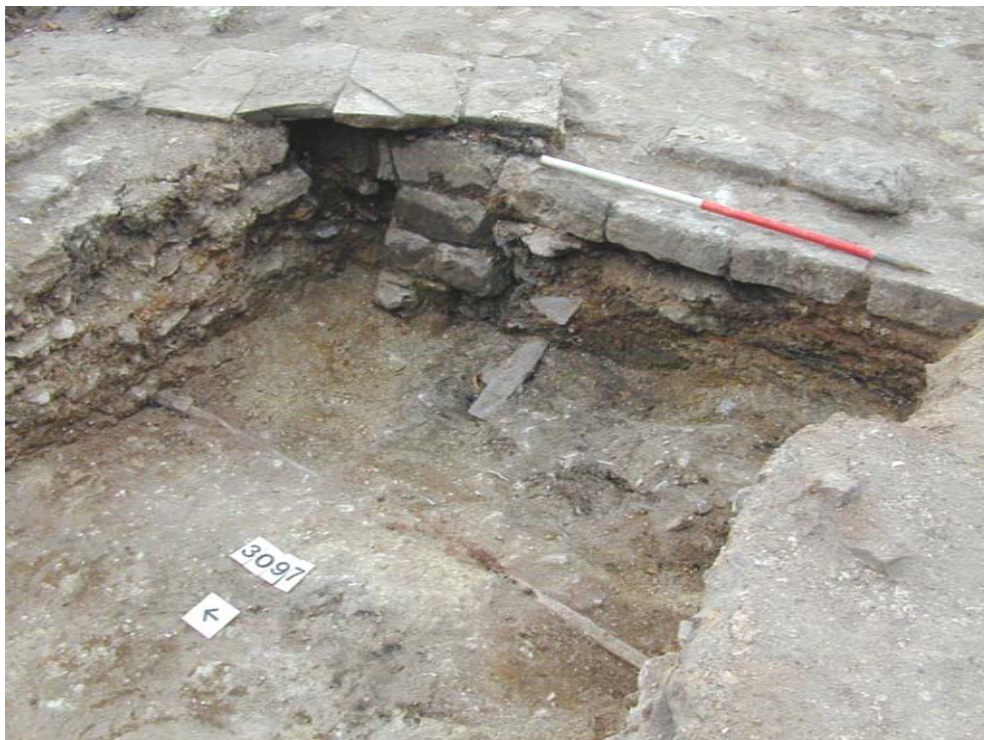
Figure 11 Trench 30: View of the external face of the west wall of the kitchen showing later refacing, the entry point of the slate-capped drain and lead water pipe.
