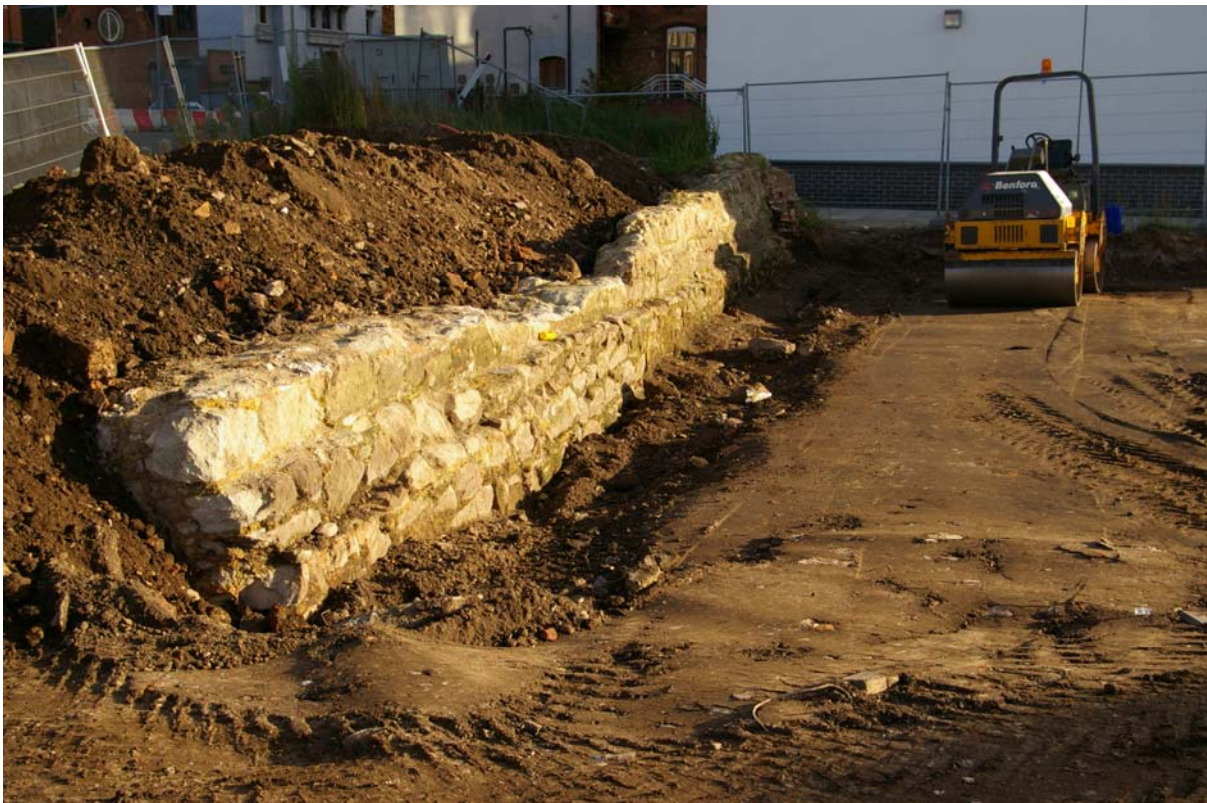
Plate 2 A2.2007 Fragment of the Newark Wall prior to demolition
