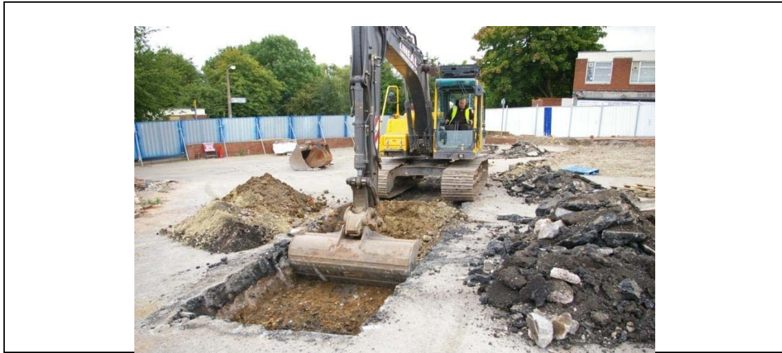
Plate 1: Excavation through overburden
