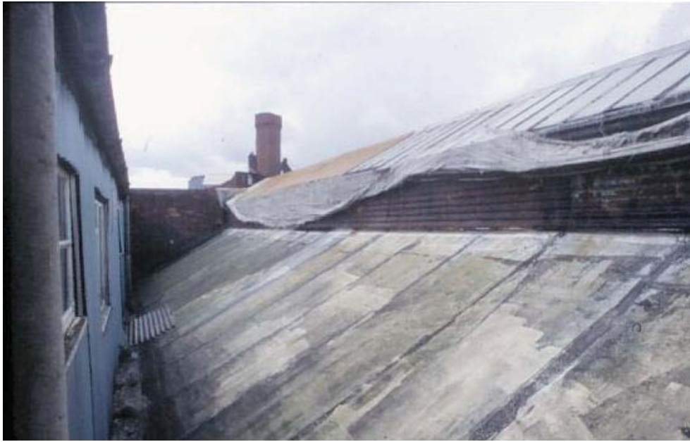
Figure 8 Plot 30(i) External Roof
