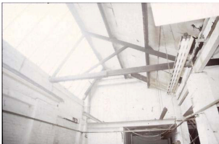
Figure 15 Plot 30 (ii) Roof detail
