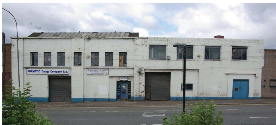
Figure 11 Plot 30 (ii) Lawley Street Middleway Frontage.
