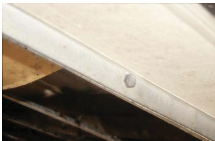
Figure 16 Plot 30 (ii) showing RSJ with makers stamp
