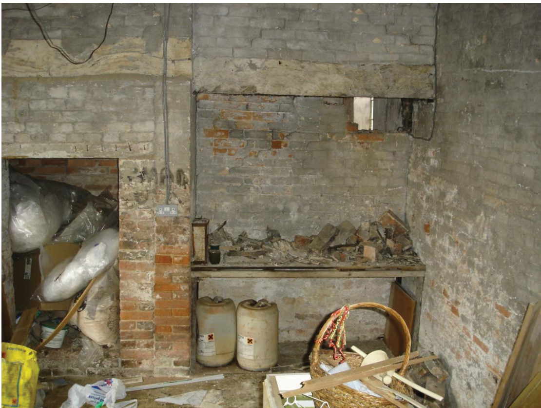
Figure 22 Stable fireplace, note reused lintel on left of picture Looking west
