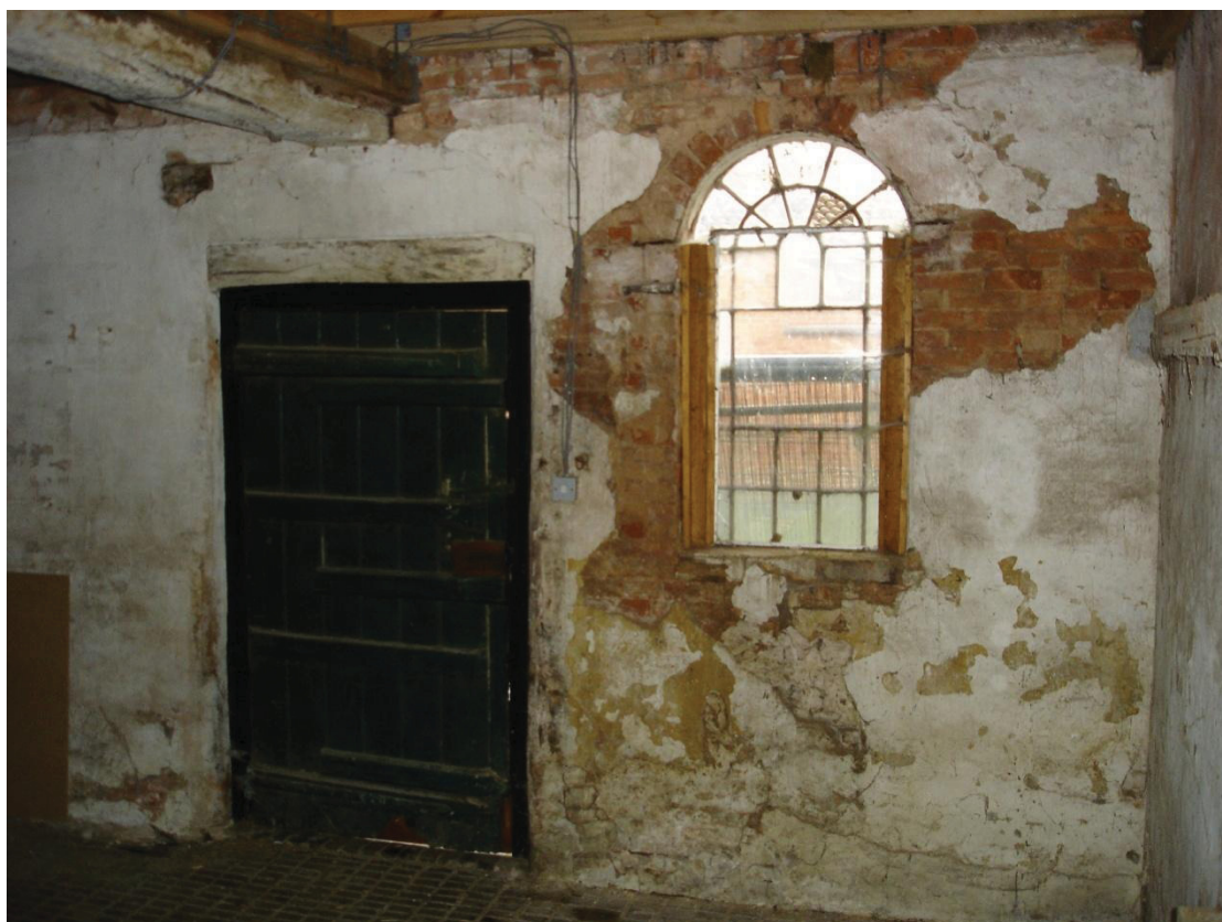
Figure 19 Stable window and door detail Looking east
