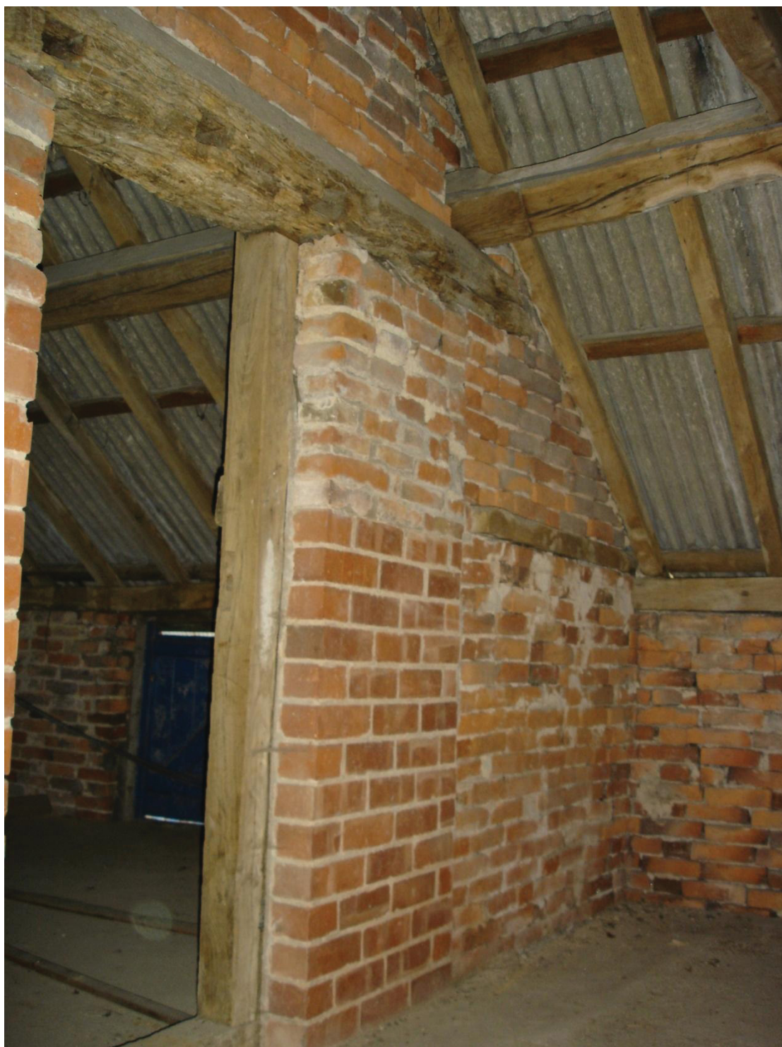
Figure 24 Room 1 dividing wall into Room 2 Looking north-east
