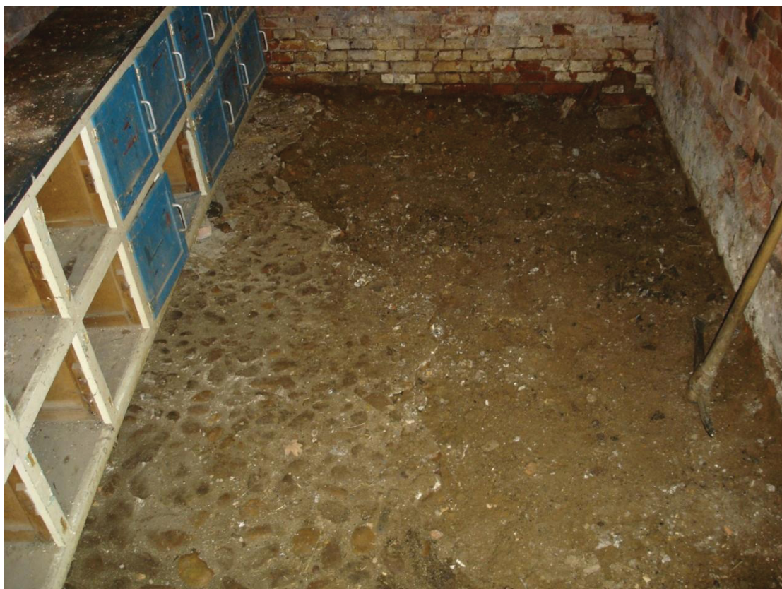
Figure 17 South end room floor being removed Looking west
