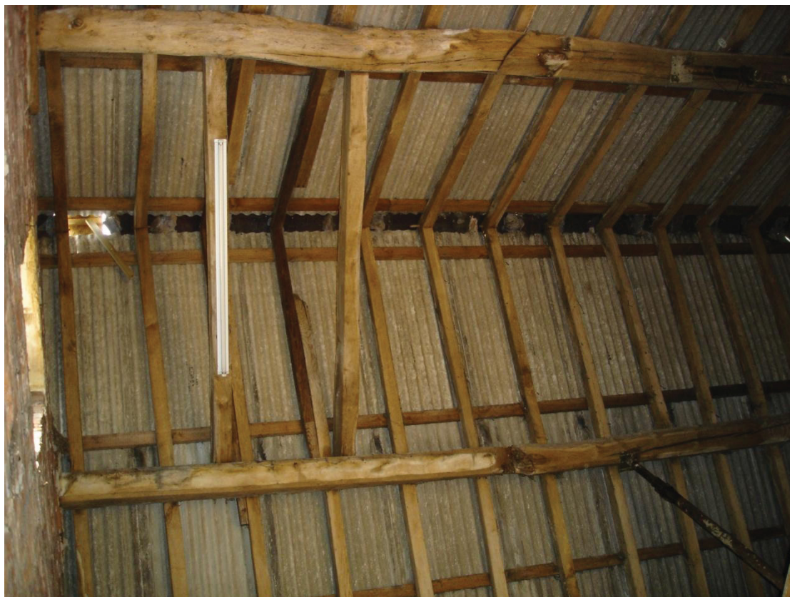
Figure 23 Roof detail of Room 1
