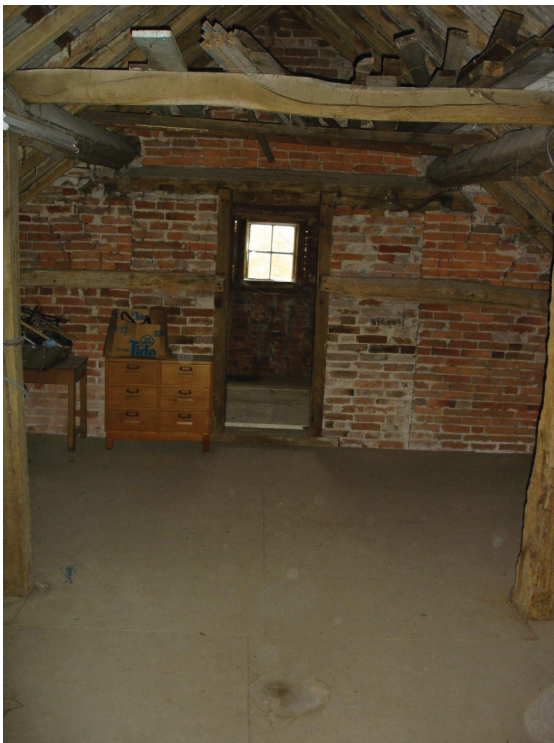
Figure 25 Room 2 dividing wall to Room 1, note purlin supports Looking south
