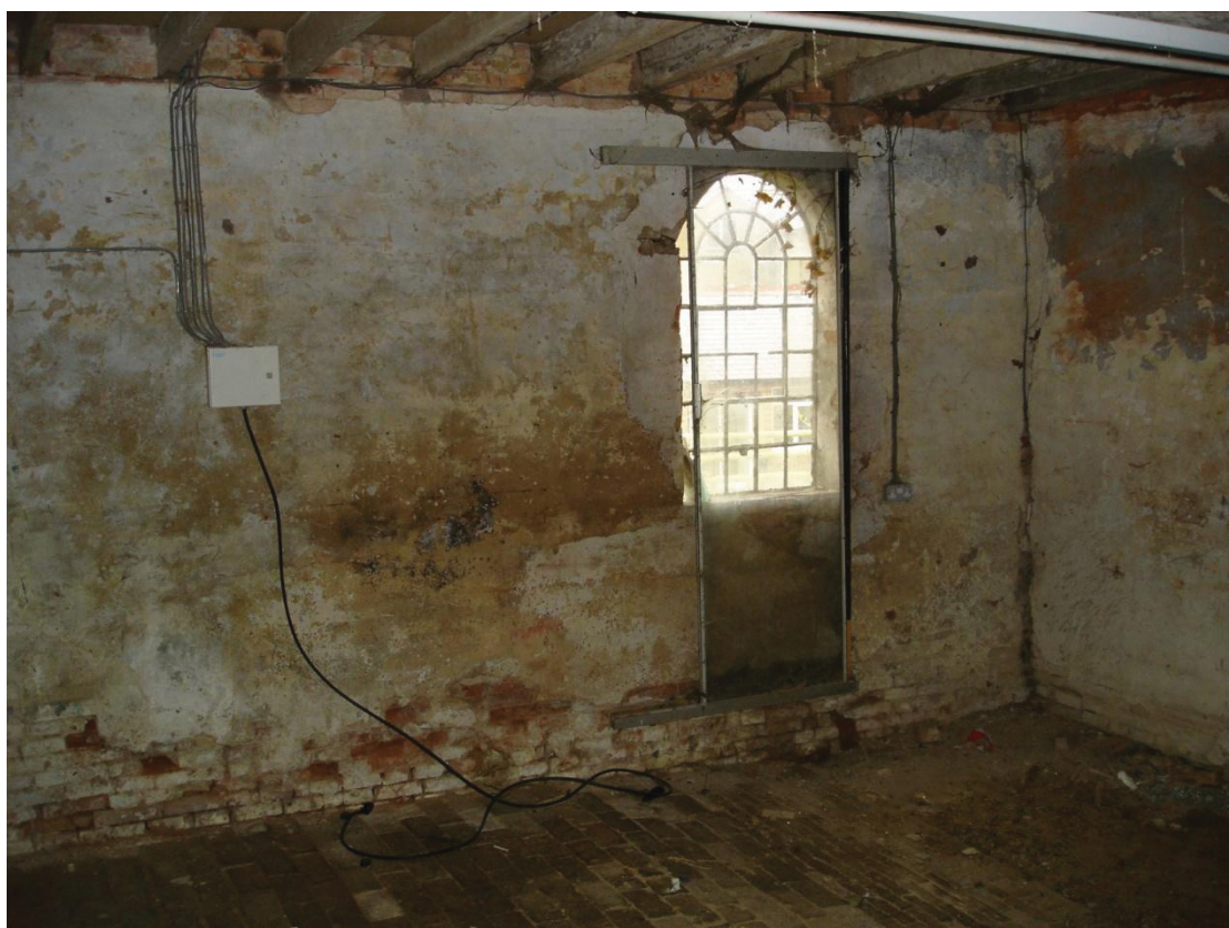
Figure 20 North-east corner room Looking north-east
