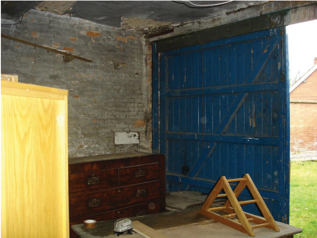
Figure 21 Outside doors of coach store, note wooden pegs on wall Looking south-east
