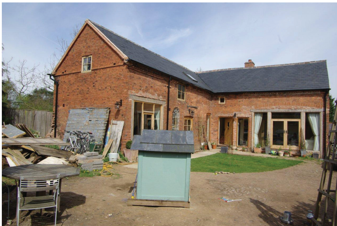
Figure 16 Southern end of building with wall stub visible Looking north-west
