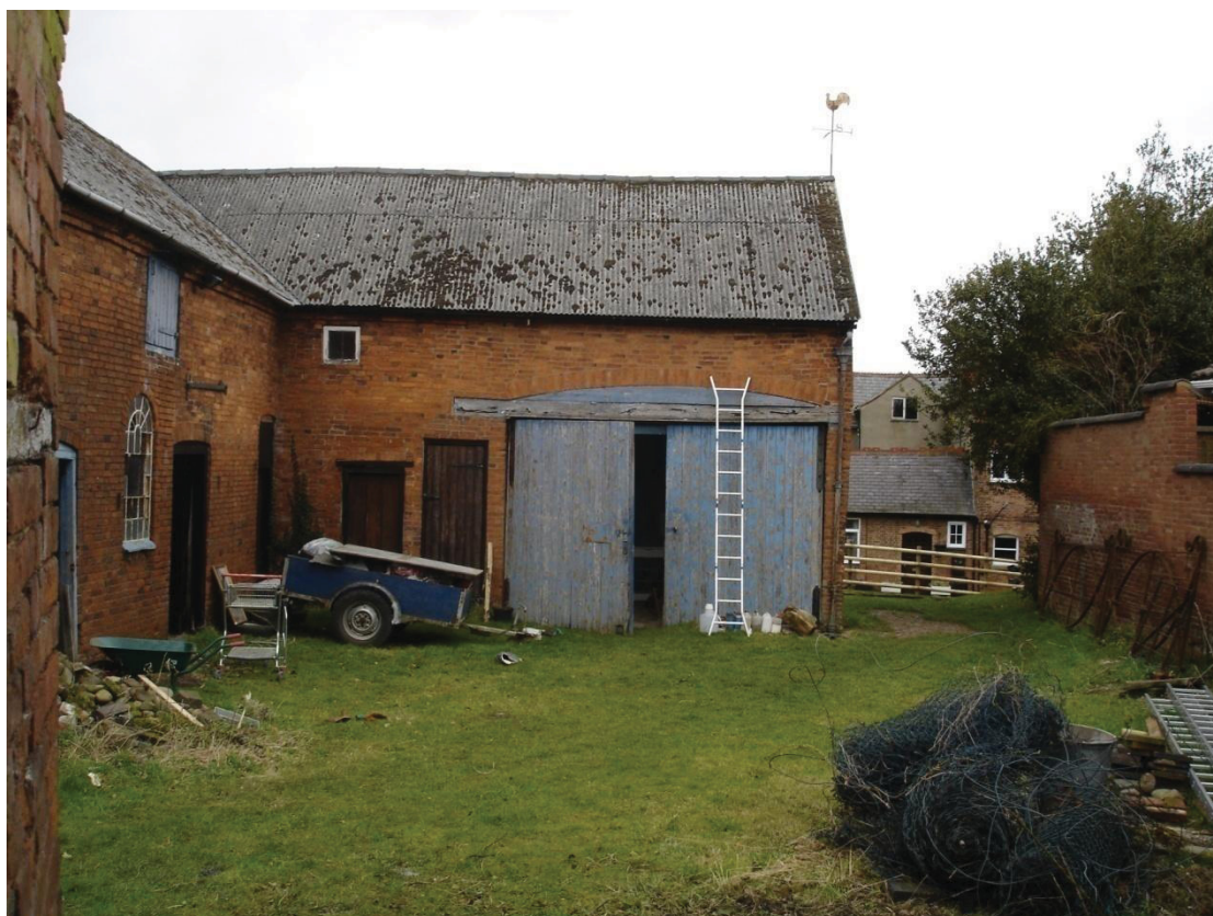
Figure 13 South elevation of east to west wing before renovation Looking north
