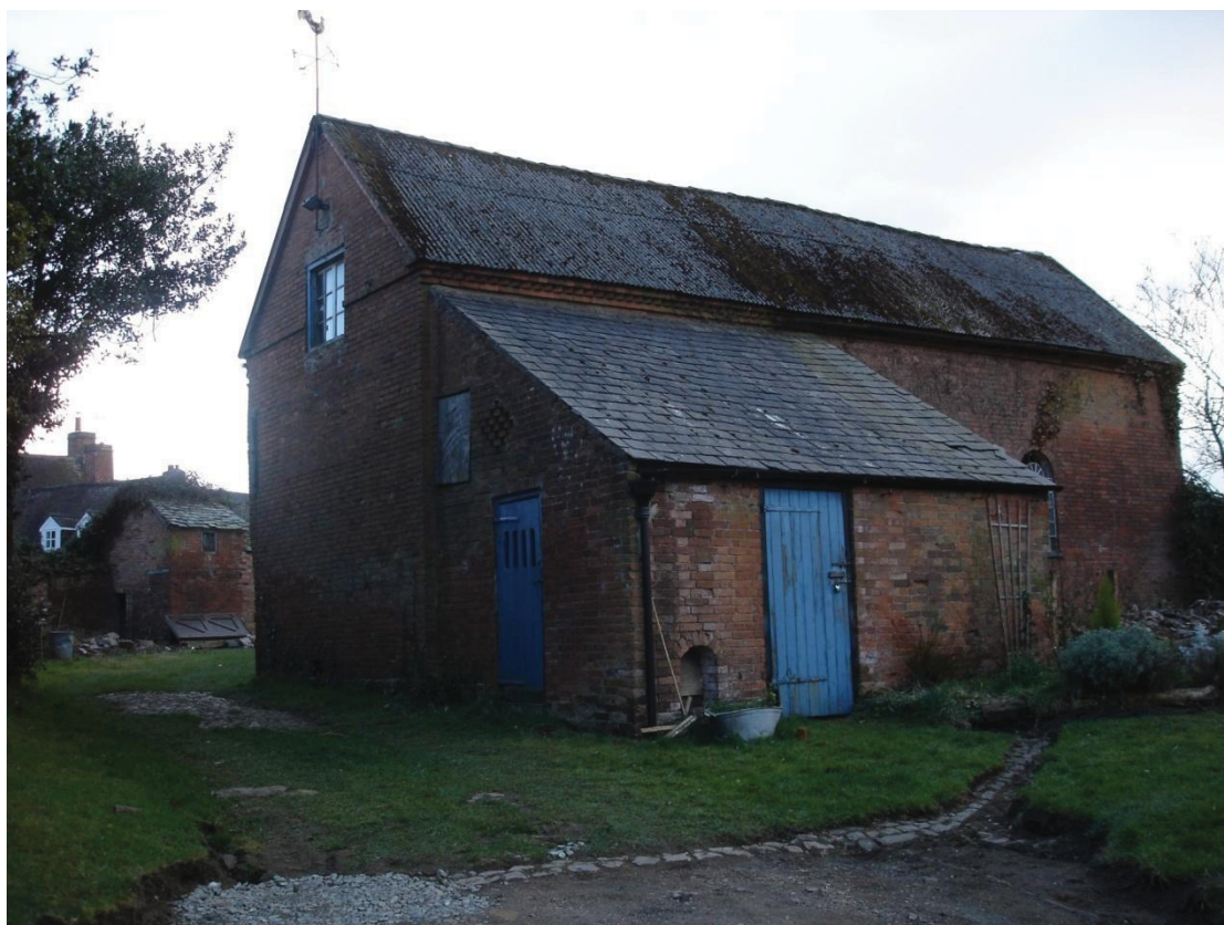
Figure 9 North and east elevations before renovation Looking south west
