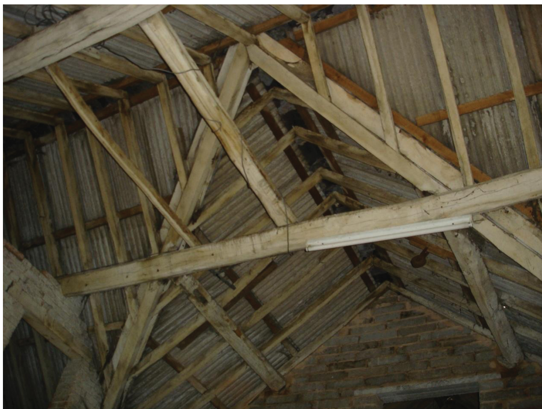
Figure 26 Room 4 roof detail at junction of the two wings Looking south-east
