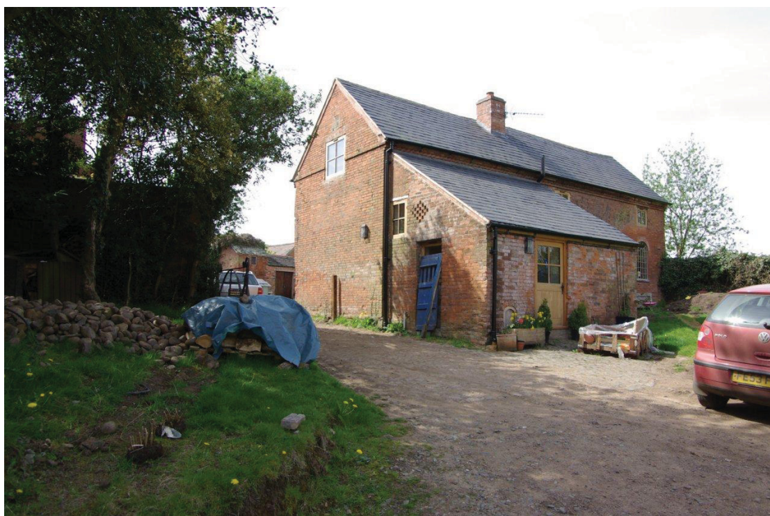
Figure 7 Coach House from the entrance drive (after renovation) Looking south west
