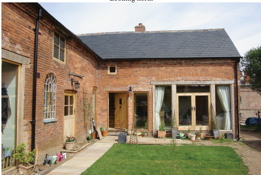
Figure 14 South elevation of east to west wing after renovation Looking north
