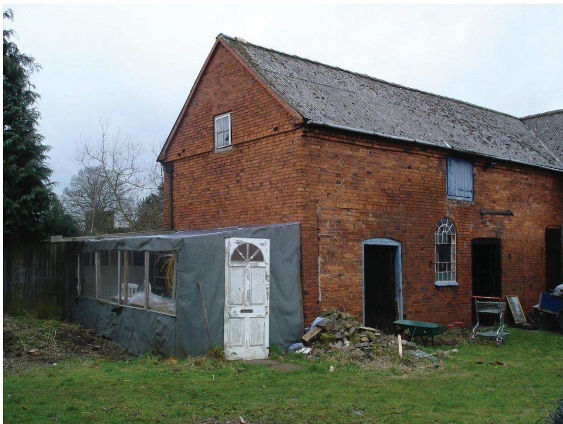
Figure 15 East and south elevations of north to south wing before renovation Looking north-west
