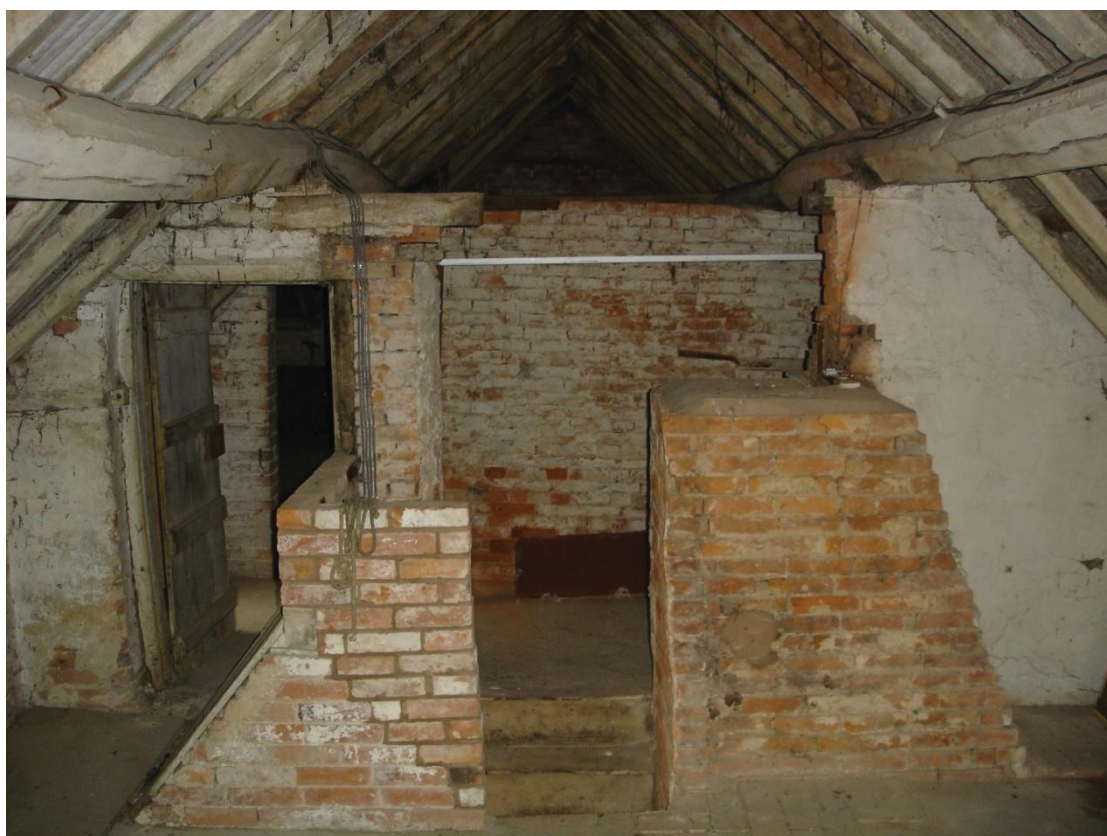
Figure 27 Room 6, top of stairs and capped chimney Looking west
