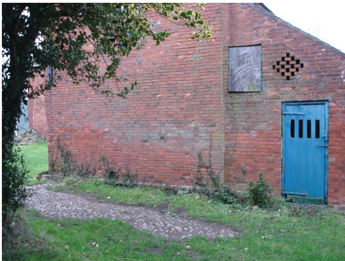
Figure 12 East elevation and lean-to Looking south-west
