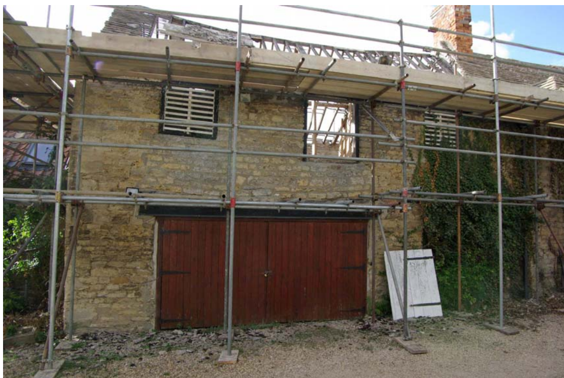
Figure 11 Outbuilding Facing west
