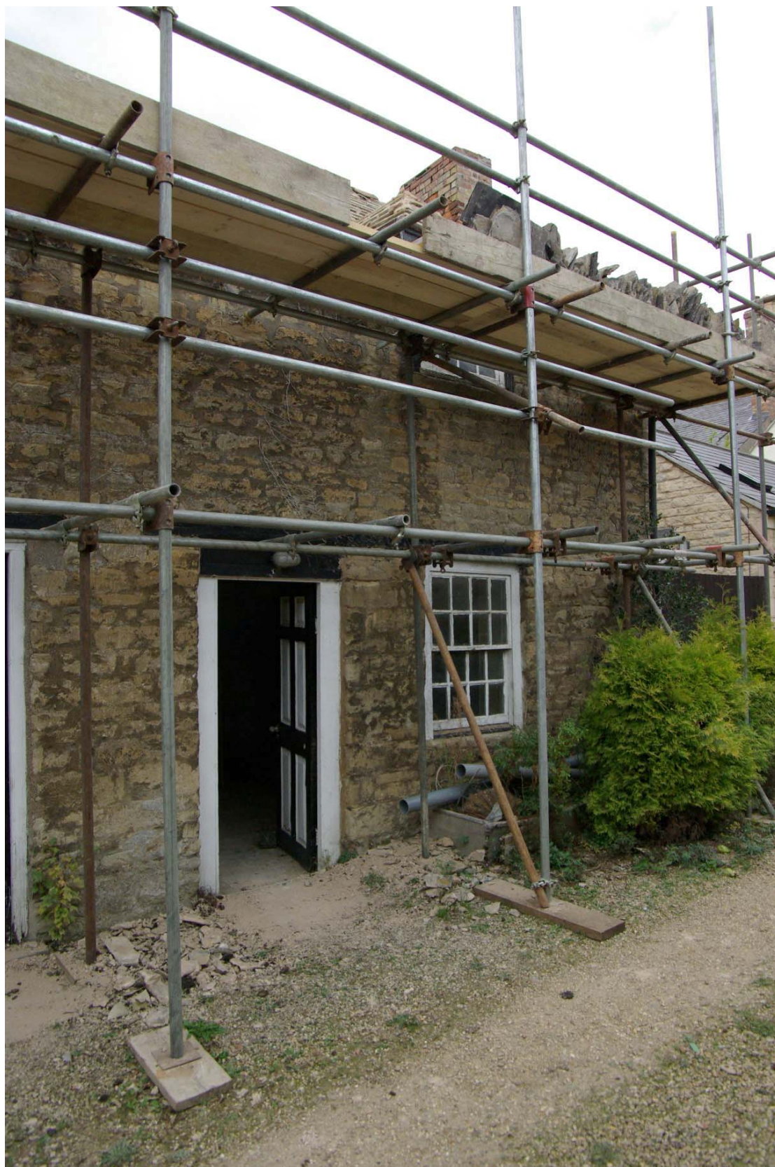
Figure 9 Number 1 Setchells Yard Facing north west
