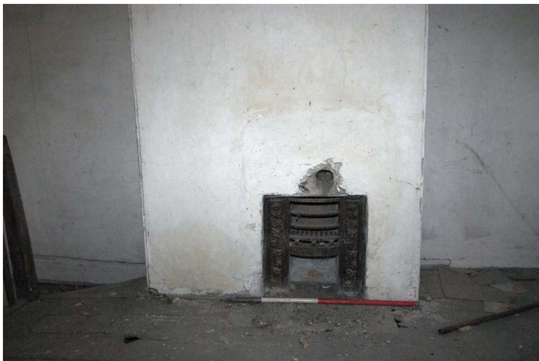
Figure 22 Number 1, first floor. Pantheon fire grate Facing north, 1m scale
