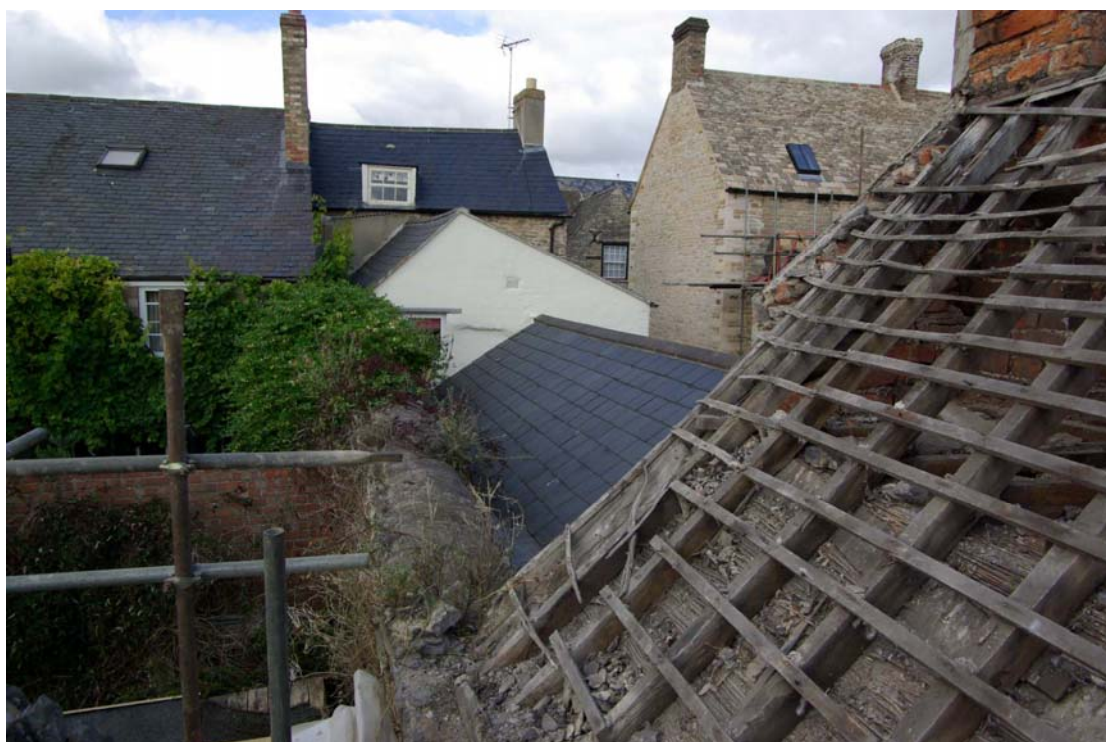
Figure 13 Continuation of western wall from number 1 towards West Street Facing north
