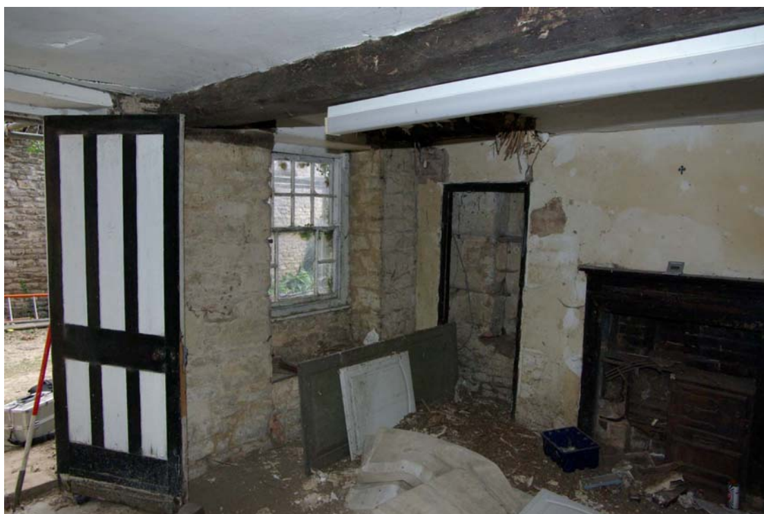
Figure 23 Number 2, ground floor Facing south east
