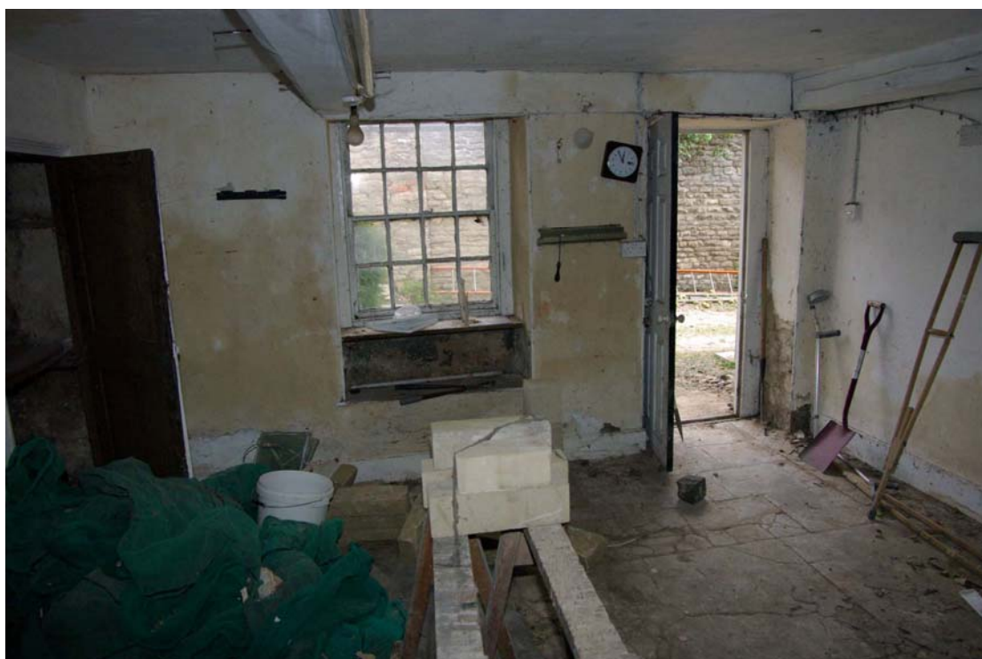
Figure 19 Number 1, ground floor Facing south east
