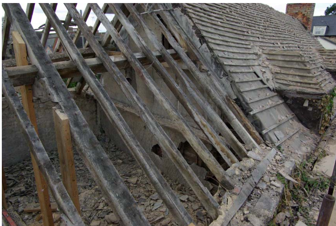
Figure 17 Roof structure of outbuilding Facing north west
