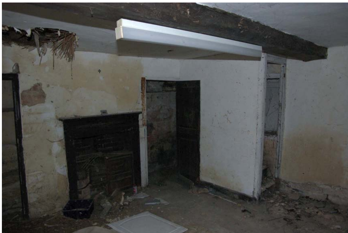
Figure 24 Number 2, ground floor Facing south west
