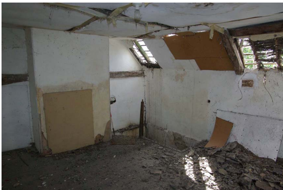
Figure 25 Number 2, first floor Facing south west
