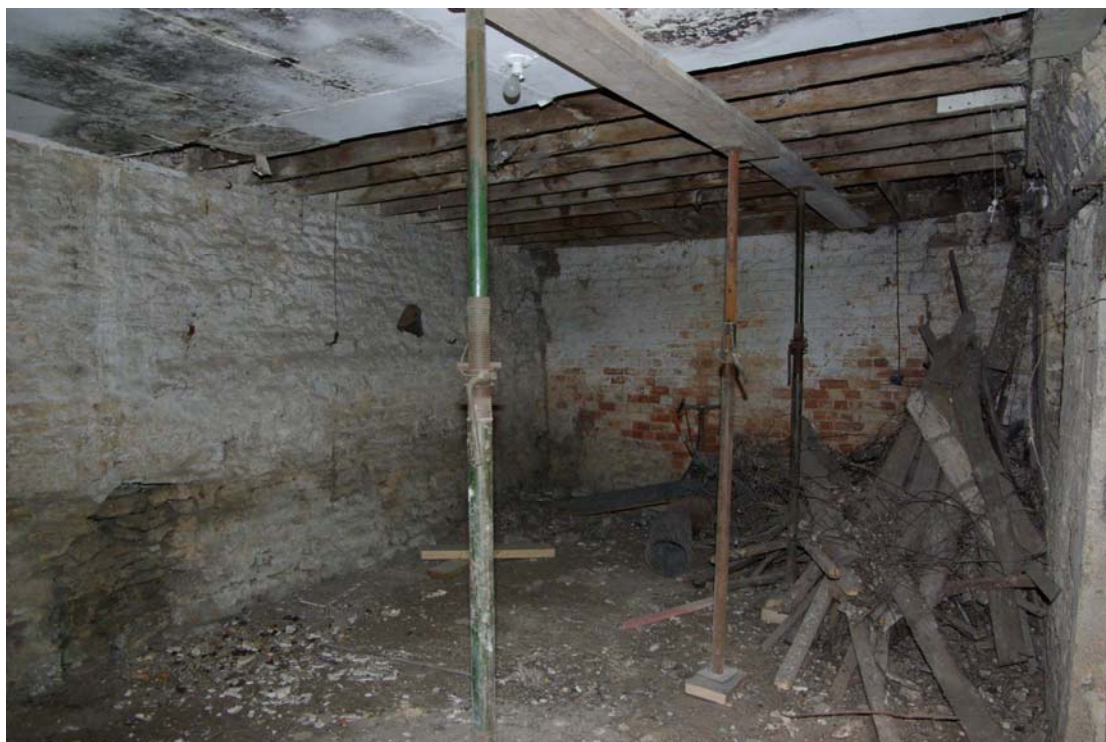
Figure 26 Outbuilding, ground floor Facing north west
