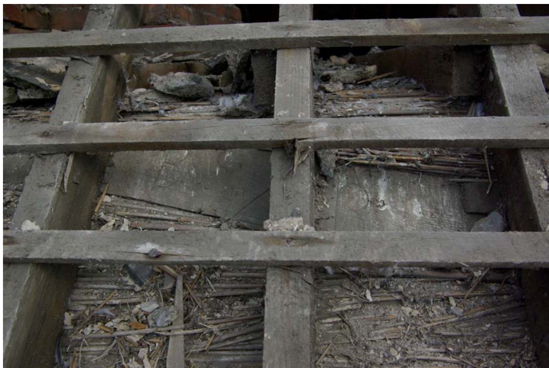
Figure 16 Marks on northern purlin of number 1 Facing east
