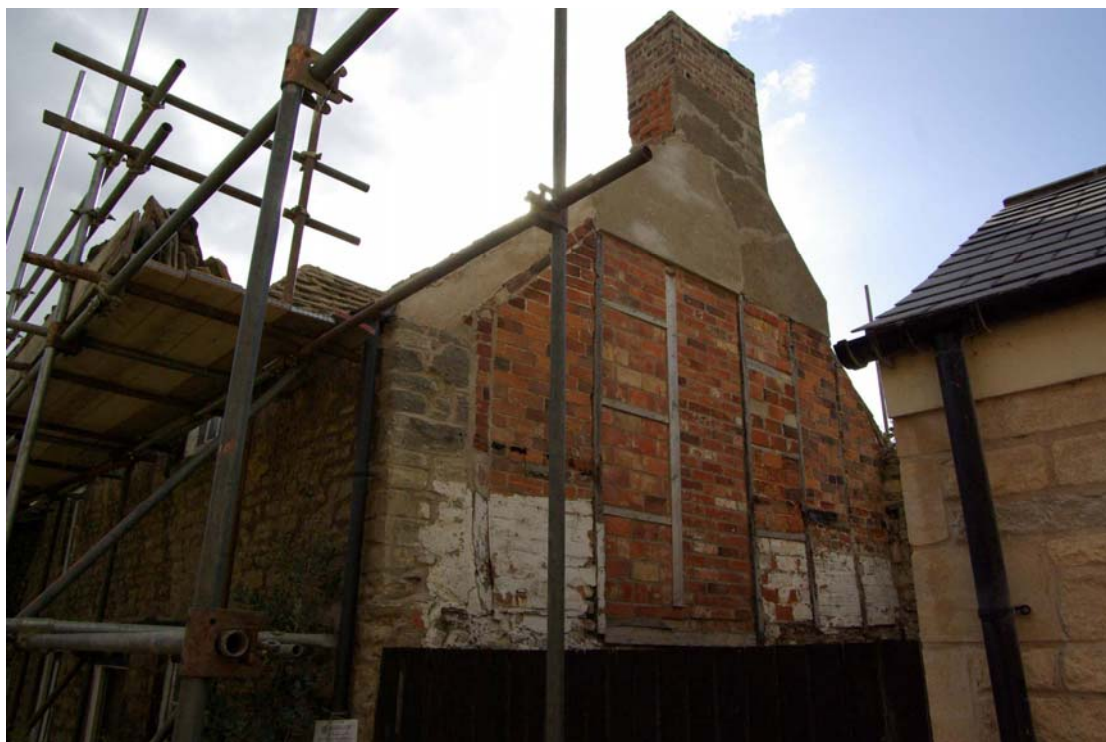
Figure 14 North elevation Facing south west
