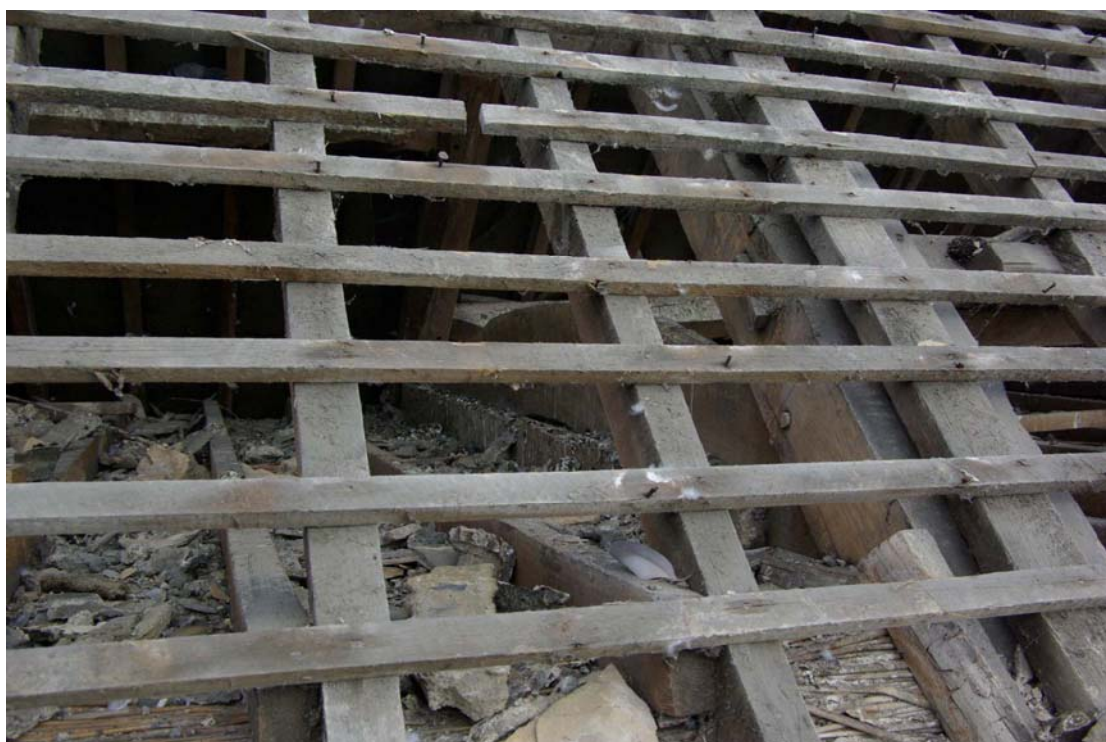
Figure 15 Collar and pegged purlin, number 1 Facing south east
