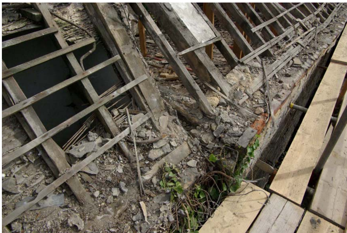
Figure 12 Butt joint between outbuilding and number 2, west wall Facing south east
