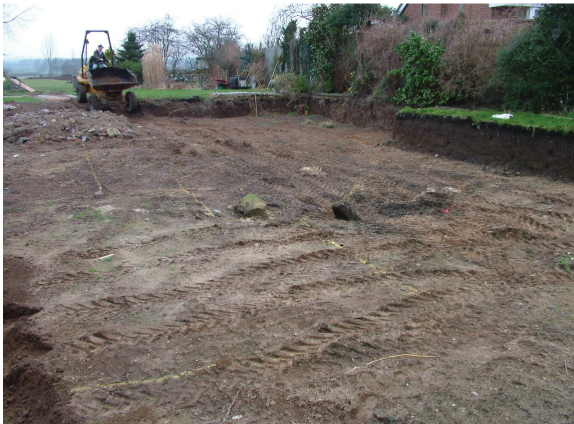
Plate 1: The site on arrival with topsoil removed, looking north
