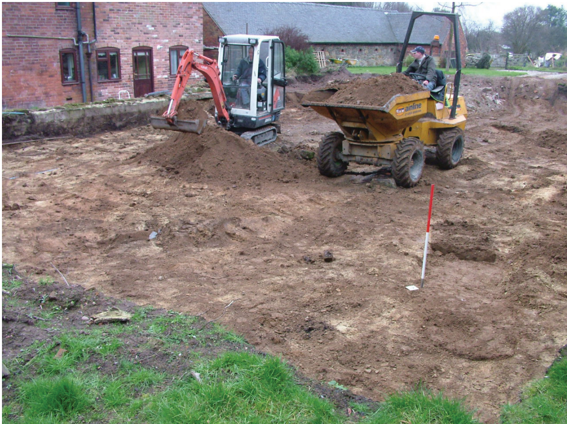
Plate 4: Stripping almost completed, showing natural clay beneath soils, looking north-west
