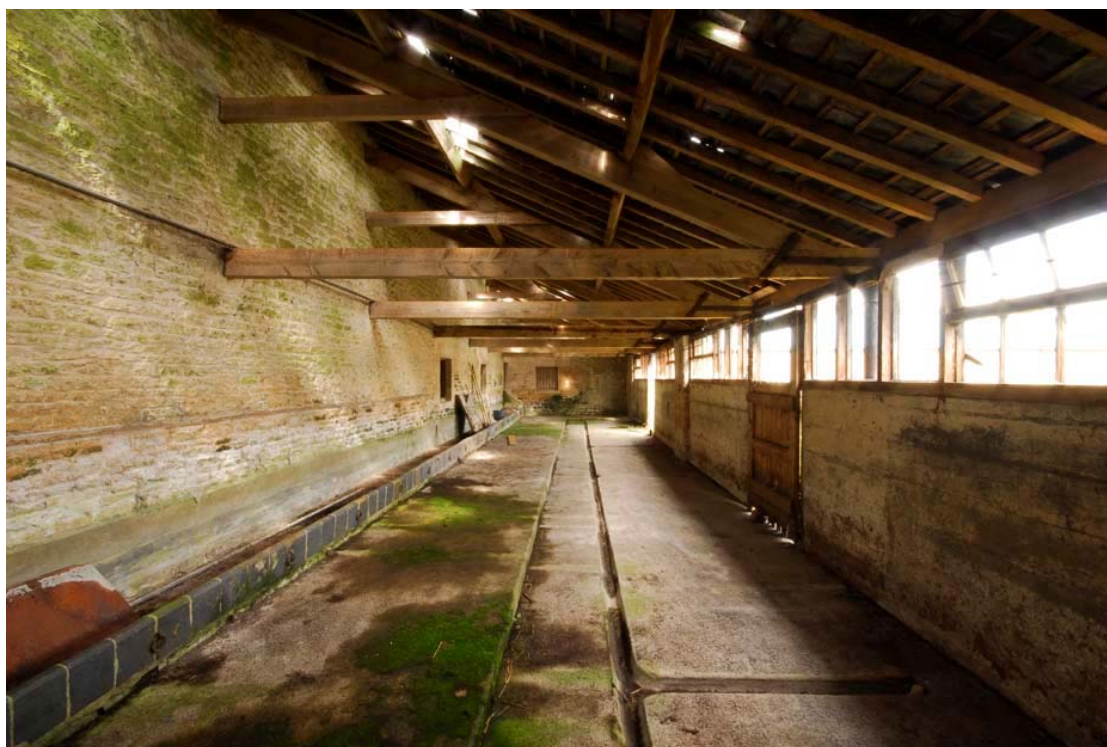
Figure 36 Room 9 Looking east
