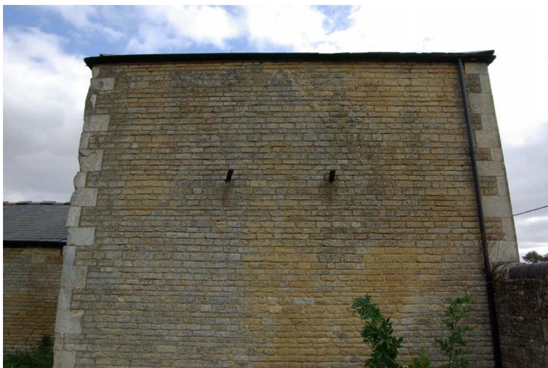
Figure 23 Courtyard 2 central building west elevation and building scar Looking east
