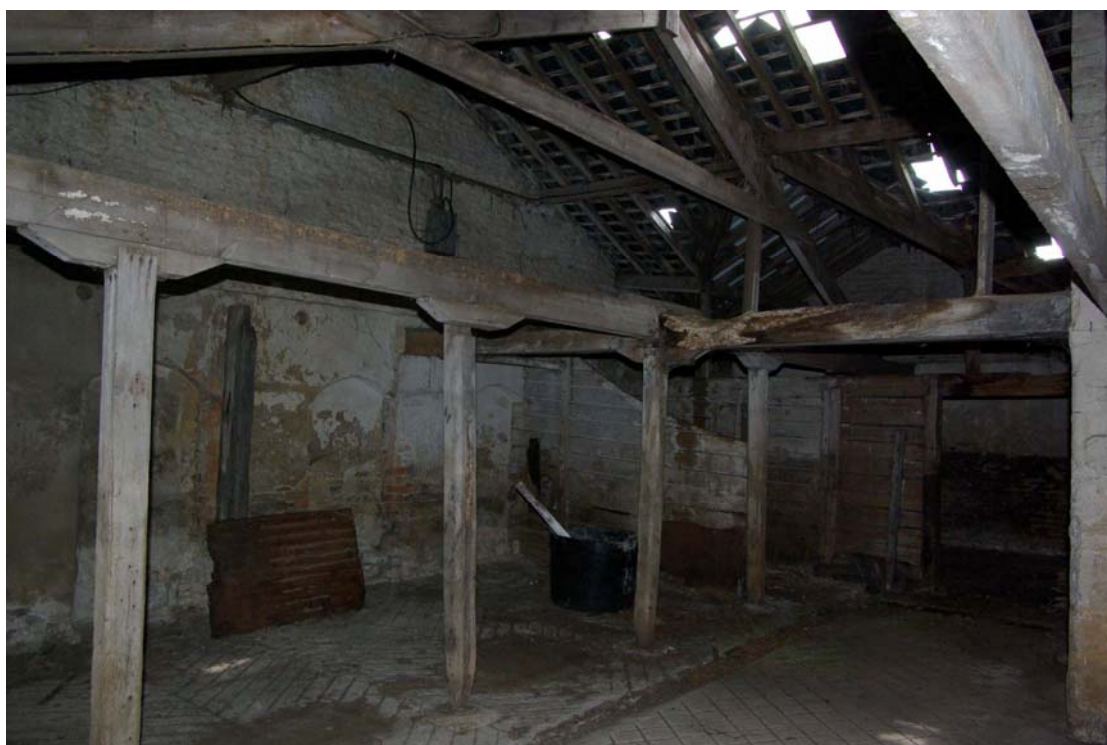
Figure 34 Room 7, east end Looking south east
