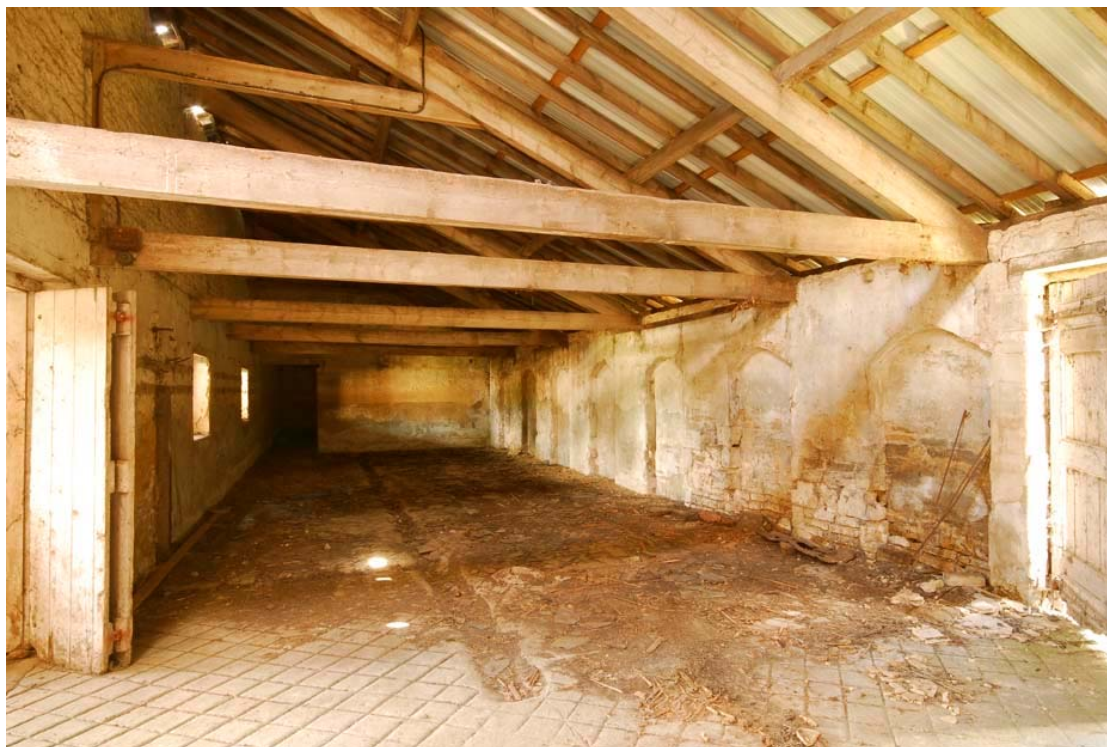
Figure 33 Room 7, west end Looking west
