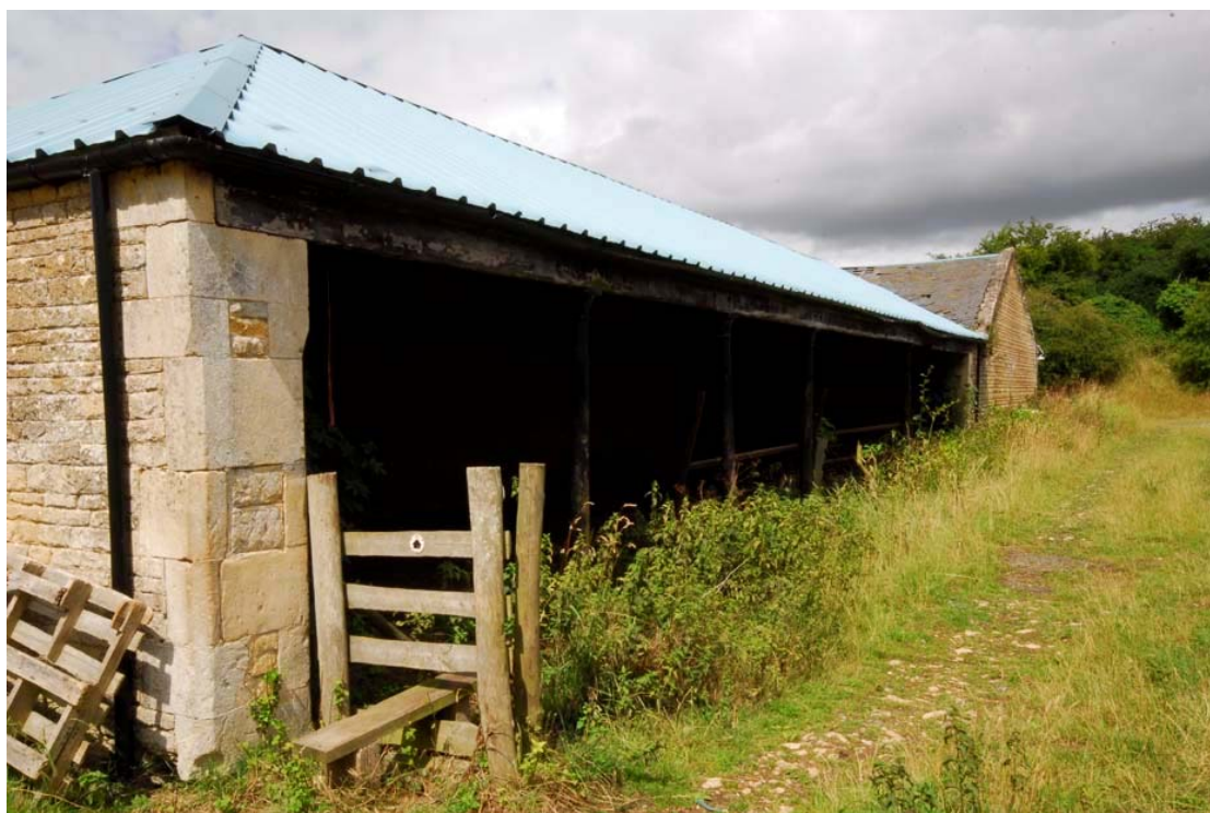
Figure 12 east elevation and track way Looking north west
