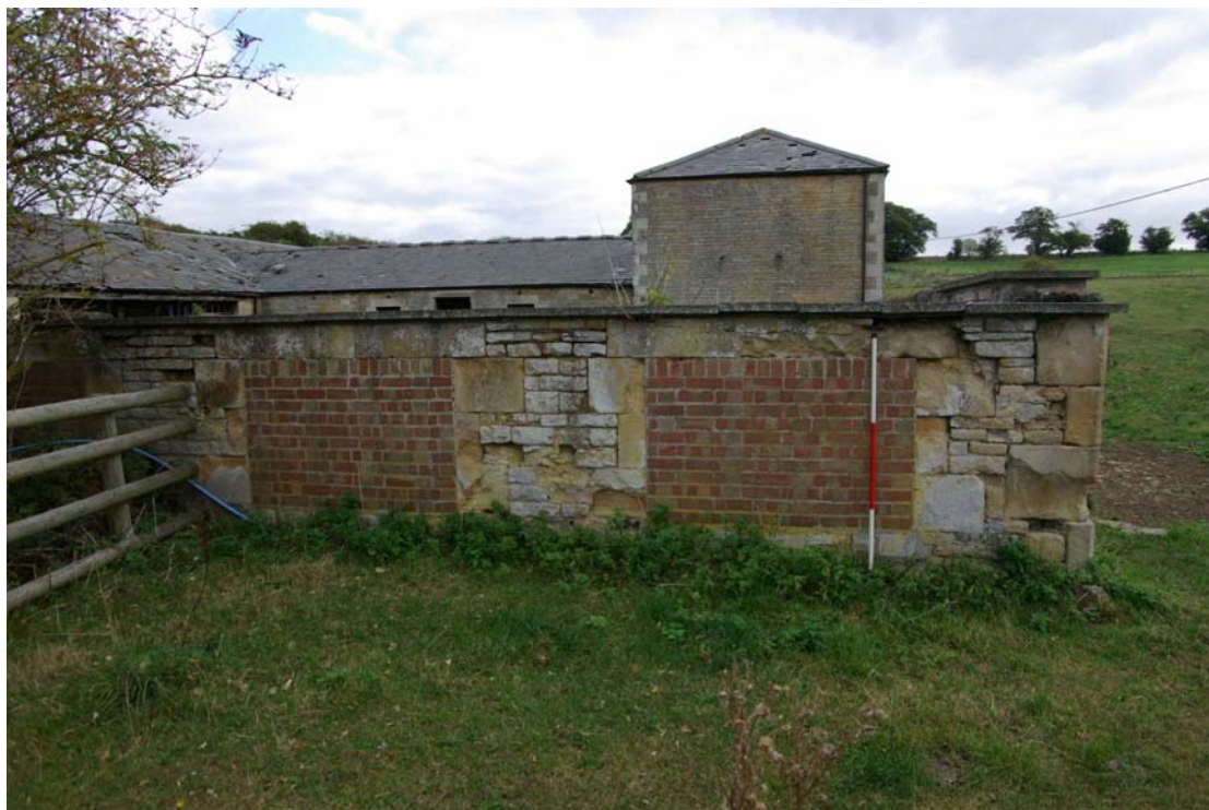
Figure 17 Western courtyard wall and blocked openings Looking east. 1.5m scale
