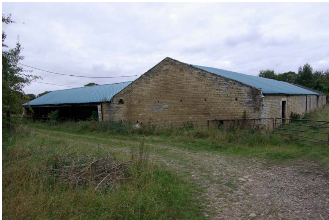
Figure 13 East elevation of north range Looking south west
