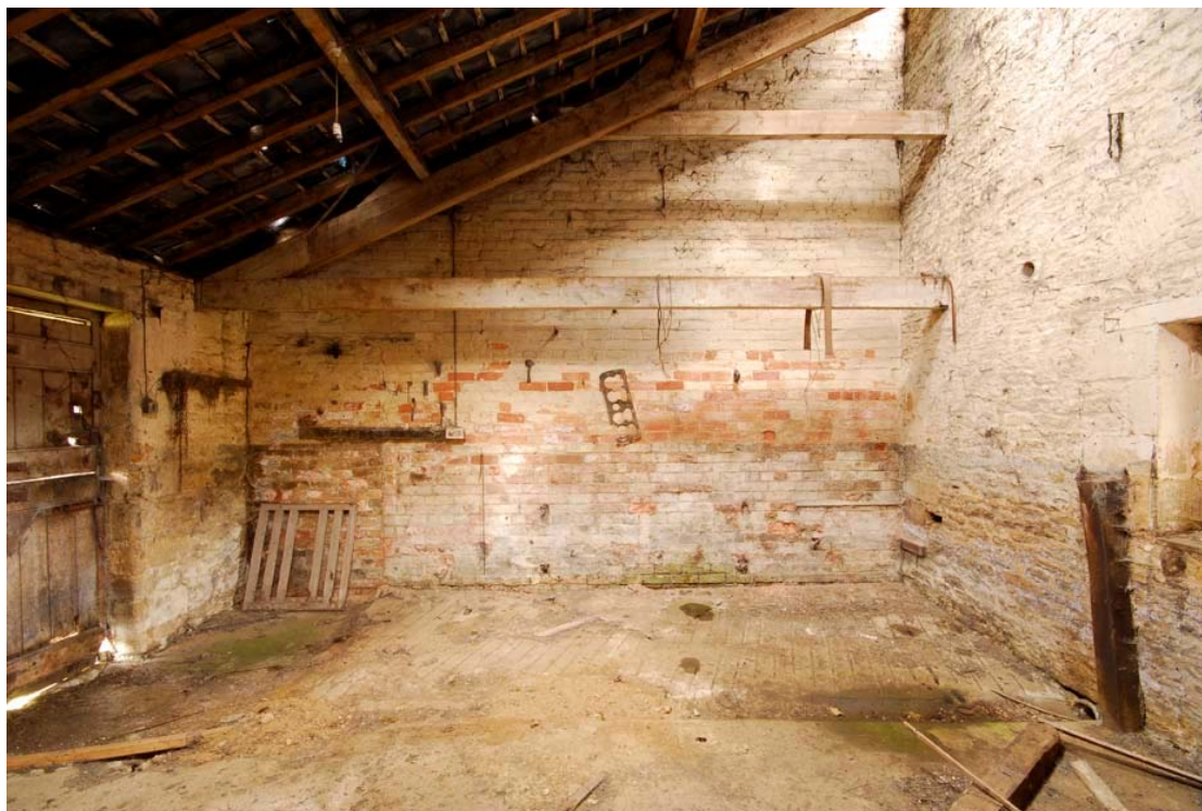
Figure 28 Room 3 with blocked door Facing east
