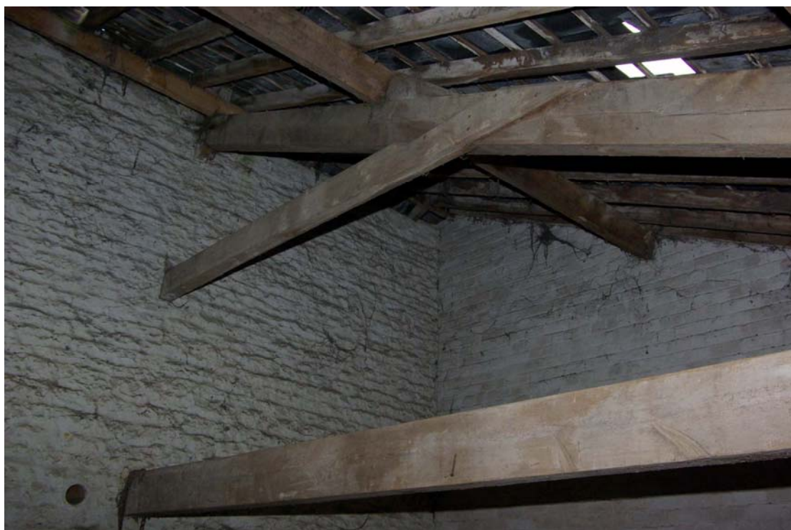
Figure 25 Roof detail of northern half of north range
