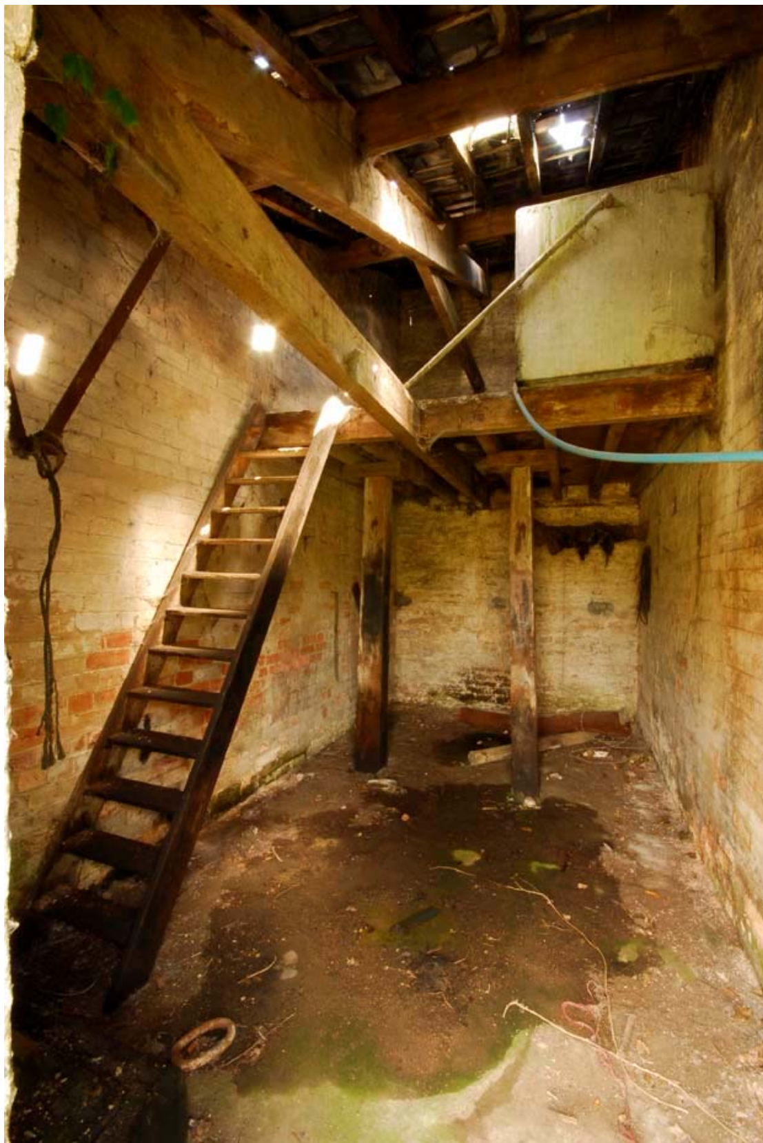
Figure 27 Room 2 mezzanine Looking north
