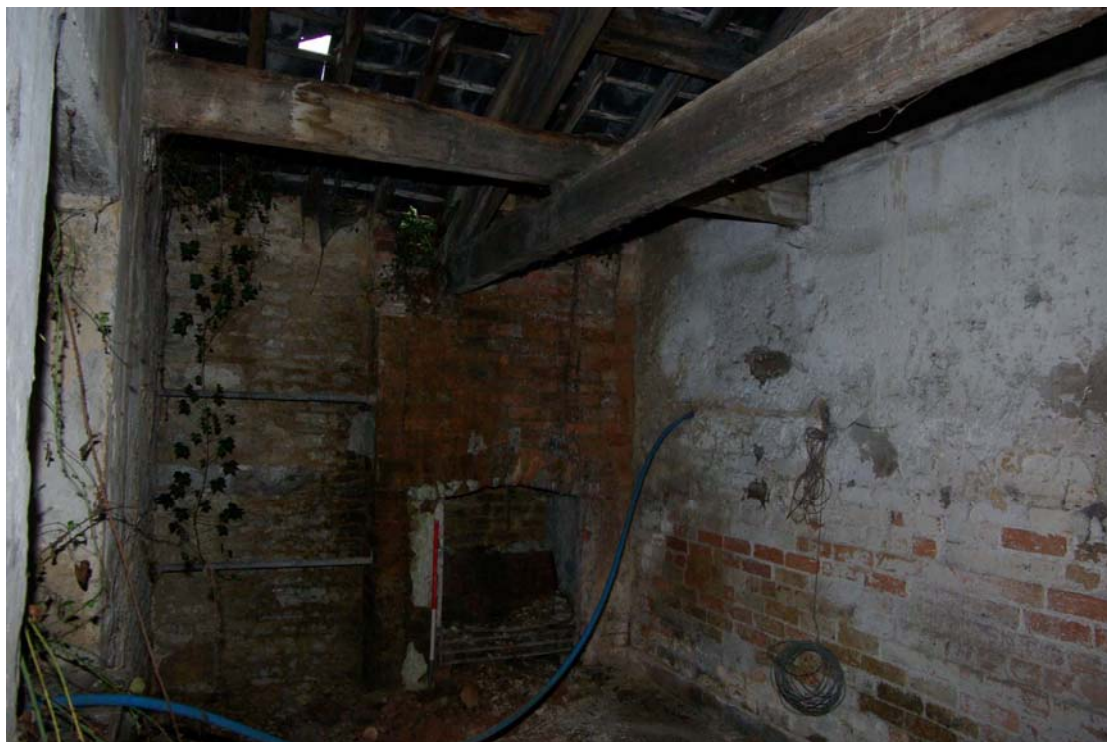
Figure 24 Room 1 fireplace Looking north. 1m scale
