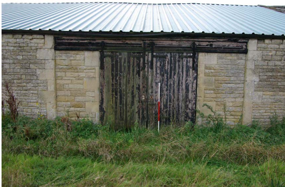
Figure 15 Central sliding doors, north elevation Looking south. 1.5m scale
