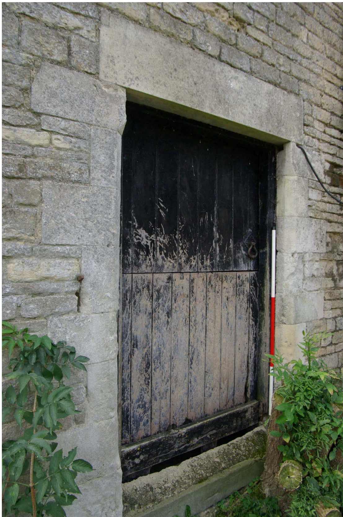
Figure 21 Central building north door detail Looking south west. 1.5m scale
