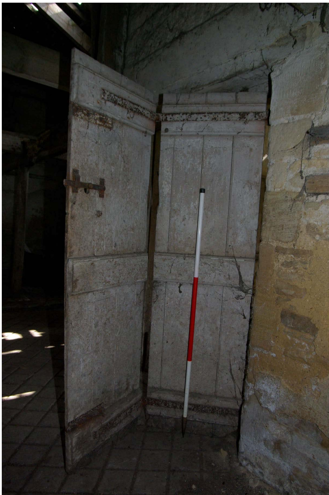
Figure 37 Door from room 7 to 9, detail Looking east. 1.5m scale
