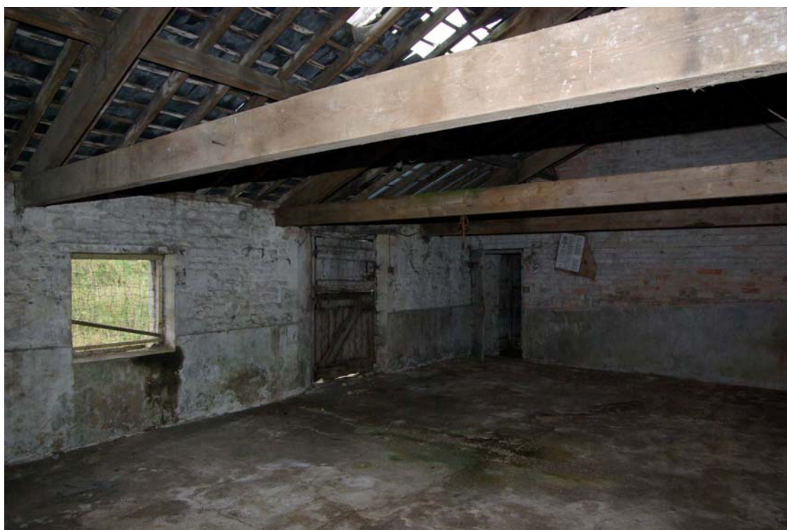
Figure 29 Room 4 Looking north east
