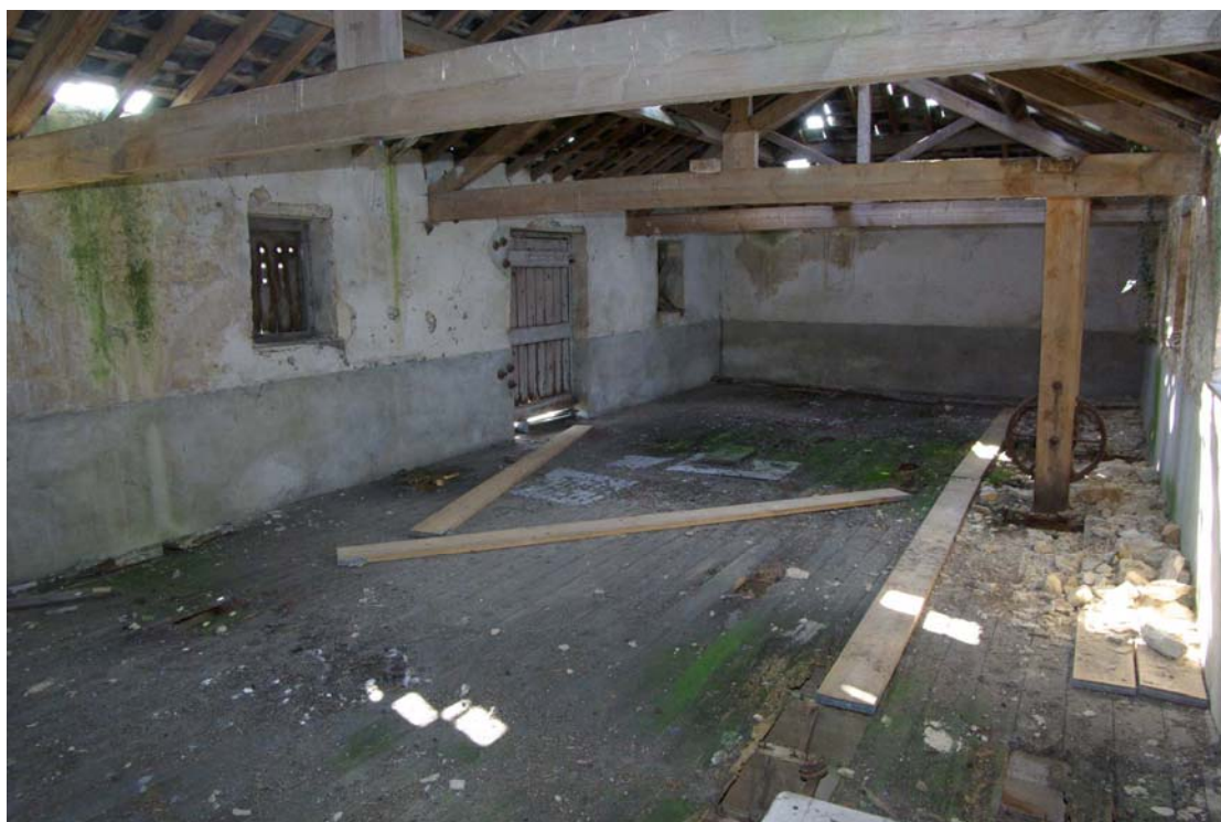
Figure 40 Room 13 central building, first floor Looking south west
