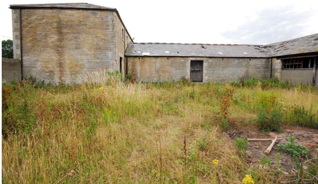
Figure 19 Courtyard 1 east elevation Looking west
