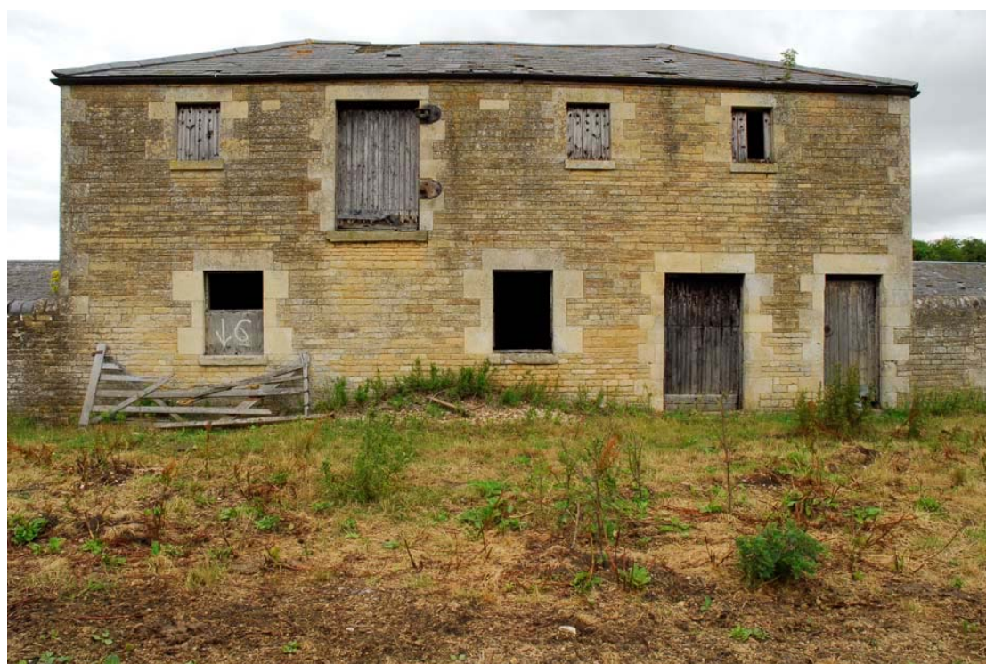
Figure 10 south elevation of central building Looking north
