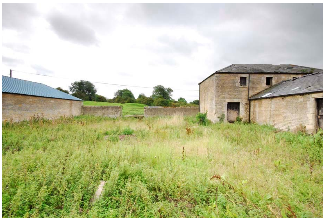
Figure 20 Courtyard 1 north elevation Looking south
