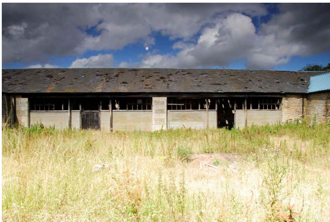
Figure 18 Courtyard 1 south elevation Looking north
