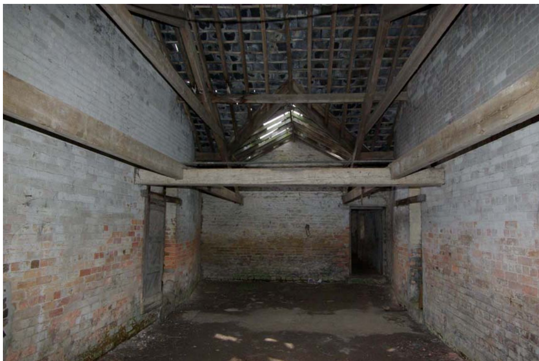
Figure 32 Room 5 south end Looking south
