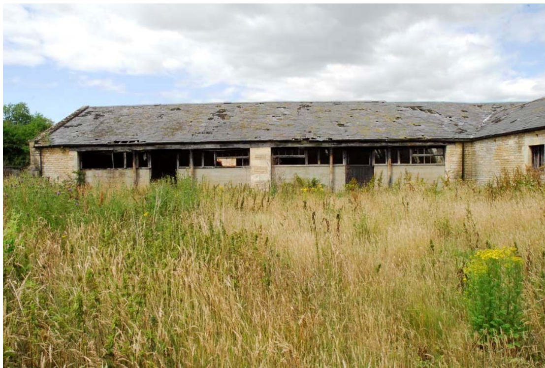
Figure 22 Courtyard 2 south elevation Looking north
