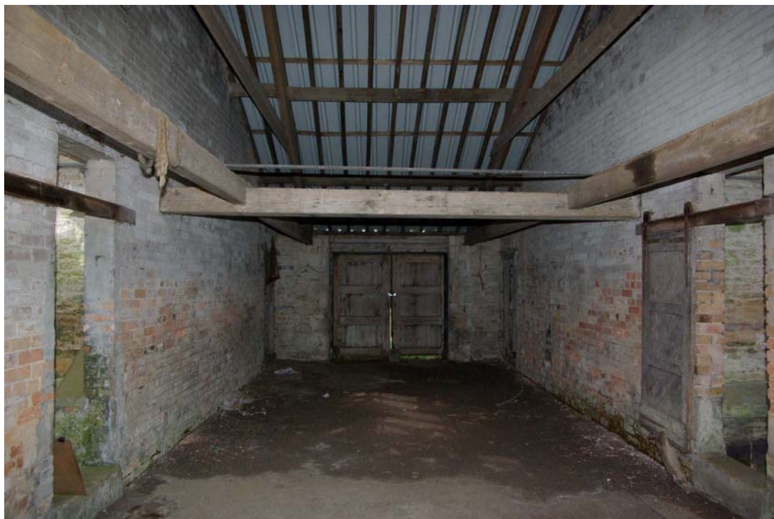
Figure 31 Room 5 door and roof detail, north end Looking north
