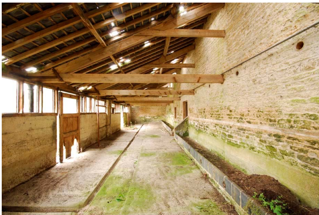
Figure 35 Room 8 Looking west
