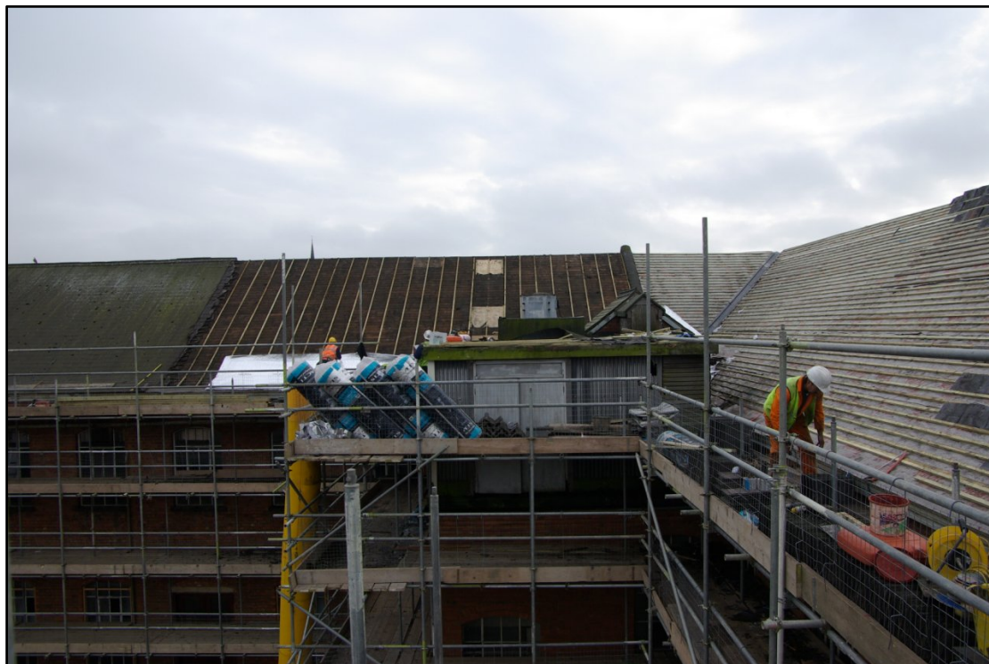
Figure 6 Baine's Lane and Lower Bond Street roof junction. Looking south.
