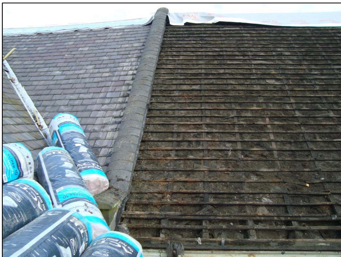
Figure 7 Junction of Baine's Lane and 1870s range Facing north.
