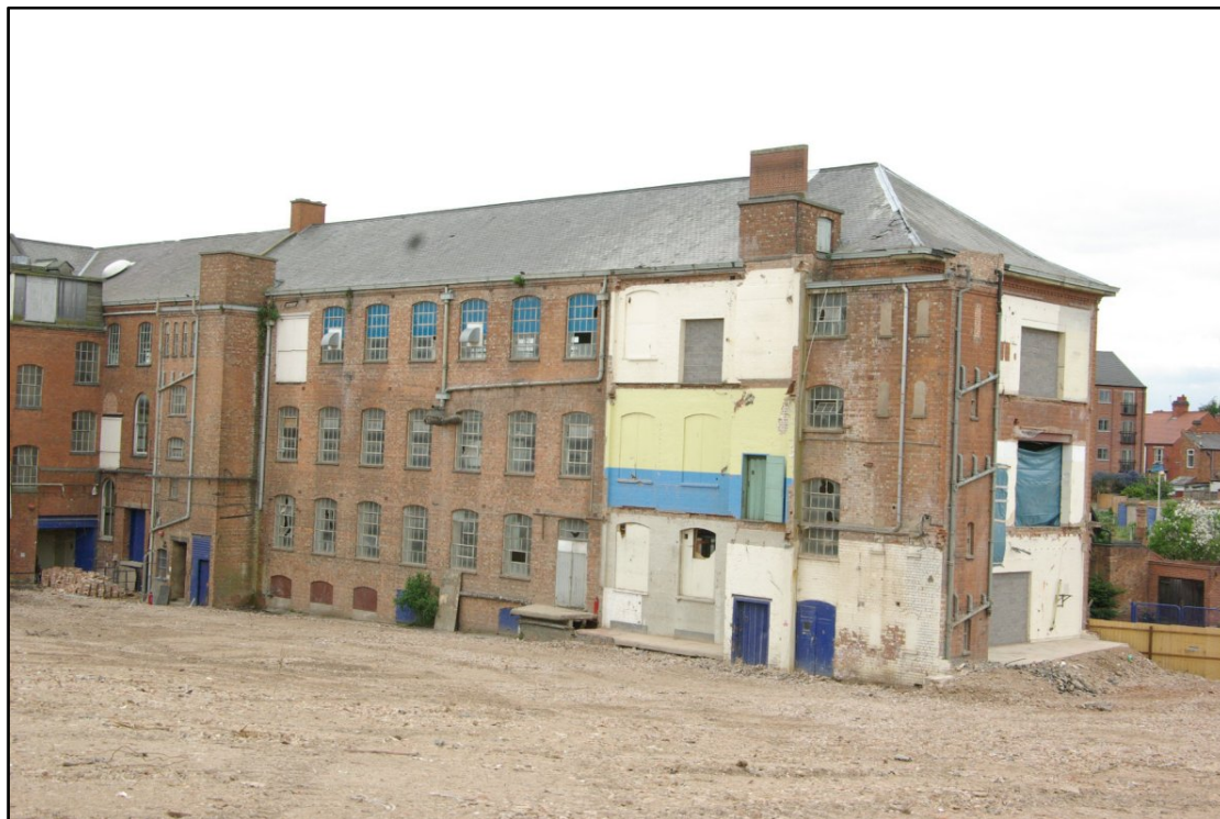
Figure 3. Rear of Lower Bond Street range showing poor state of roof prior to repairs. Looking south west.
