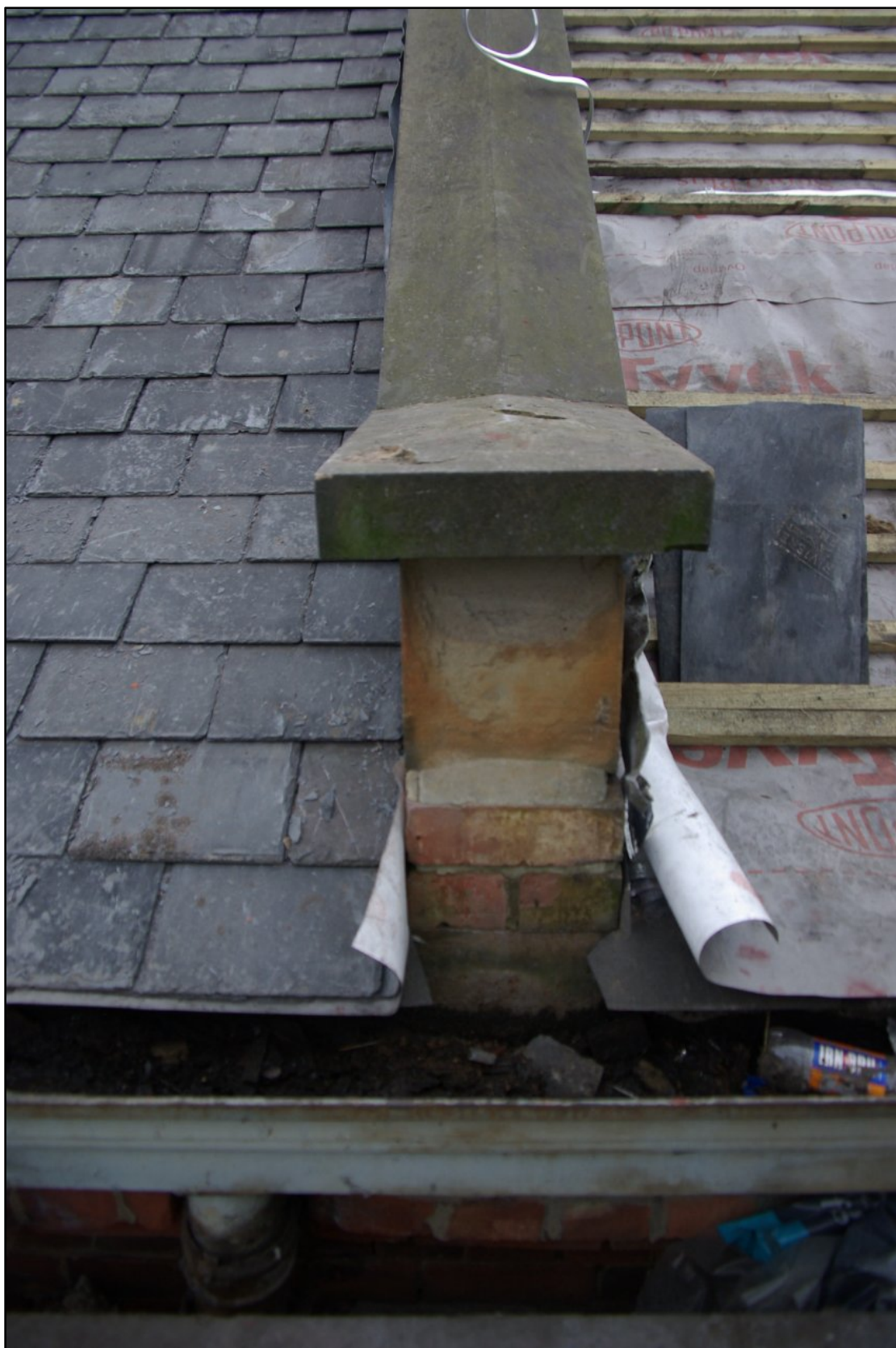
Figure 8 Parapet at junction of 1870s and 1910 ranges Looking west
