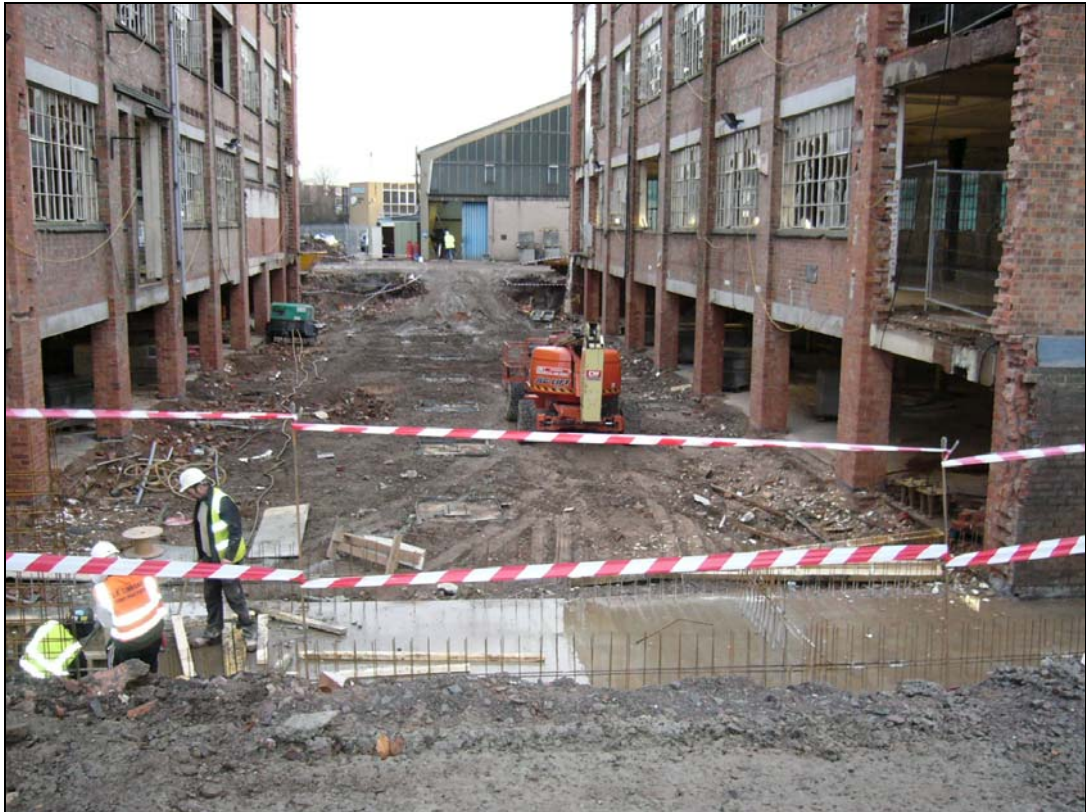
Plate 2. Stripped car park area, looking north.
