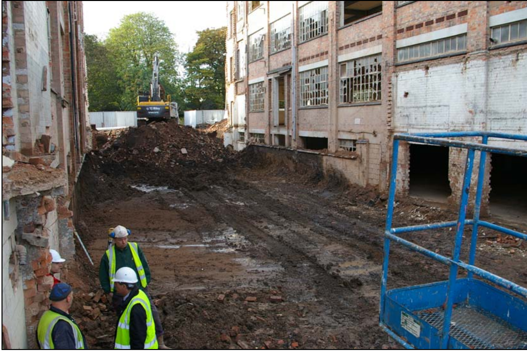
Plate 1. Stripped car park area between wings looking south.
