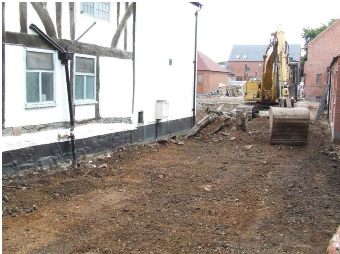
Figure 6 Removal of Driveway Looking East
