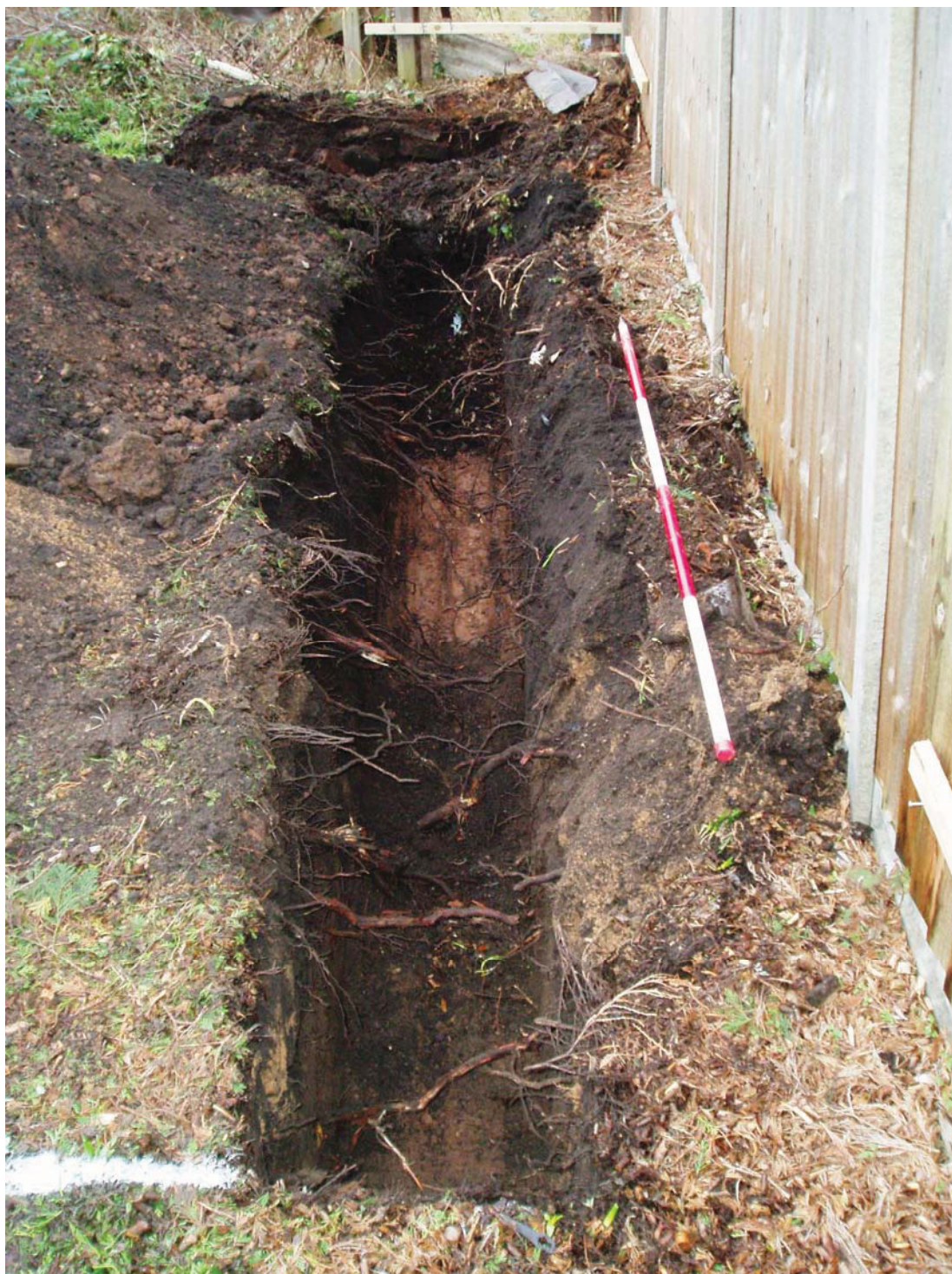
Fig.4 Foundation Trench Looking South
