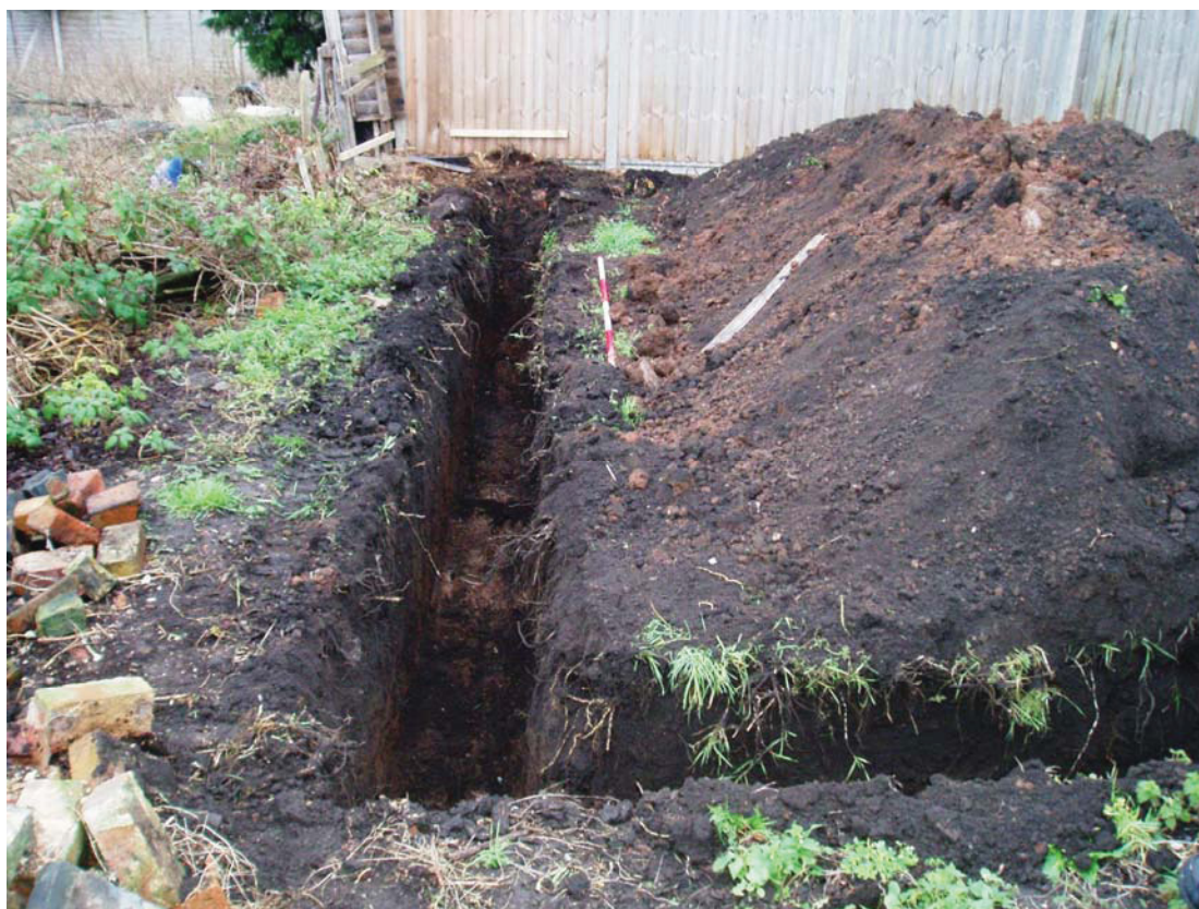
Fig.5 Trenches Looking West
