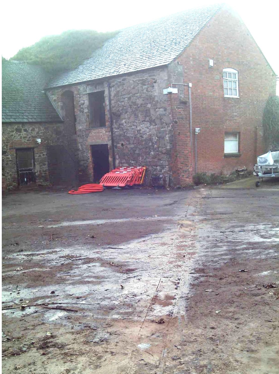
Figure 7 Depot cable trench Asphalt cut ready for excavation. Looking south-east
