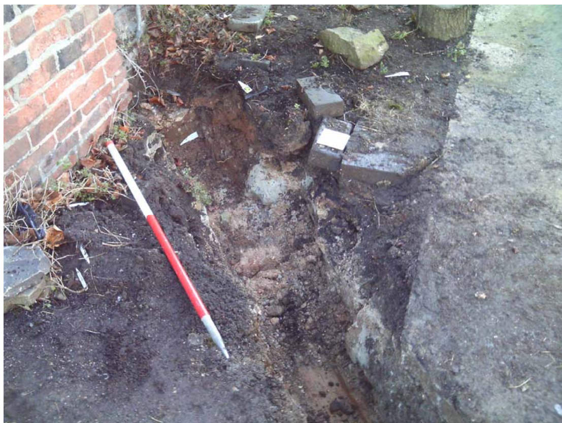
Figure 8 Foundation of stable building Looking south-east
