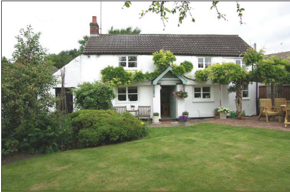
Plate 1: The principal (south) elevation of the cottage. The outhouse is to the left of the picture. The right-hand end of the cottage has already been extended.
