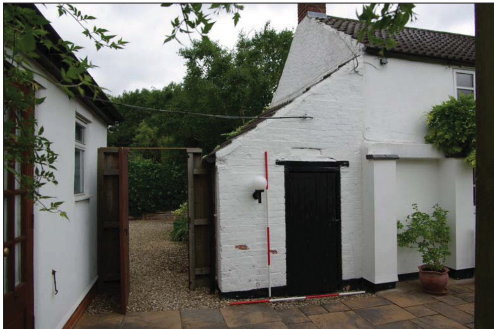
Plate 2: South elevation of the 19th century lean-to that will be demolished.
