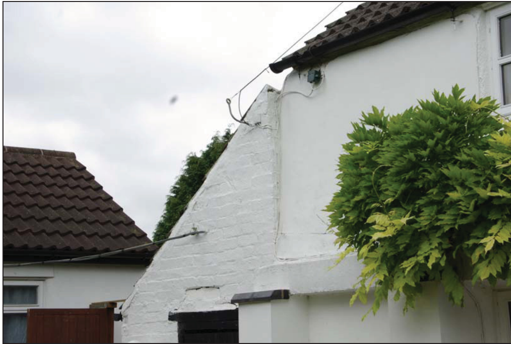
Plate 3: The join between the brick 'lean-to' and cob walls of the original cottage.
