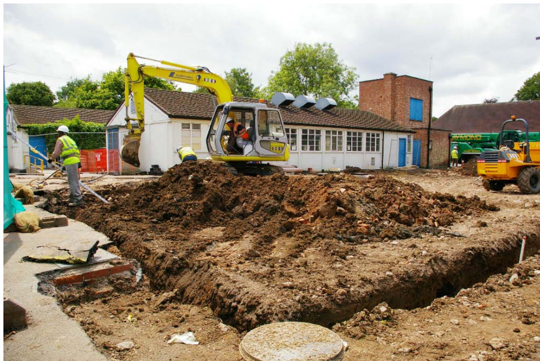
Plate 2 Excavation of trenches on the east side of the development area.
