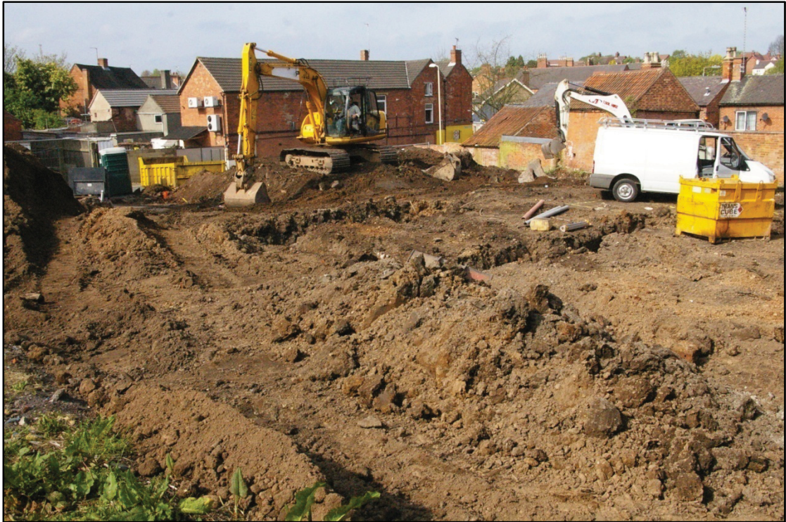
Figure 4: Ground reduction on development area at rear 22-24 Loughborough Road
