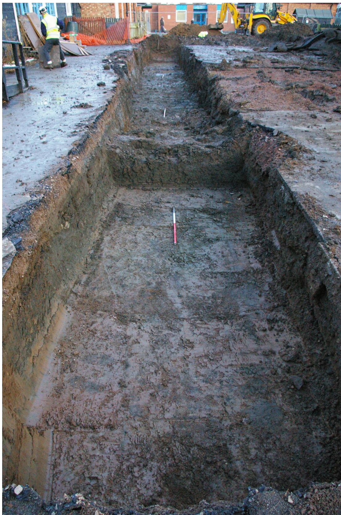
Plate 1 Evaluation Trench 1 looking east
