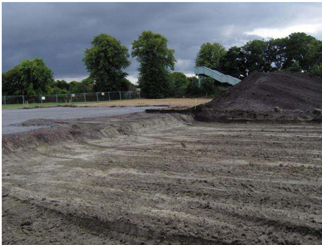
Figure 3: Groundwork excavations area strip
