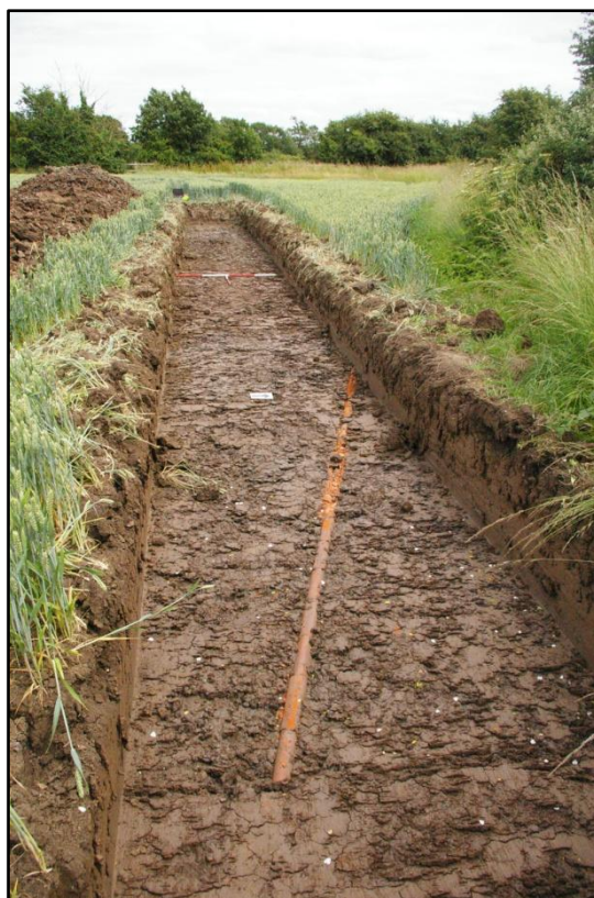
Plate 1 Evaluation Trench 5 looking east ceramic field drain found at base of the trench
