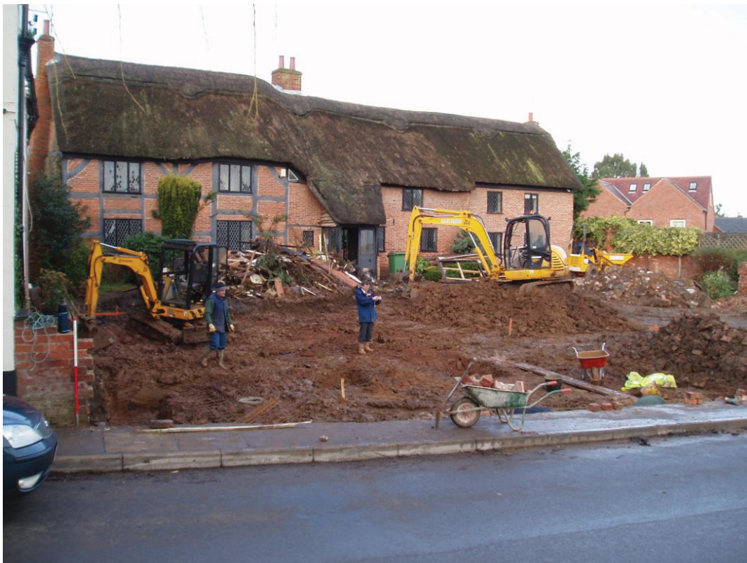
Figure 6 General view of the garage area looking west
