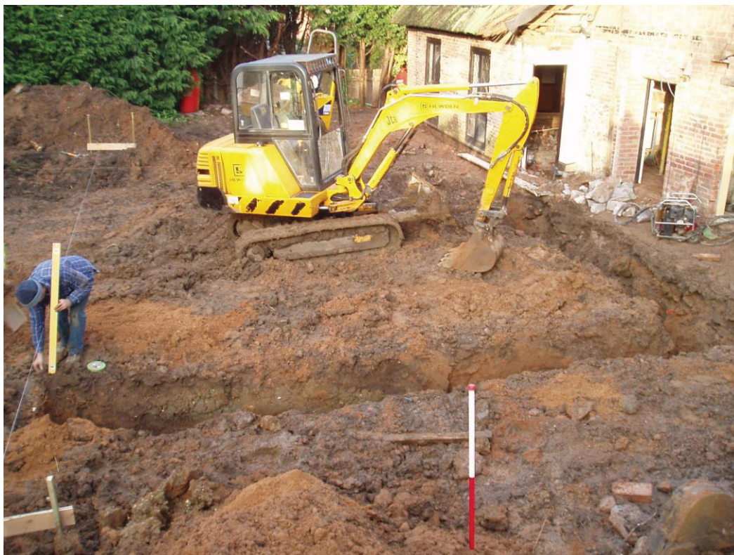
Figure 4 General view of rear looking north
