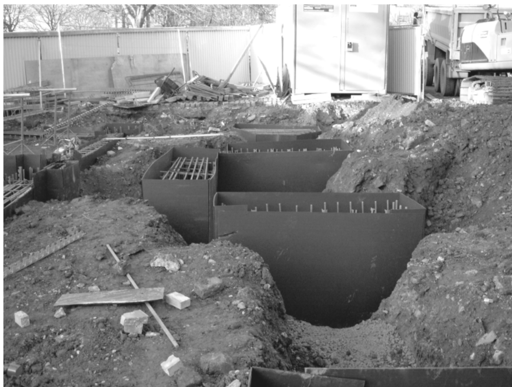
Figure 4 - The lift pit partly constructed, looking north
