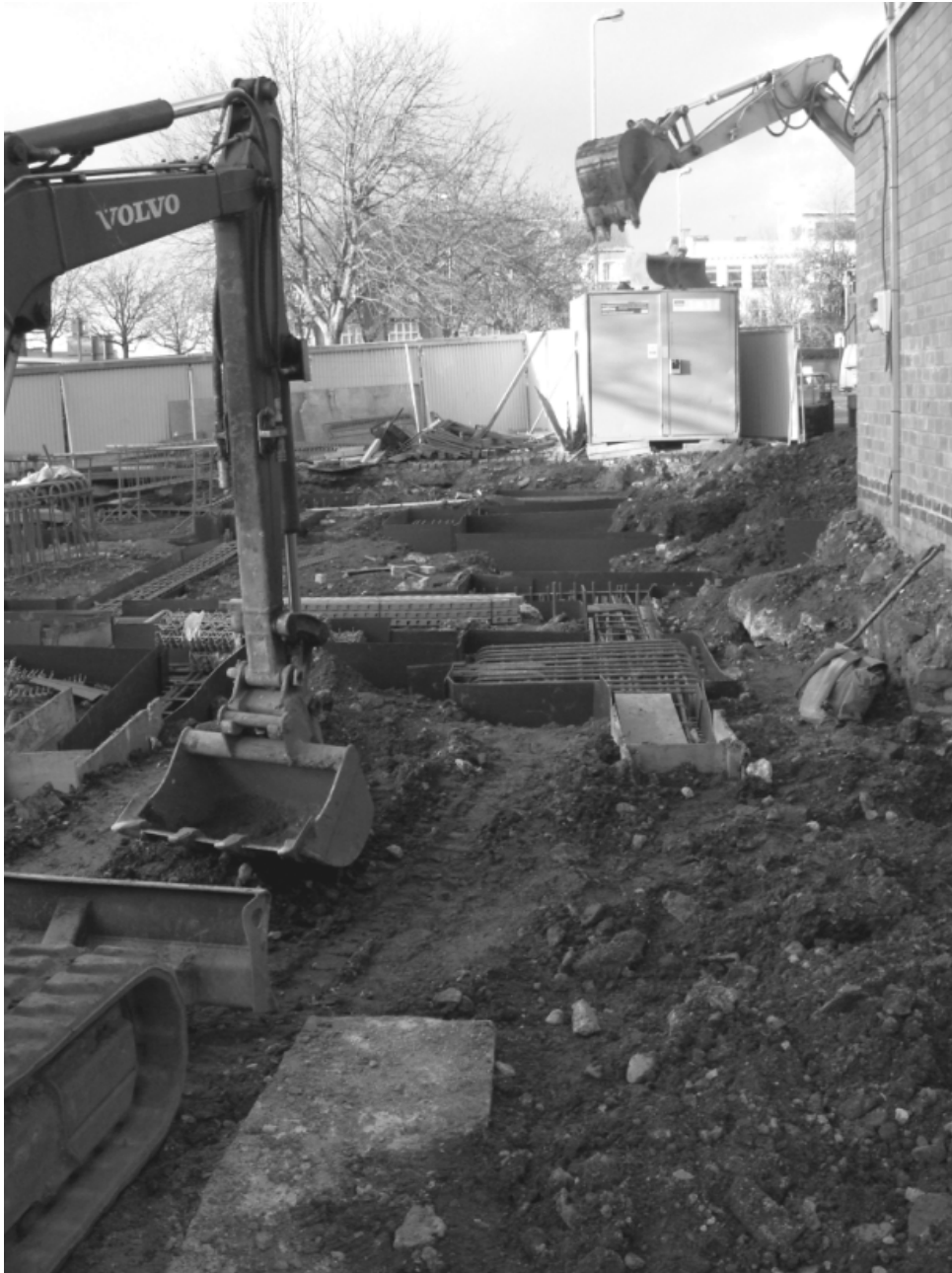
Figure 5 - the foundations in progress showing constrained nature of site. Looking north
