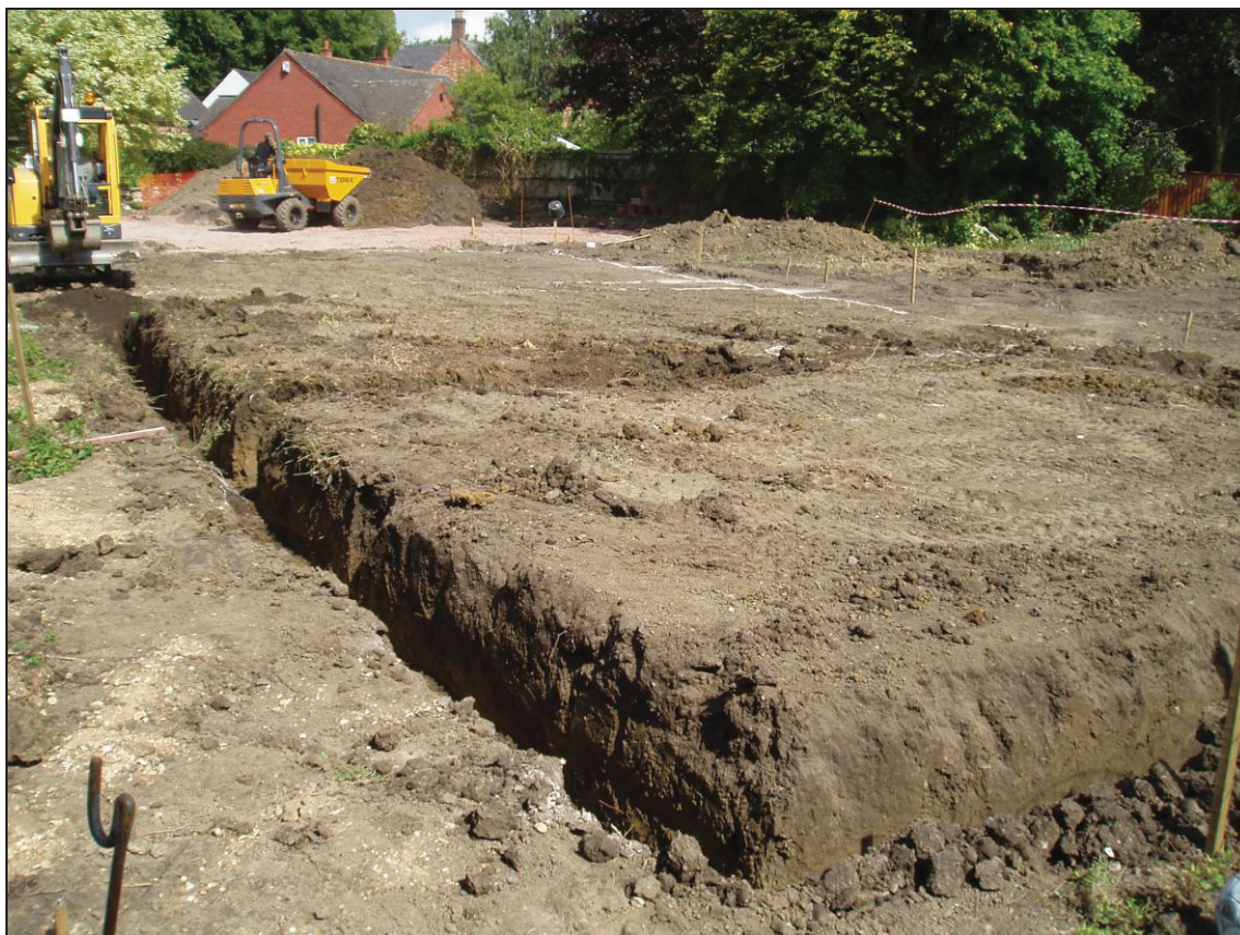
Figure 5 General view looking north-west
