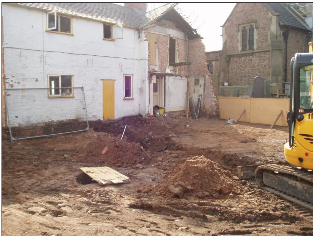
Figure 5 General view looking east
