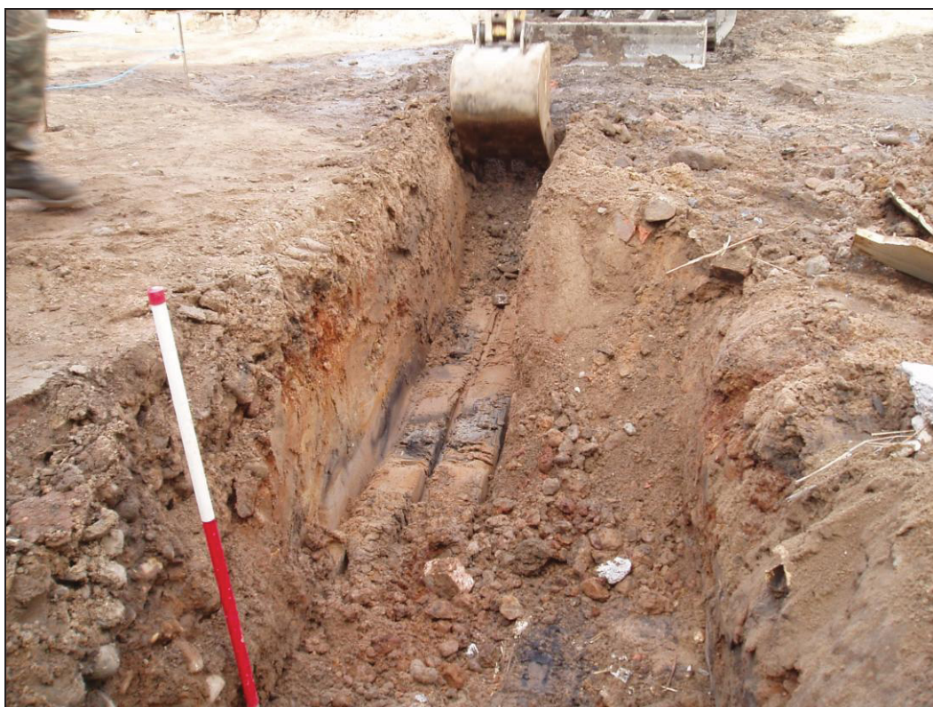
Figure 6 Re-excavated sewer trench looking west
