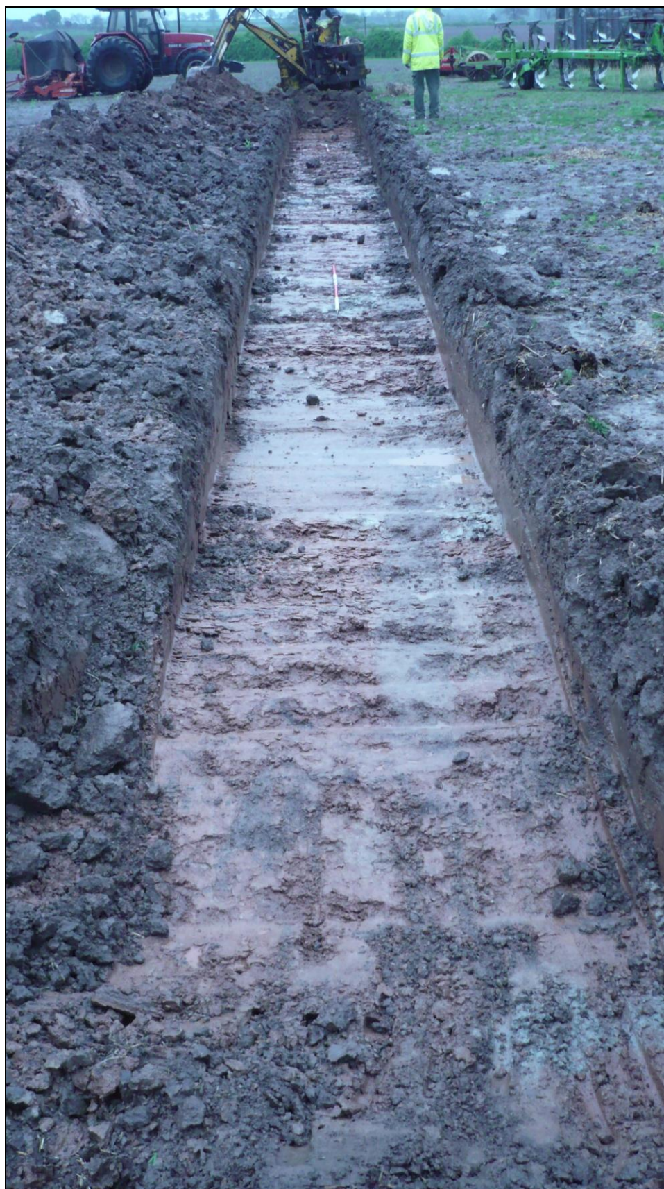
Figure 4 Trench 1 looking north-west
