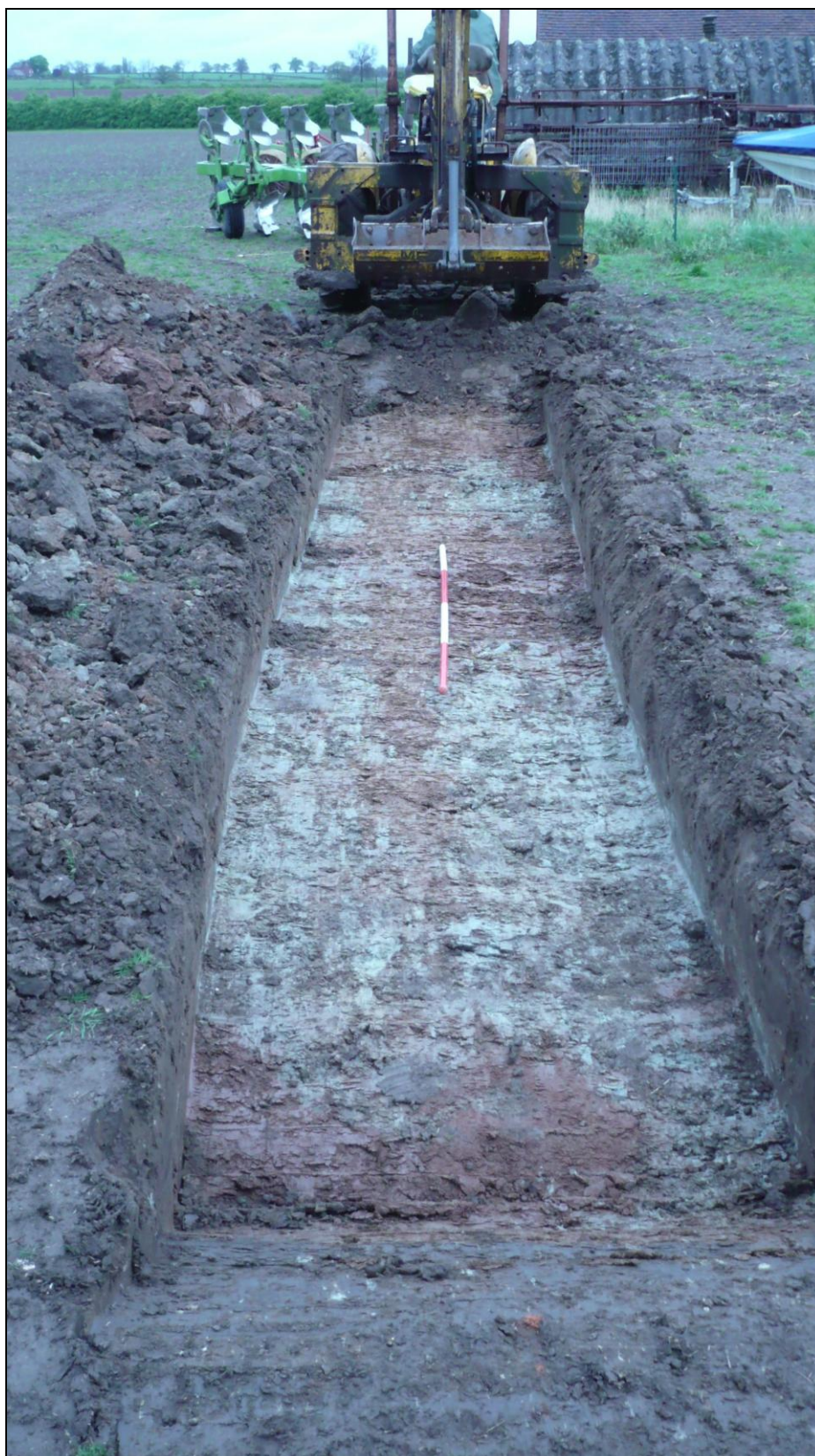
Figure 5 Trench 2 looking north-west
