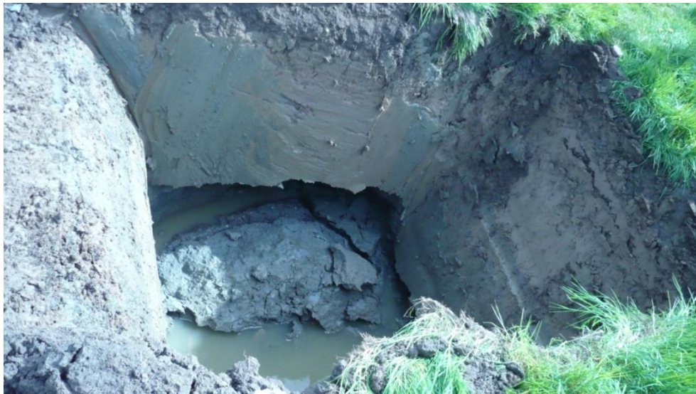
Figure 11: Trench 4 southern end west facing section of soil profile collapse
