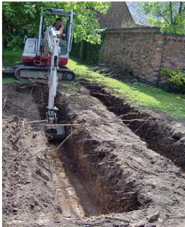
Plate 2 Excavation of foundation trenches in progress
