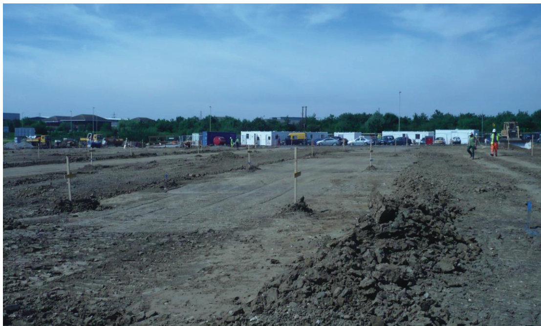
Figure 6: View of site groundworks from the south
