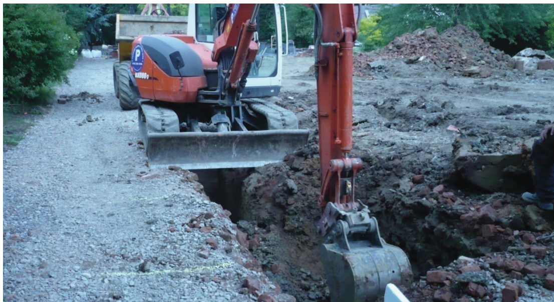
Figure 4: Working shot of west gable wall foundation trench ( view north)
