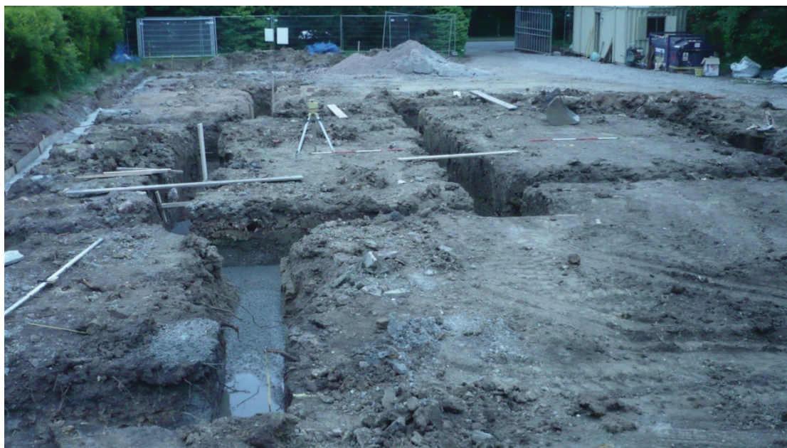
Figure 3: Front of site showing new residence foundation trenches (view south)
