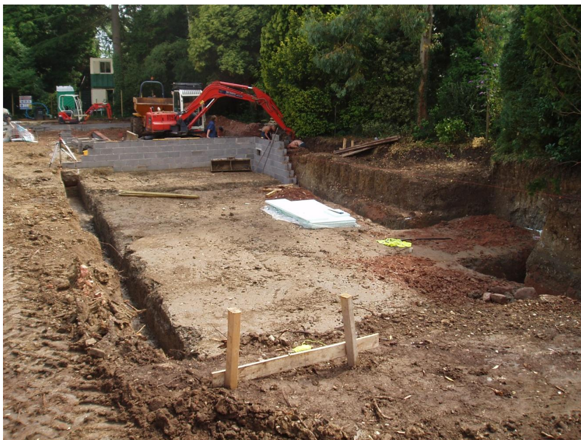
Figure 8 General view looking south
