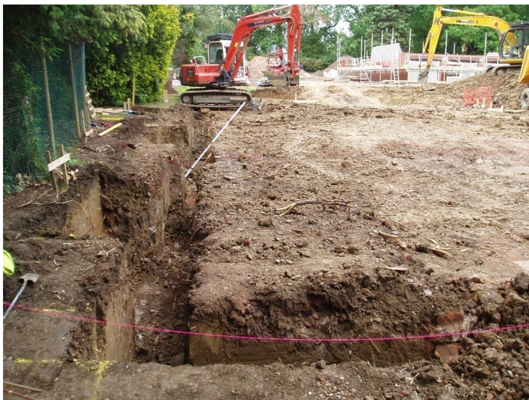
Figure 6 General view looking north
