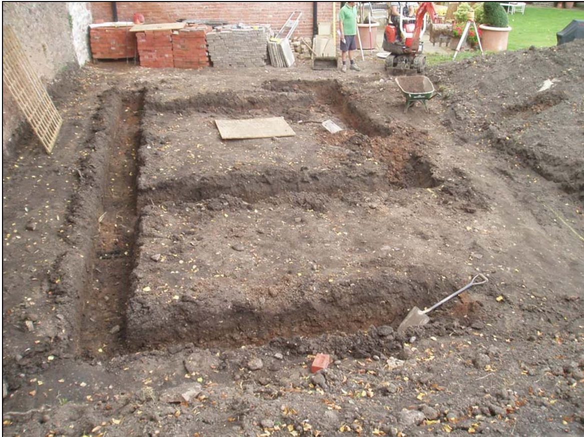
Figure 5 General shot looking west
