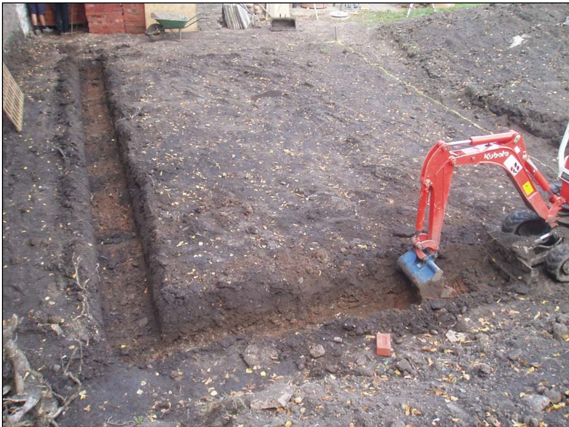
Figure 4 General shot looking west
