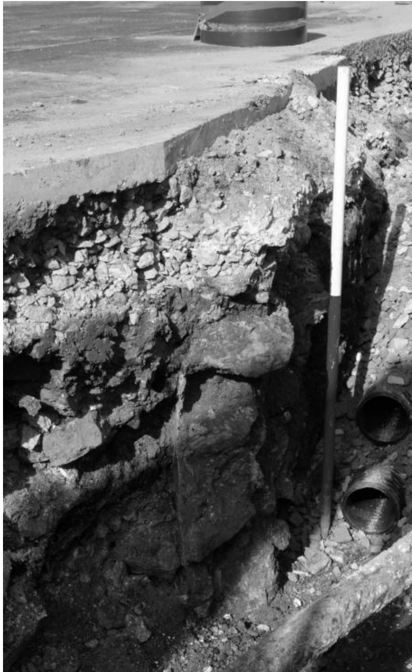
Figure 9 - Stone Built cellar, (Wall 4) with vertical plaster strip visible, looking south-west
