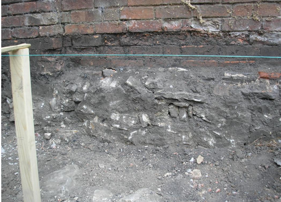
Plate 3: Brick retaining wall overlying earlier stone wall
