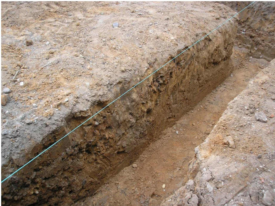
Plate 2: Section of foundation trench showing exposed natural subsoils.
