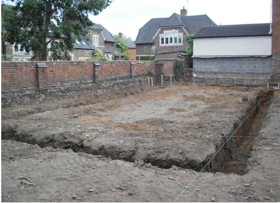
Plate 1: Foundation trenches looking north-east
